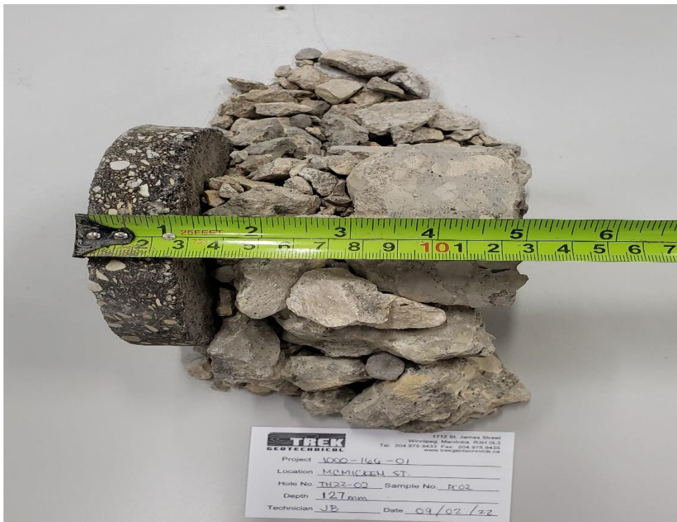
Photo 2: Pavement Core Sample at Test Hole TH22-02
