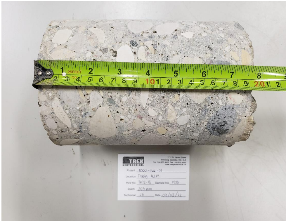
Photo 3: Pavement Core Sample at Test Hole TH22-15
