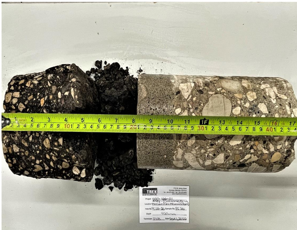
Photo 4: Pavement Core Sample PC-26
