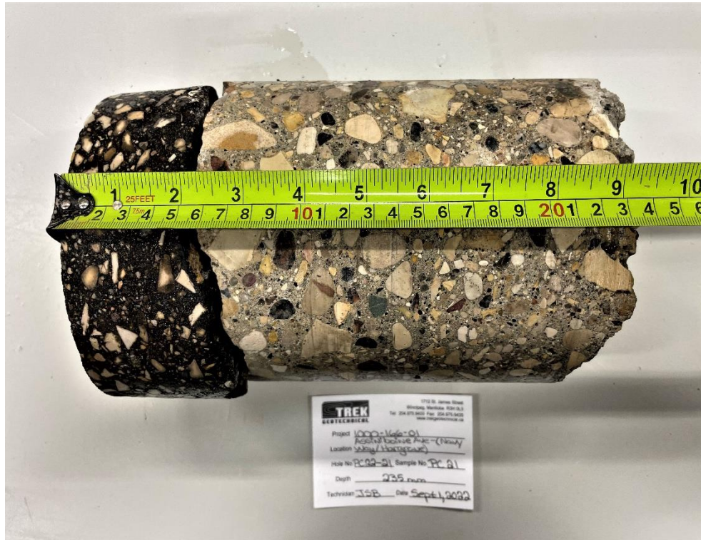
Photo 1: Pavement Core Sample PC-21
