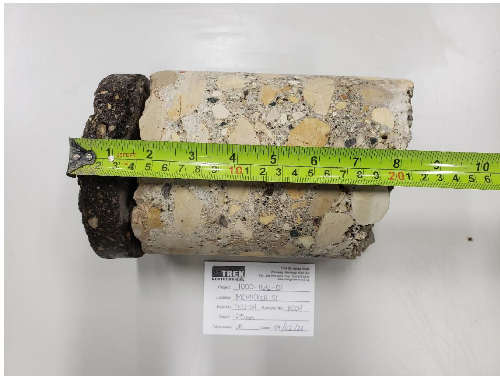
Photo 4: Pavement Core Sample at Test Hole TH22-04
