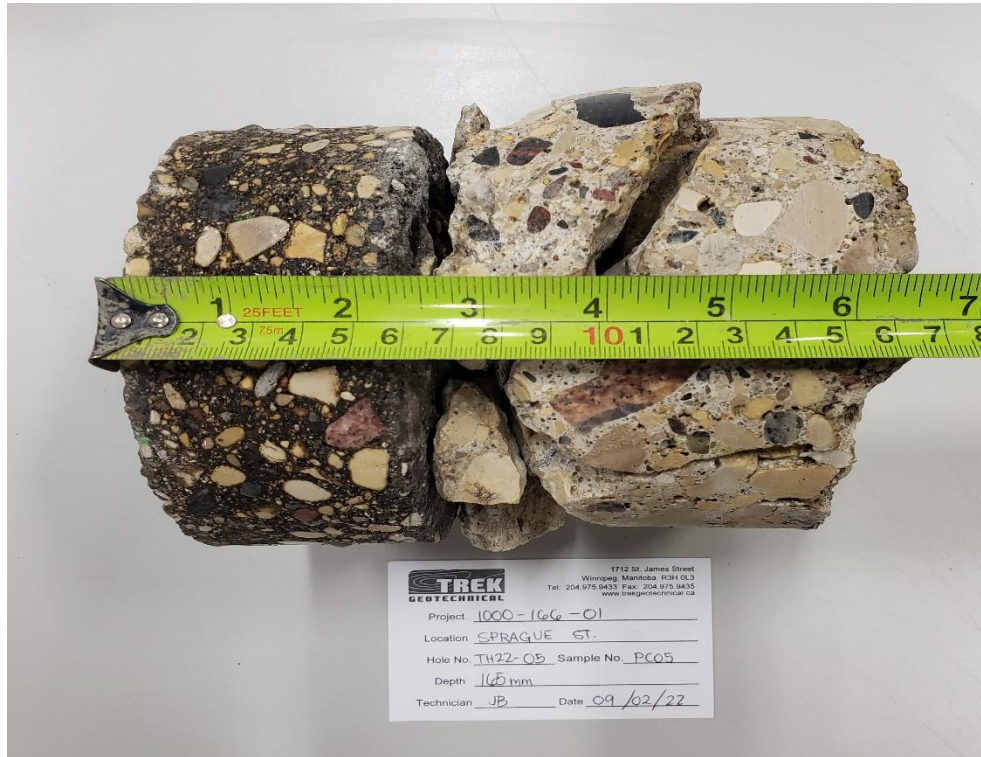
Photo 1: Pavement Core Sample at Test Hole TH22-05
