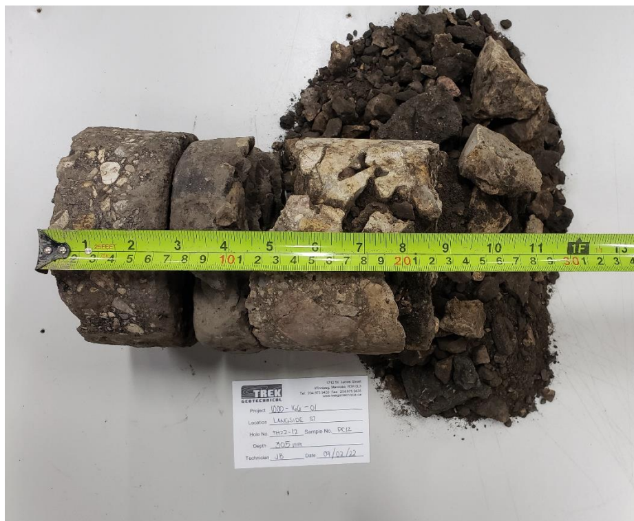
Photo 4: Pavement Core Sample at Test Hole TH22-12
