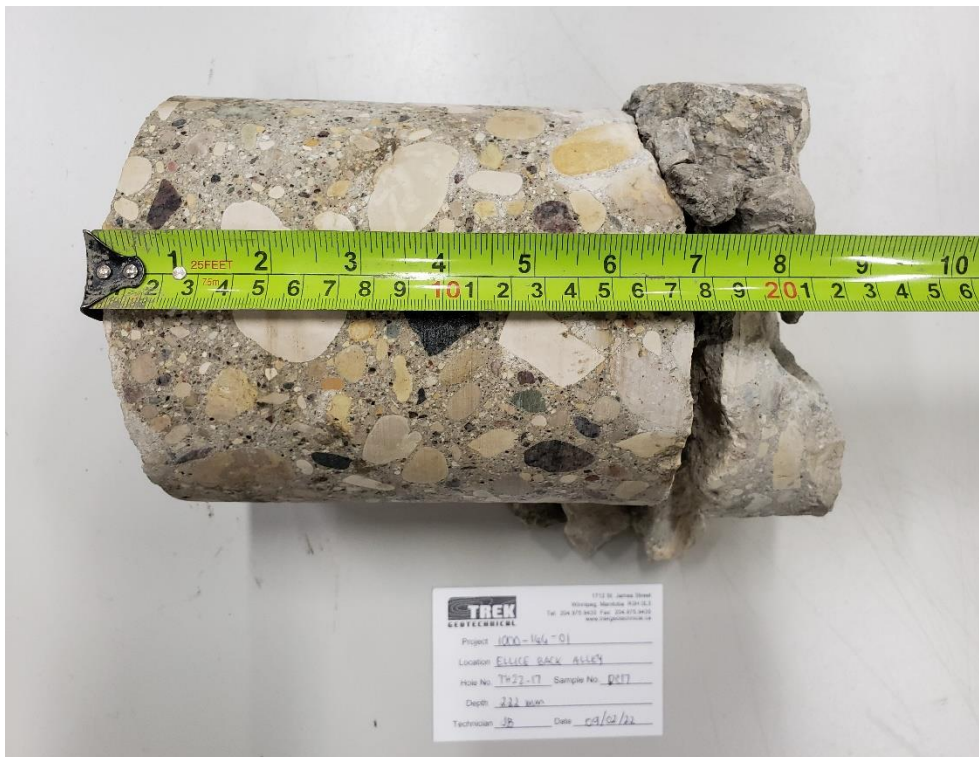
Photo 2: Pavement Core Sample at Test Hole TH22-17
