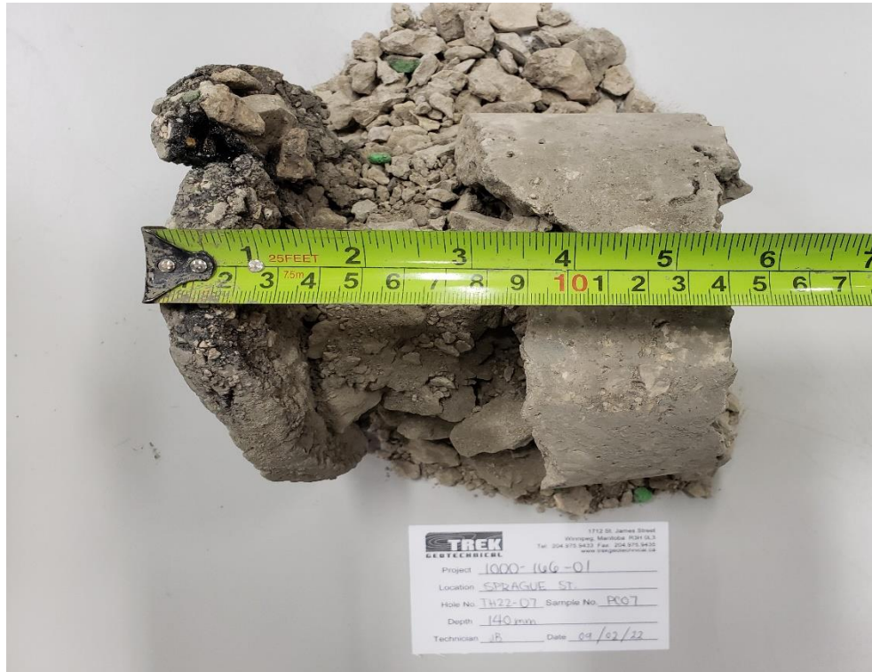
Photo 3: Pavement Core Sample at Test Hole TH22-07
