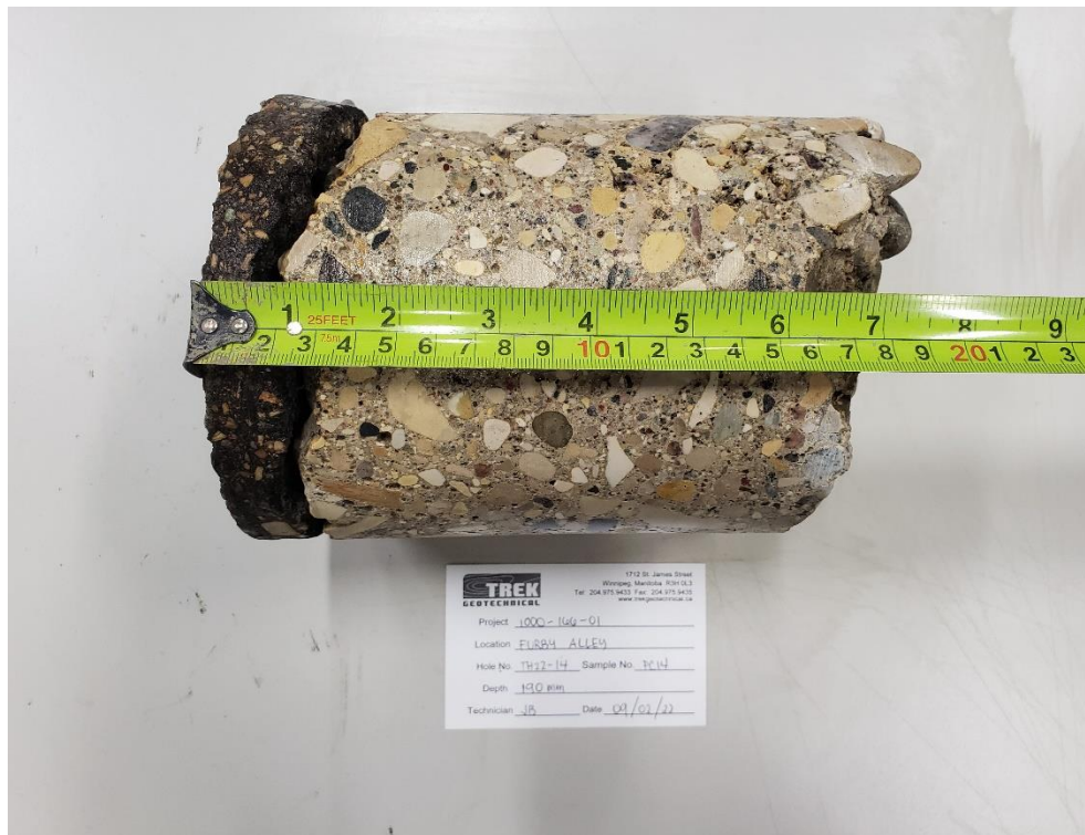
Photo 2: Pavement Core Sample at Test Hole TH22-14
