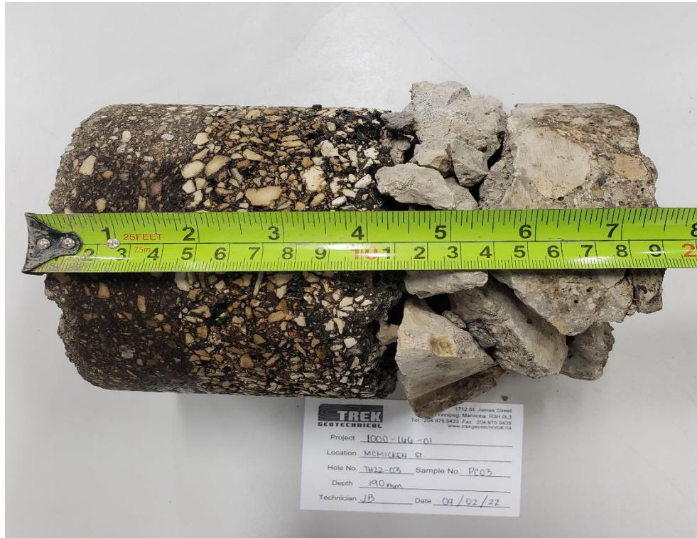
Photo 3: Pavement Core Sample at Test Hole TH22-03
