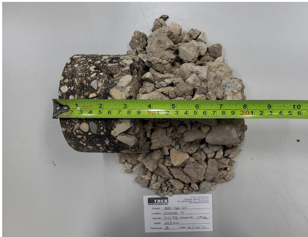
Photo 4: Pavement Core Sample at Test Hole TH22-08
