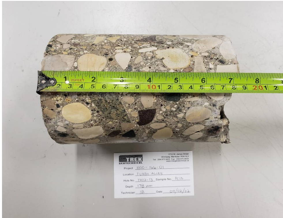
Photo 1: Pavement Core Sample at Test Hole TH22-13
