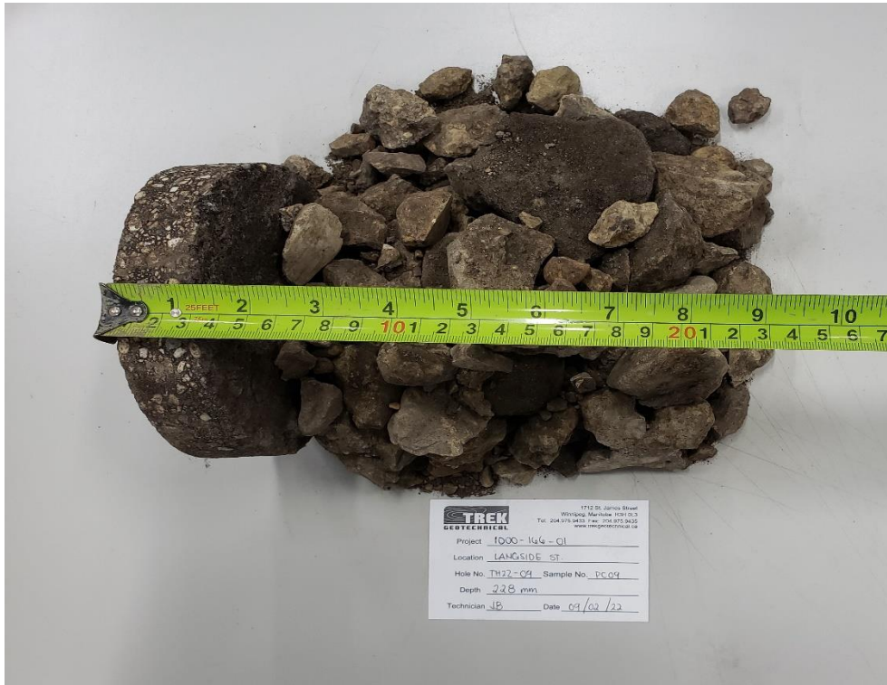
Photo 1: Pavement Core Sample at Test Hole TH22-09
