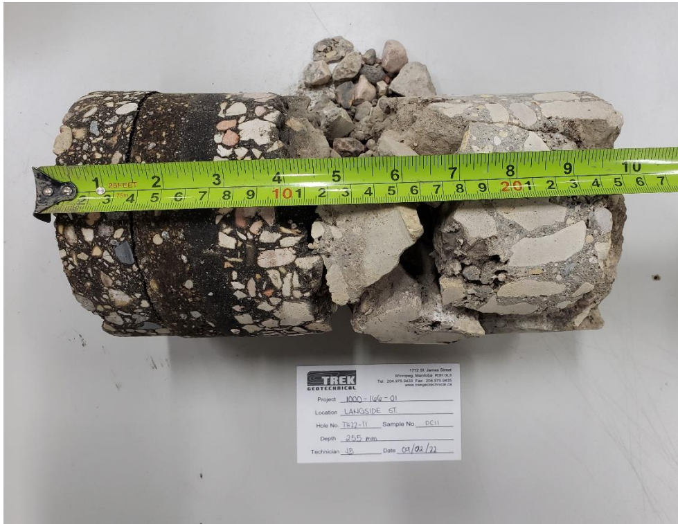
Photo 3: Pavement Core Sample at Test Hole TH22-11
