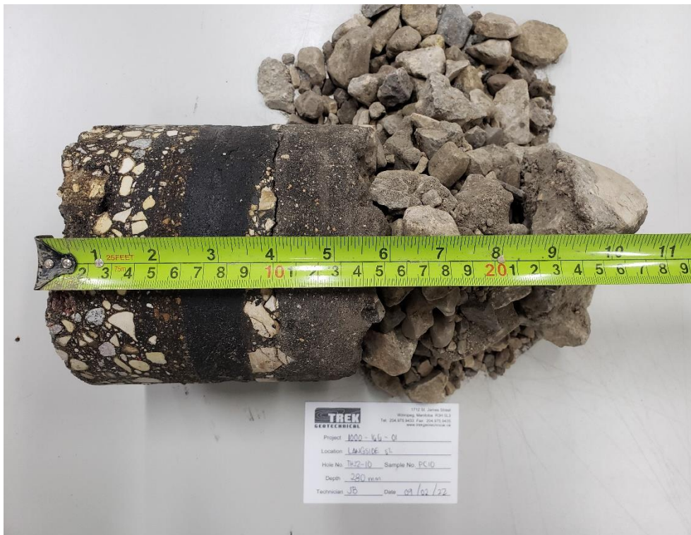
Photo 2: Pavement Core Sample at Test Hole TH22-10
