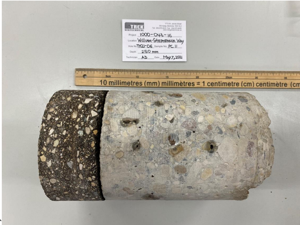
Photo 3: Pavement Core Sample at Test Hole TH21-06
