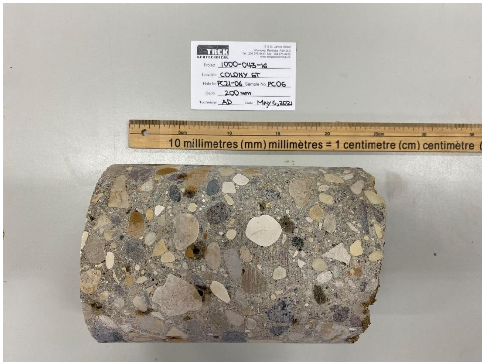
Photo 2: Pavement Core Sample at PC21-06
