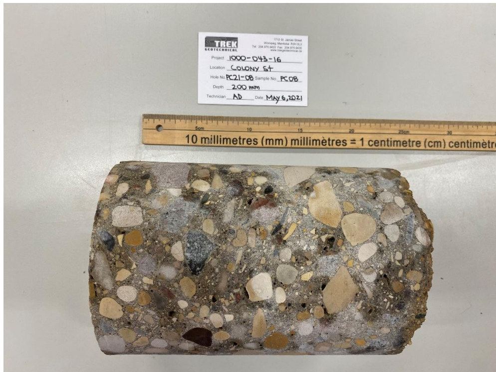
Photo 4: Pavement Core Sample at PC21-08
