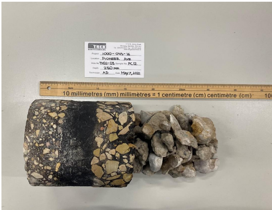
Photo 2: Pavement Core Sample at Test Hole TH21-03
