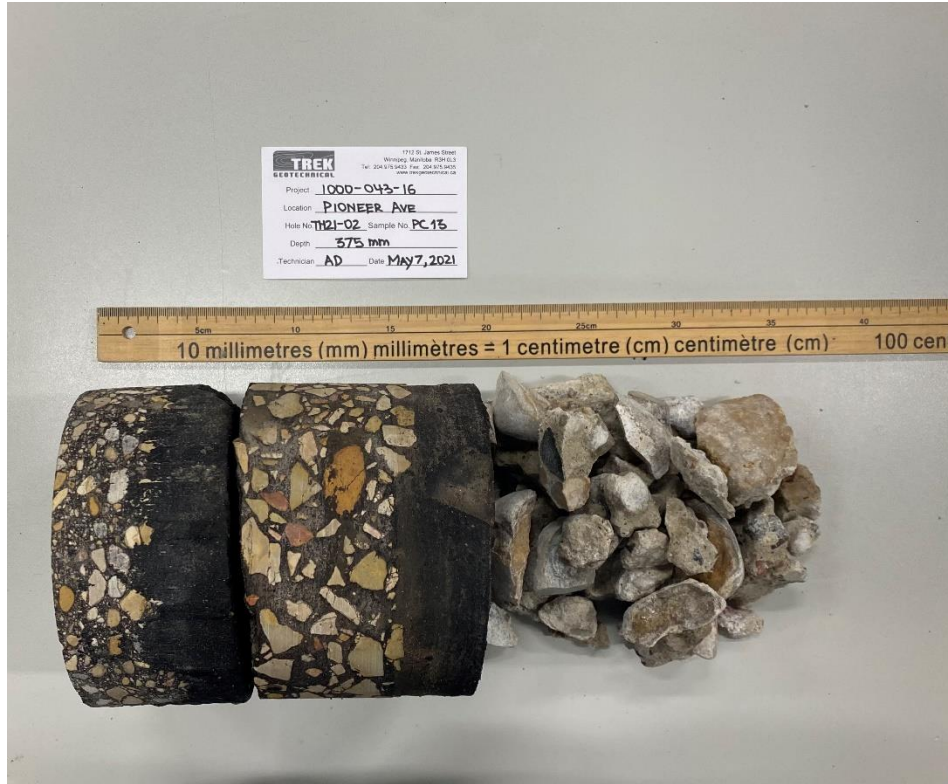
Photo 1: Pavement Core Sample at Test Hole TH21-02
