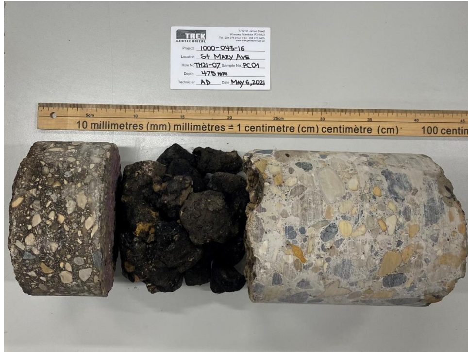
Photo 1: Pavement Core Sample at Test Hole TH21-07
