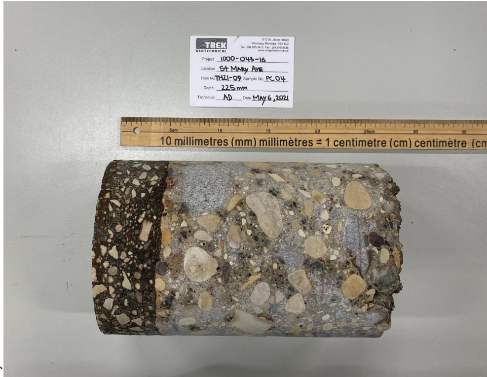
Photo 3: Pavement Core Sample at Test Hole TH21-09
