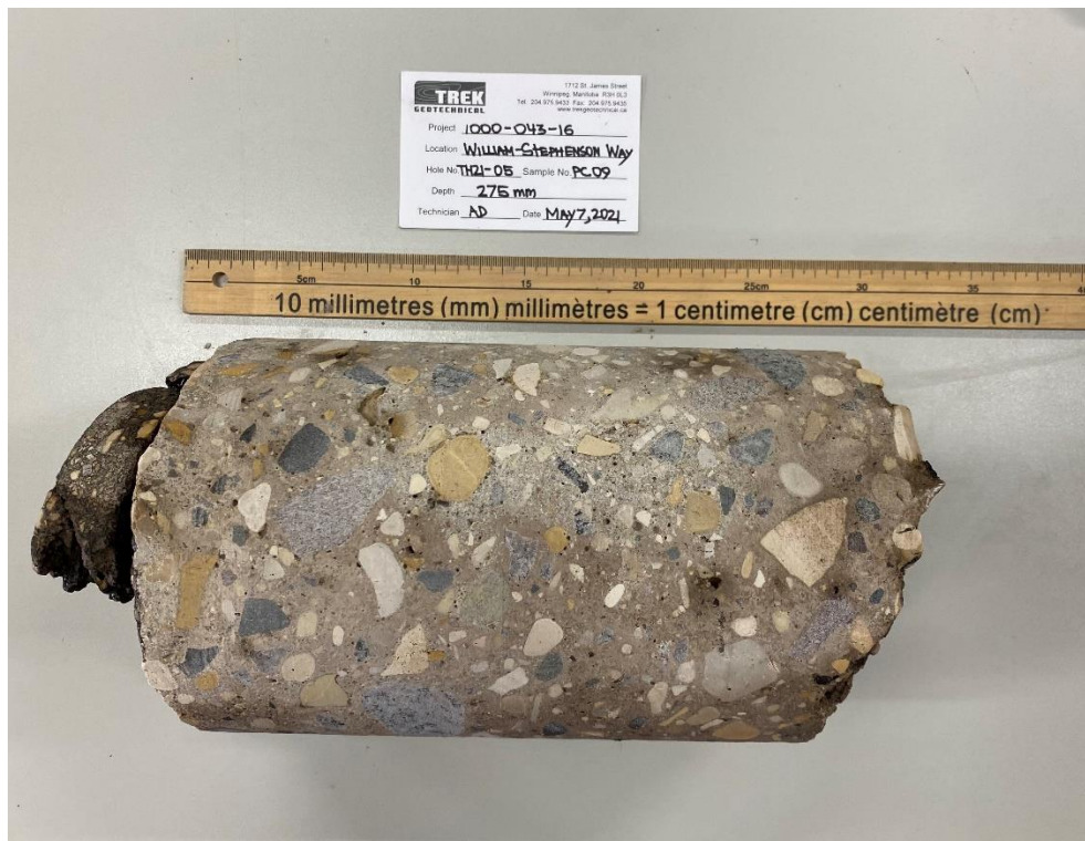
Photo 2: Pavement Core Sample at Test Hole TH21-05
