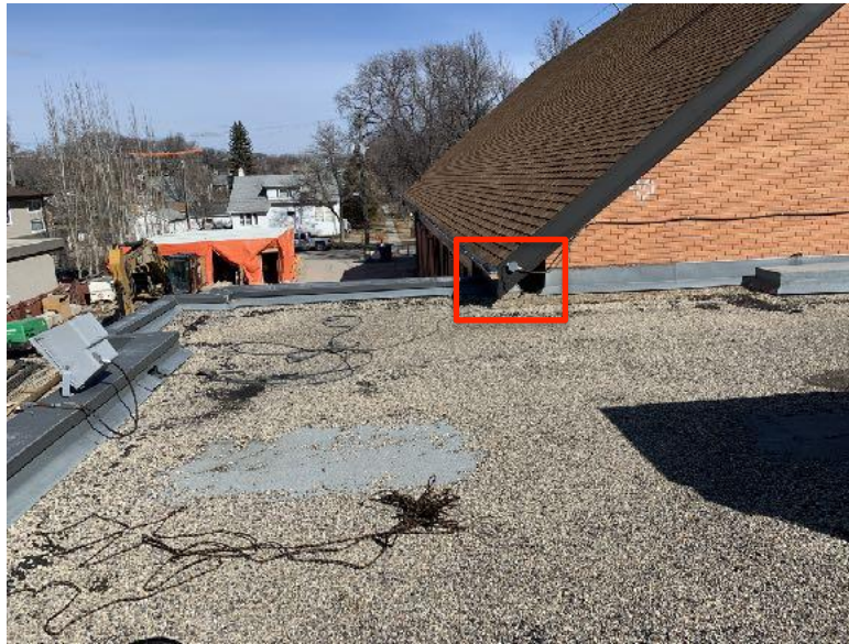
Fig. 3: Roof-A low-slope inset at steep-slope overhang to be boxed-out, insulated fully with batt insulation & sheathed to facilitate SBS roof assembly up-stand stripping.
