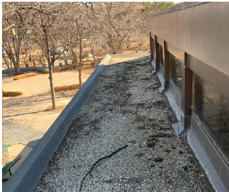
Fig. 9: Roof-A: Provide & install new A/C Platform curb.
