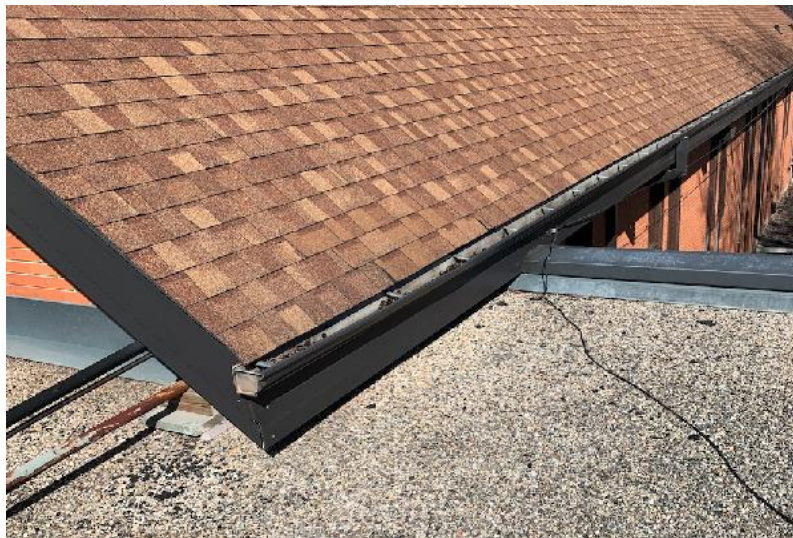
Fig. 3: Roof-A low-slope inset at steep-slope overhang to be boxed-out, insulated fully with batt insulation & sheathed to facilitate SBS roof assembly up-stand stripping.
