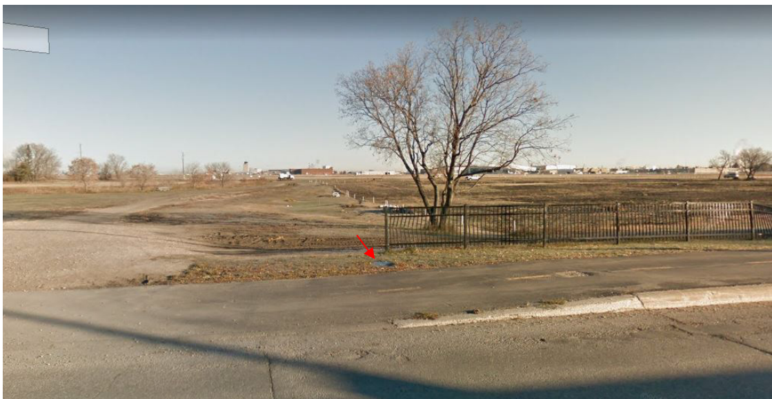
Site 9 – 750 manhole lid to air release valve, looking north from Silver Avenue.
