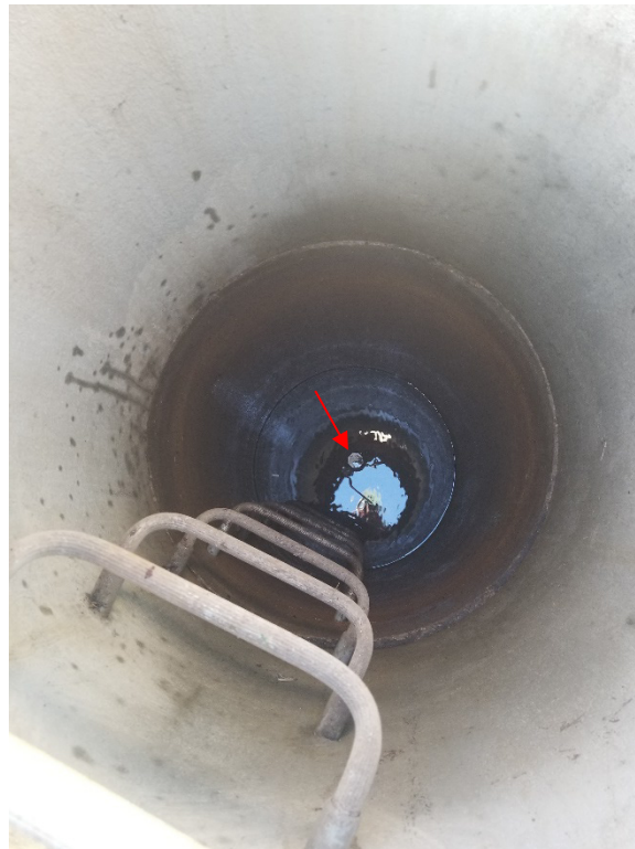
Site 9 - Existing air release valve in existing 750 manhole, looking south.
