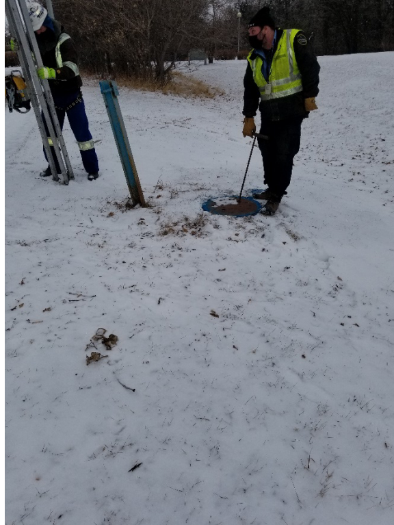
Site 10 – South chamber cover, looking north.
