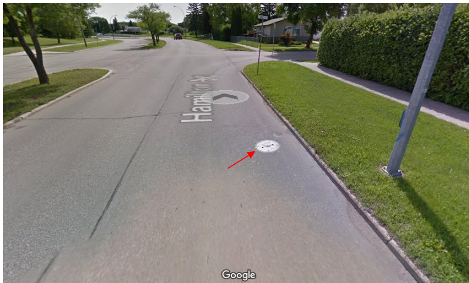
Site 7 – Existing manhole cover to valve chamber, eastbound Hamilton Avenue looking east.
