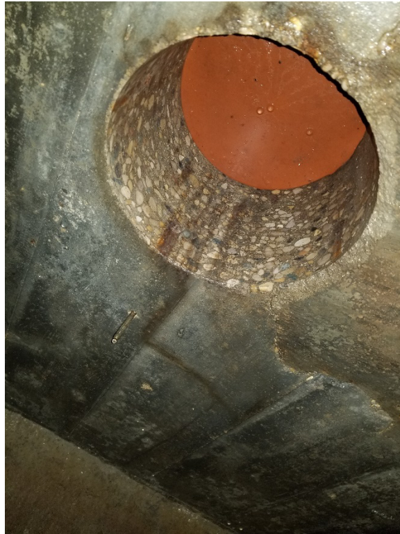
Site 10 - Existing core hole in south chamber roof slab, looking north.
