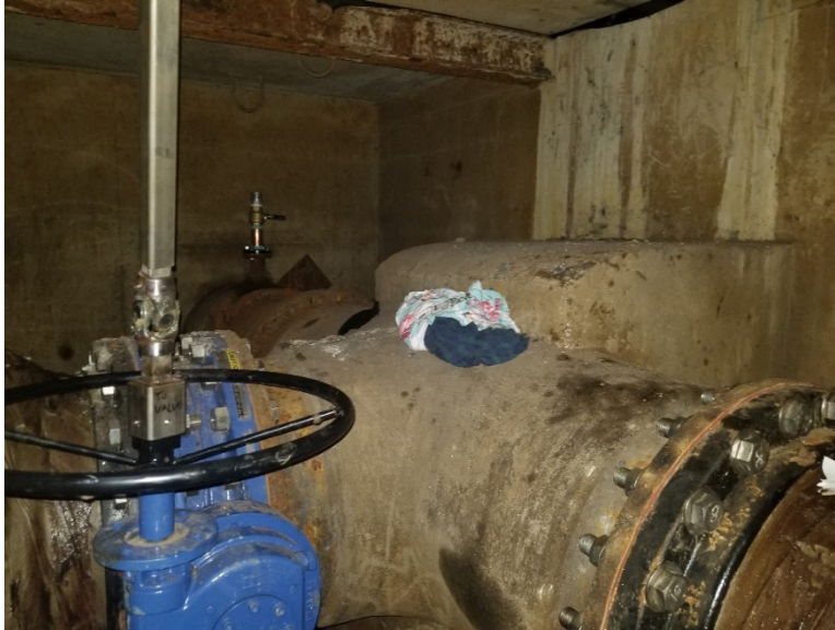
Site 11 – General layout of chamber, looking northwest.
