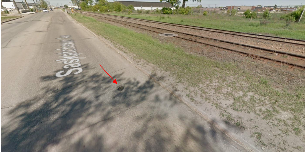
Site 8 – Existing air release valve in roadway, looking north.
