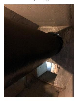
Site 1 – 500 mm FRM at south abutment wall, typical access hole in box girders.
