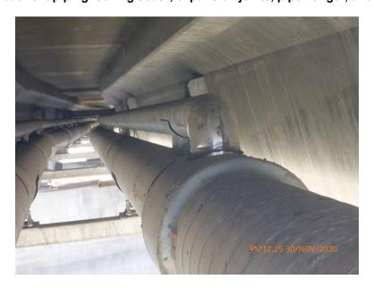
Site 2 – Air release connection at mid span of bridge, looking west.
