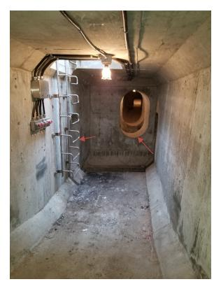
Site 3 – Hatch access girder looking west, pier access hole (west), bridge girder access hole (south).
