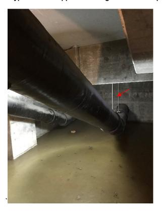
Site 1 – South abutment chamber looking south, wall penetration, hanger supports, elbow and couplers.
