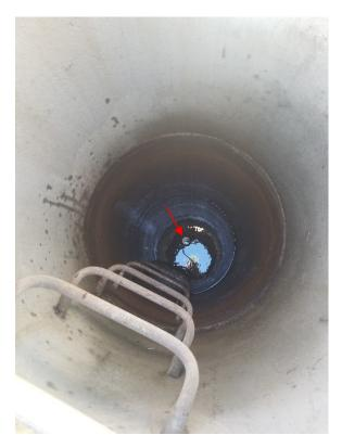
Site 9 - Existing air release valve in existing 750 manhole, looking south.
