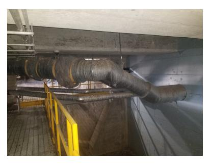
Site 2 – West abutment piping looking south, expansion joints, pipe hanger, and welded joints.
