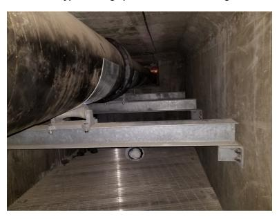
Site 3 – Force main piping and typical inspection platform at bridge piers.
