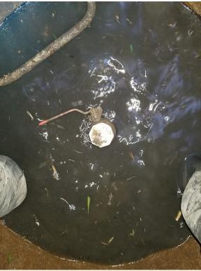
Site 9 – Existing air release valve in existing 750 manhole.
