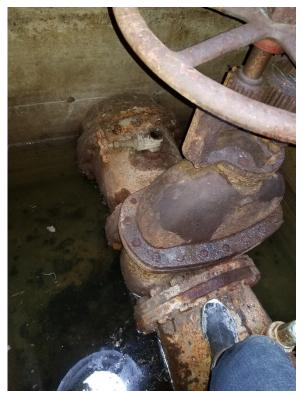
Site 10 – Existing 50 mm air valve in south chamber, looking north.
