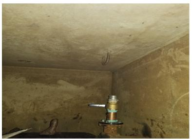
Site 11 – Existing 50 mm air valve and roof slab in chamber located west of McPhillips Street.
