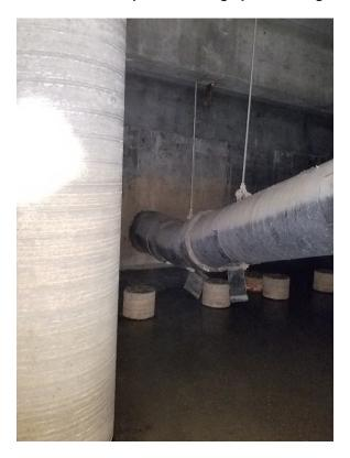
Site 3 – North abutment looking northeast, wall penetration, elbow, couplers, expansion joint, and hanger supports.
