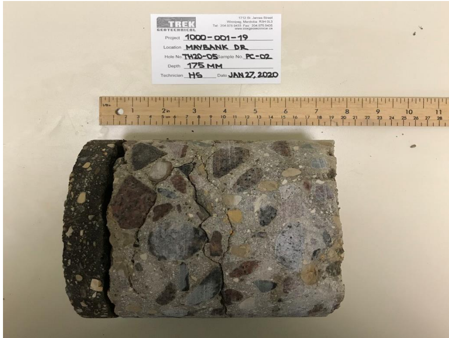
Photo 5: Pavement Core Sample at Test Hole TH20-05
