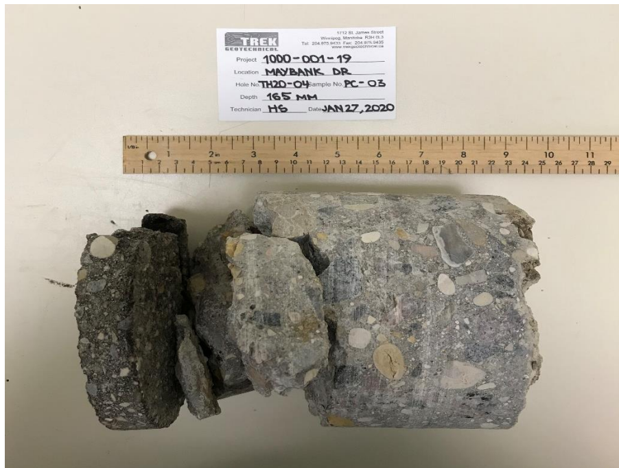
Photo 4: Pavement Core Sample at Test Hole TH20-04
