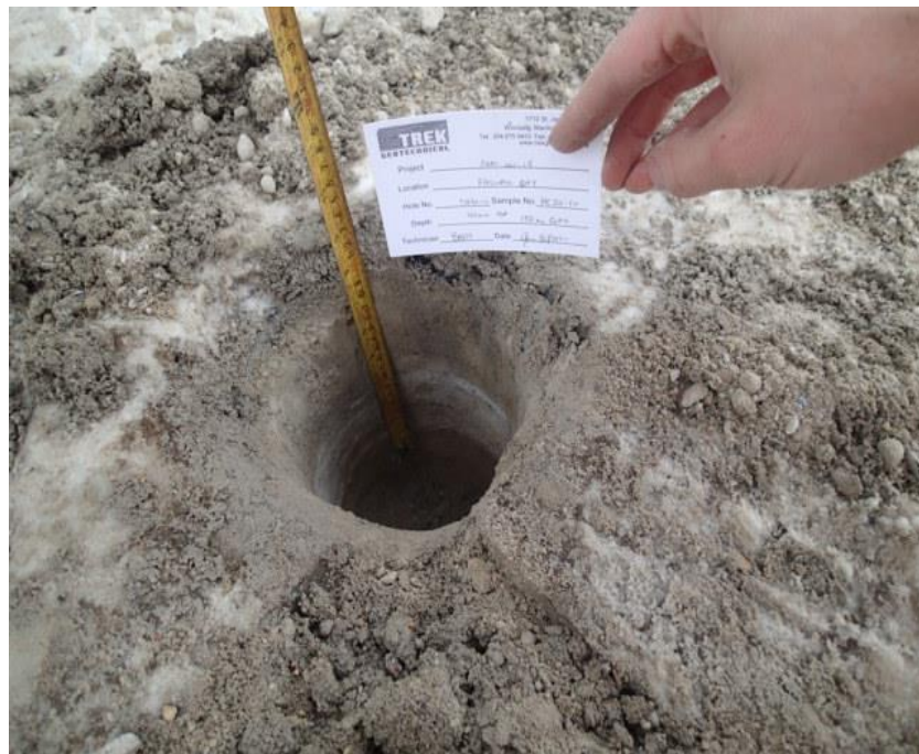
Photo 4: Pavement Core Measurement at Test Hole TH20-10
