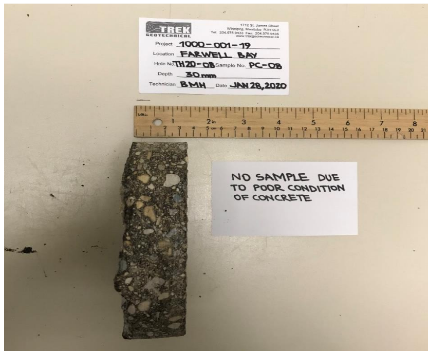
Photo 2: Pavement Core Sample at Test Hole TH20-08
