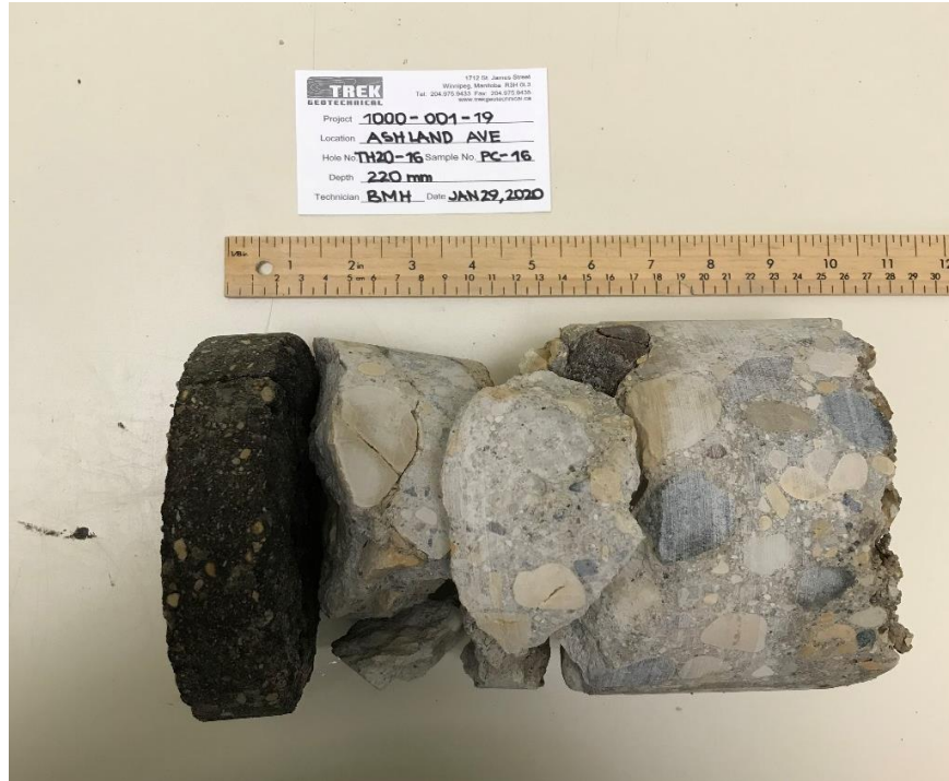
Photo 1: Pavement Core Sample at Test Hole TH20-16
