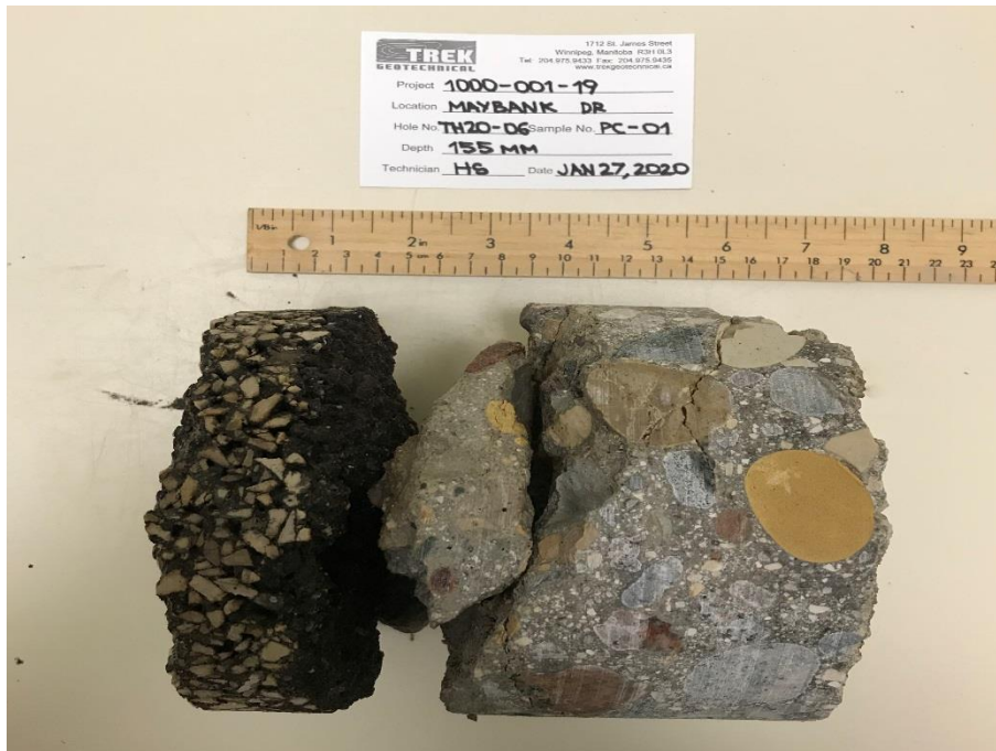
Photo 6: Pavement Core Sample at Test Hole TH20-06
