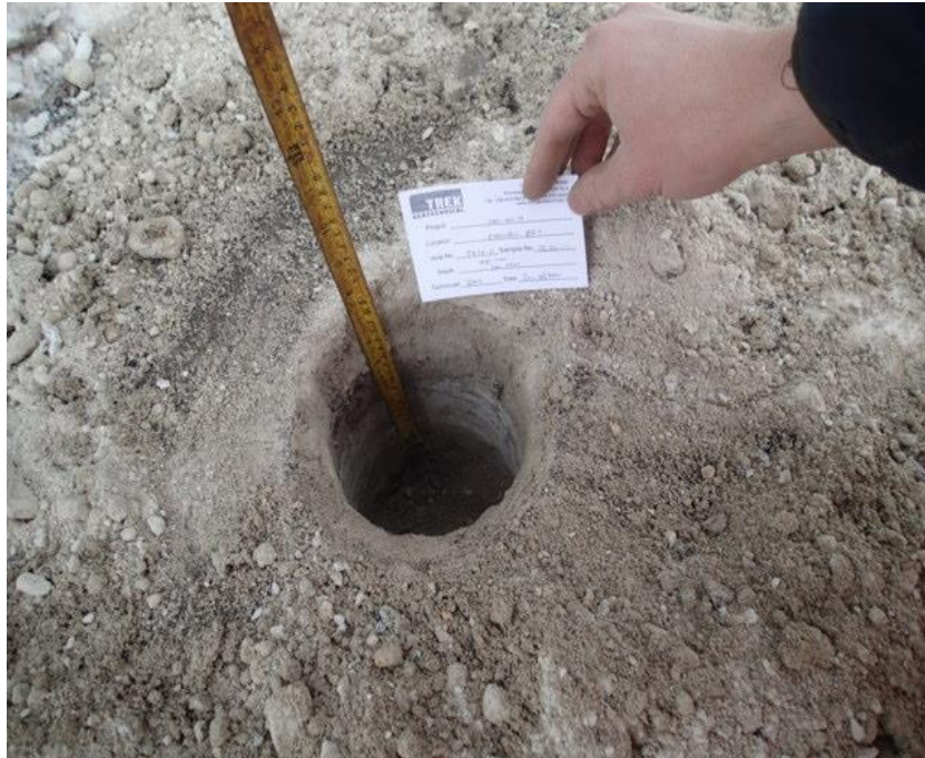
Photo 5: Pavement Core Measurement at Test Hole TH20-11
