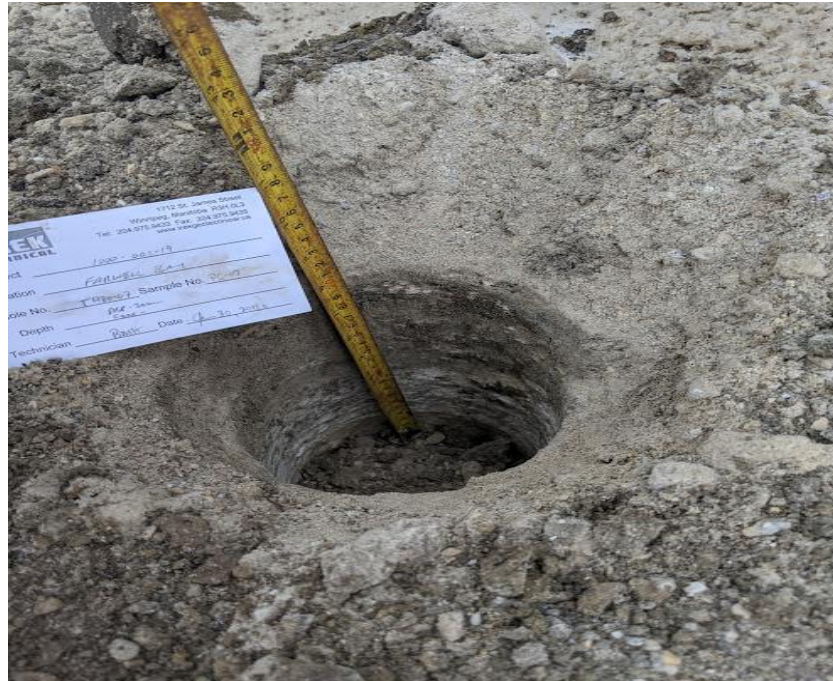
Photo 1: Pavement Core Measurement at Test Hole TH20-07
