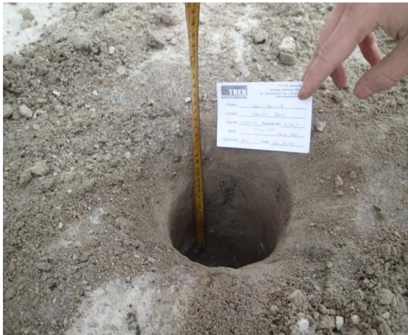
Photo 6: Pavement Core Measurement at Test Hole TH20-12
