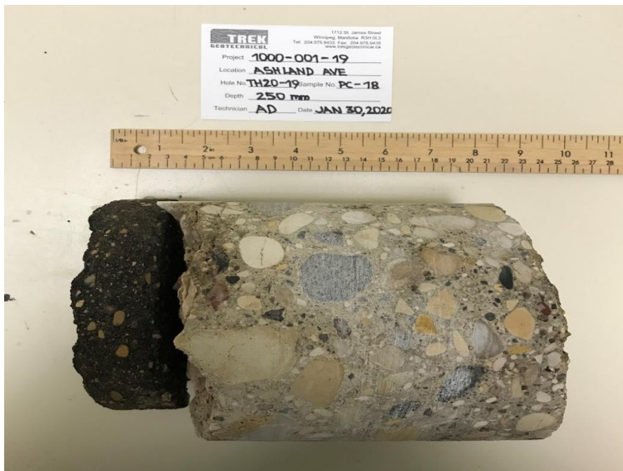
Photo 4: Pavement Core Sample at Test Hole TH20-19
