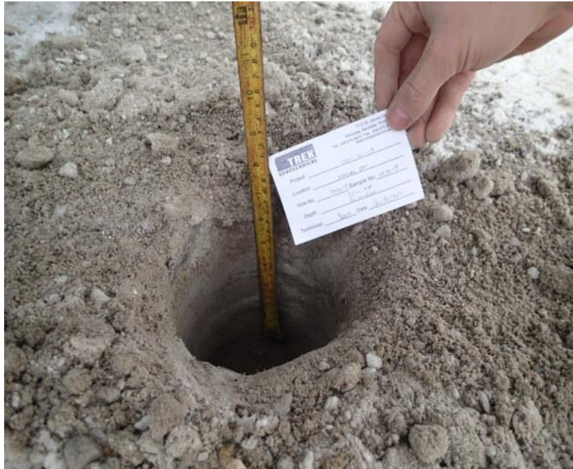
Photo 7: Pavement Core Measurement at Test Hole TH20-13
