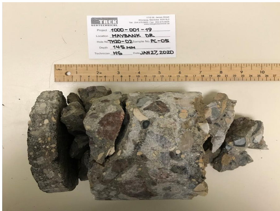
Photo 2: Pavement Core Sample at Test Hole TH20-02
