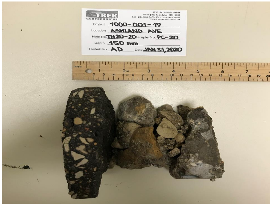
Photo 5: Pavement Core Sample at Test Hole TH20-20
