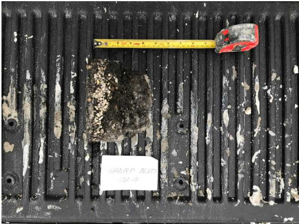
Photograph 4: Core Hole CH20-04 – Sharp Boulevard – Concrete not recovered
