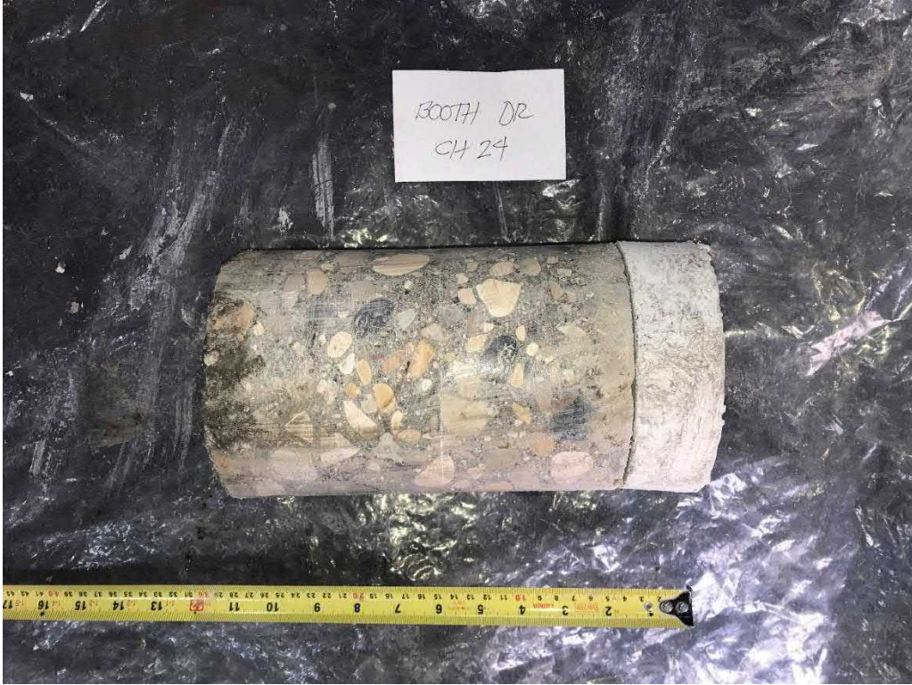
Photograph 23: Core Hole CH20-24 – Booth Drive
