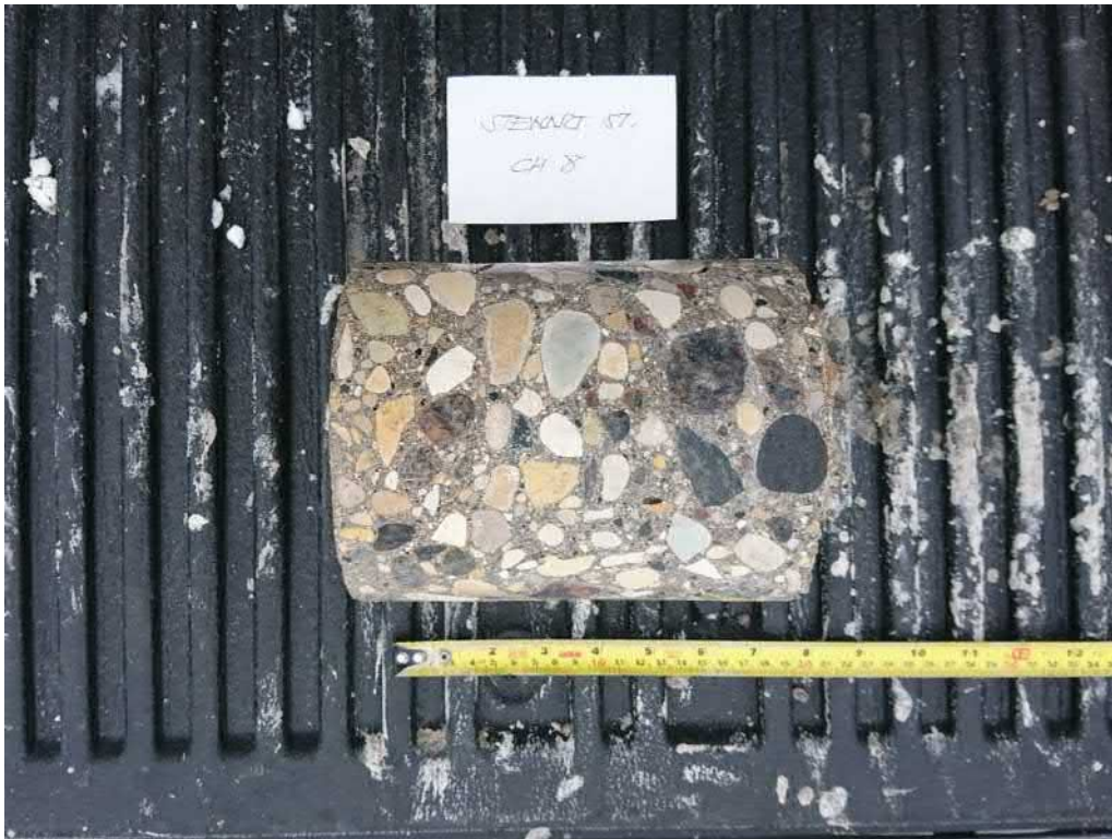
Photograph 8: Core Hole CH20-08 – Stewart Street
