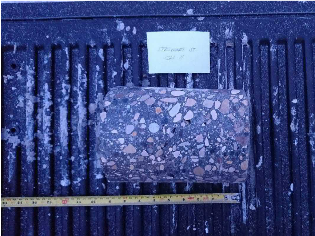
Photograph 10: Core Hole CH20-11 – Stewart Street
