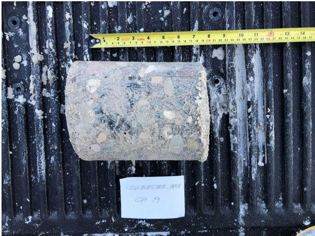
Photograph 18: Core Hole CH20-19 – Colchester Bay
