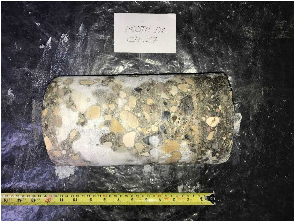
Photograph 26: Core Hole CH20-27 – Booth Drive
