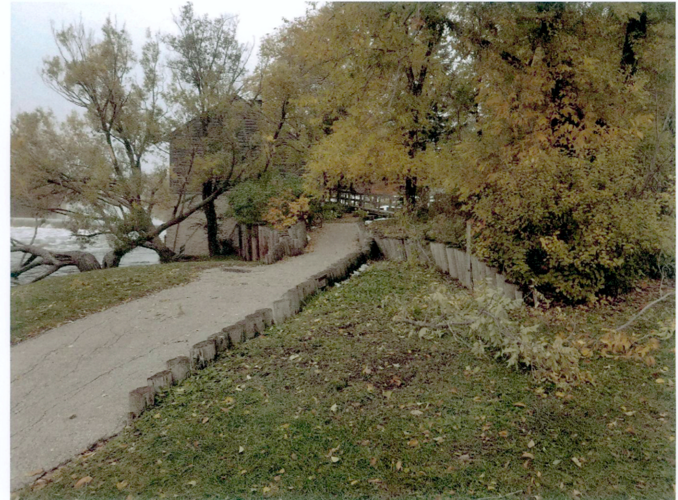
PHOTO 'A' (TO BE REMOVED AND REPLACED)
