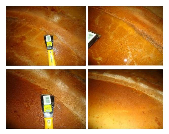
Photo Set 12: Tank floor seam bonding – delamination (lifting)
