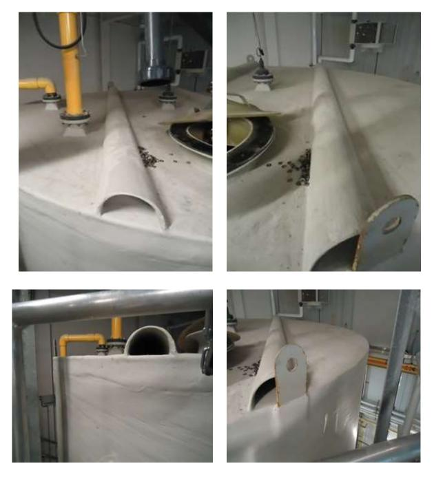
Photo Set 6: Appurtenances – Lid Rib and Lifting Lugs
