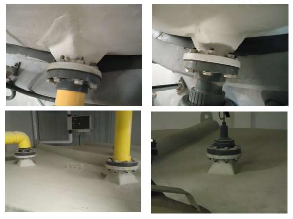
Photo Set 4: Tank Appurtenances – Flanged Nozzles (outside view)
