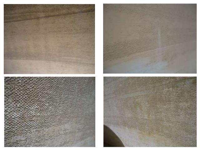
Photo Set 9: Close up view of the dryness and roughness of the compromised tank liner
