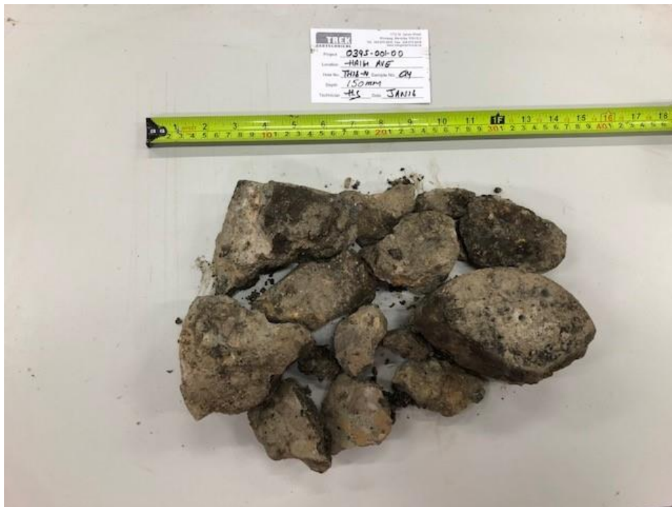
Photo 2: Pavement Core Sample at Test Hole TH17-14
