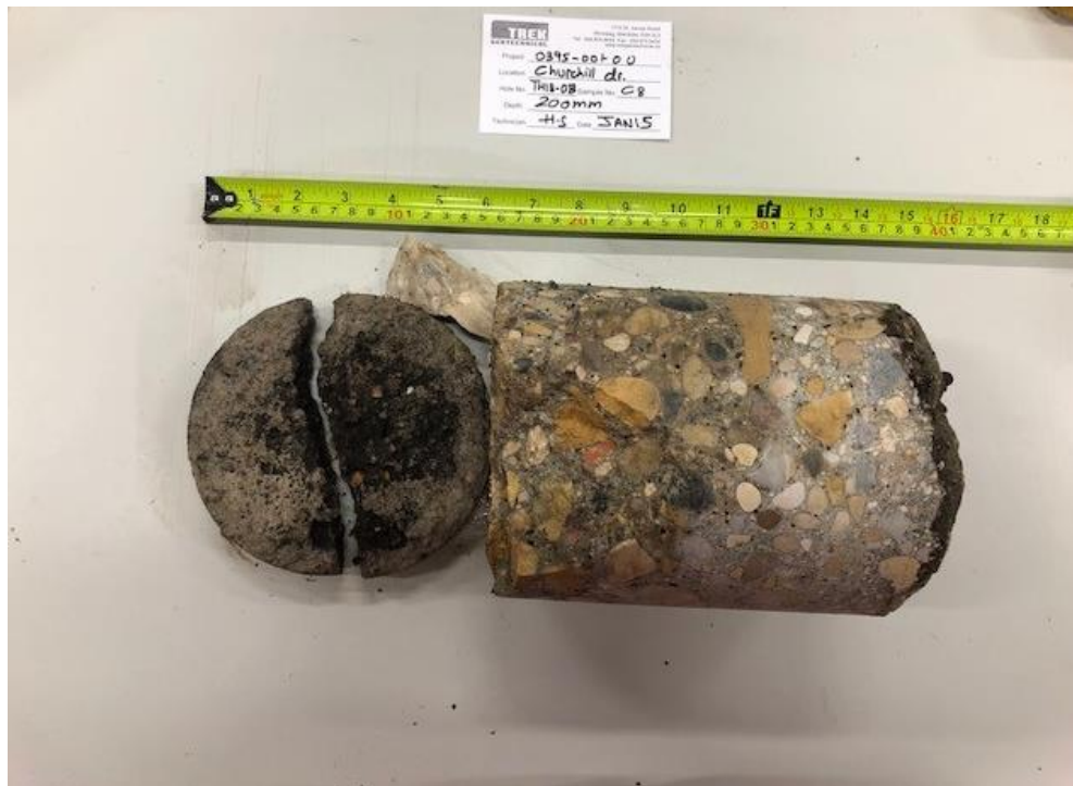
Photo 2: Pavement Core Sample at Test Hole TH17-08
