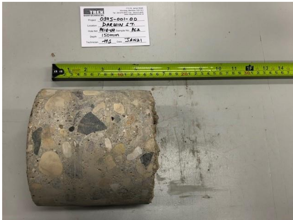
Photo 2: Pavement Core Sample at Test Hole PC18-02
