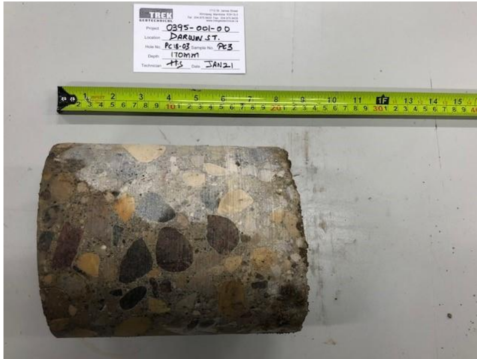
Photo 3: Pavement Core Sample at Test Hole PC18-03
