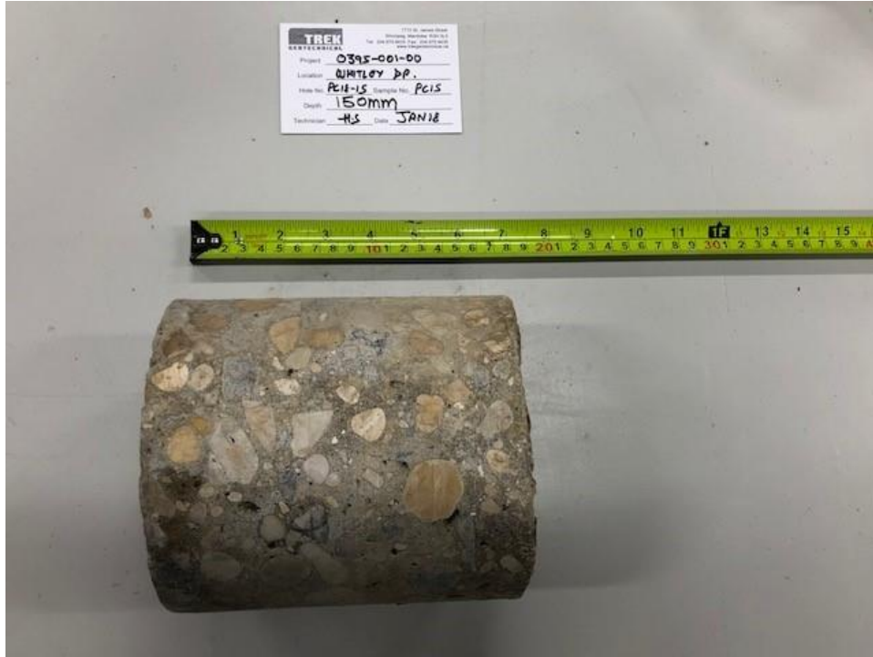
Photo 3: Pavement Core Sample at Test Hole PC18-15
