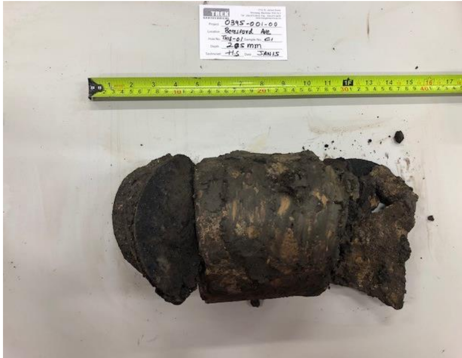
Photo 1: Pavement Core Sample at Test Hole TH17-01
