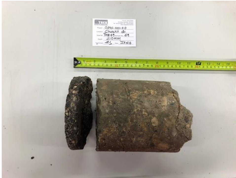
Photo 3: Pavement Core Sample at Test Hole TH17-09
