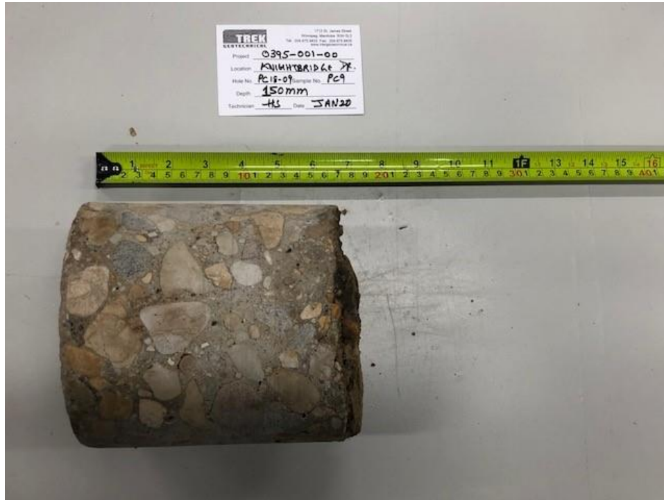
Photo 3: Pavement Core Sample at Test Hole PC18-09
