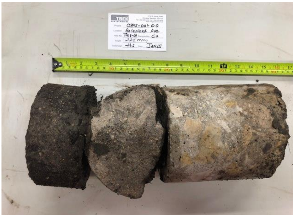
Photo 2: Pavement Core Sample at Test Hole TH17-02
