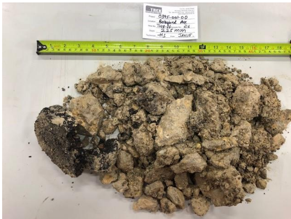
Photo 6: Pavement Core Sample at Test Hole TH17-06
