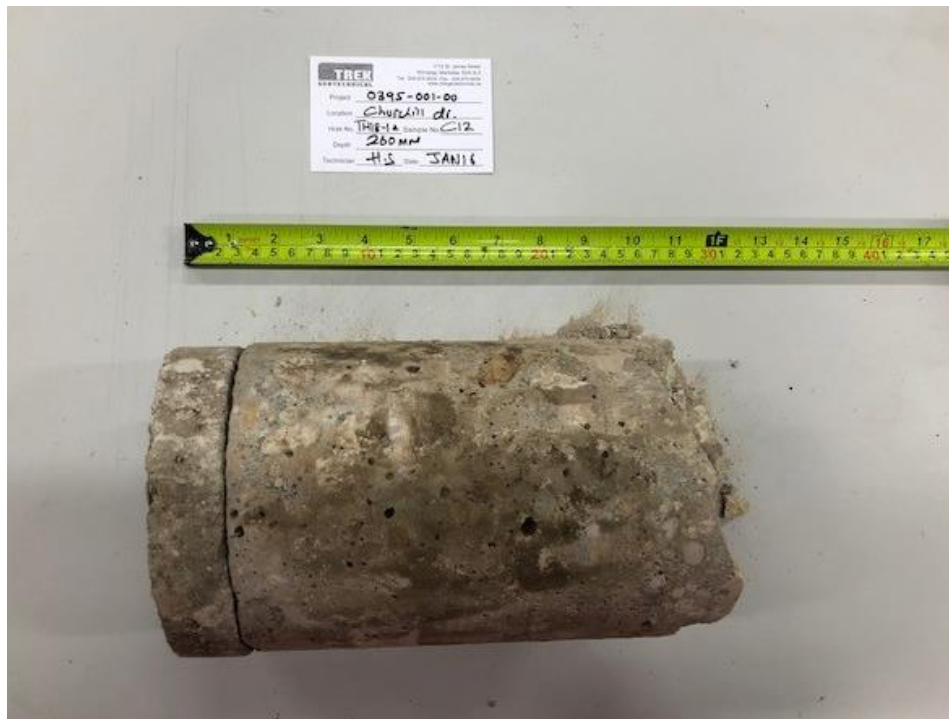
Photo 6: Pavement Core Sample at Test Hole TH17-12
