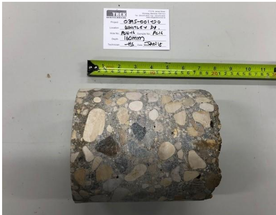
Photo 4: Pavement Core Sample at Test Hole PC18-16
