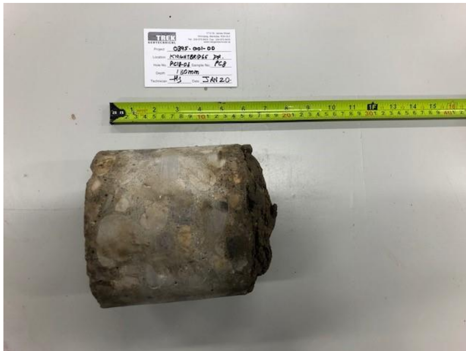
Photo 2: Pavement Core Sample at Test Hole PC18-08
