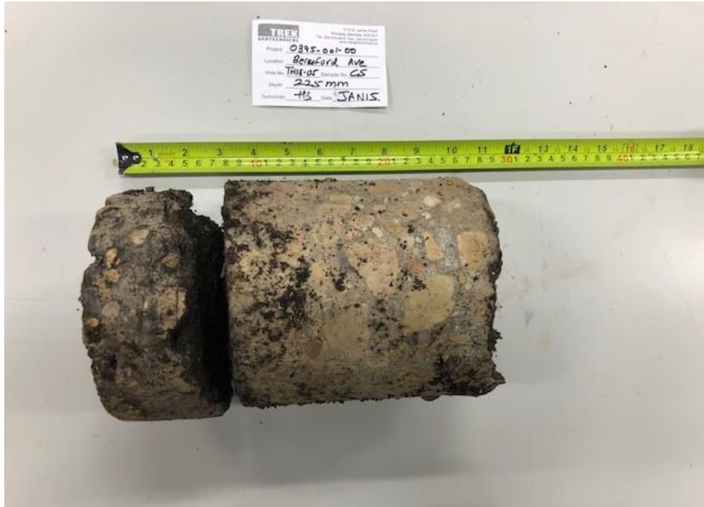
Photo 5: Pavement Core Sample at Test Hole TH17-05
