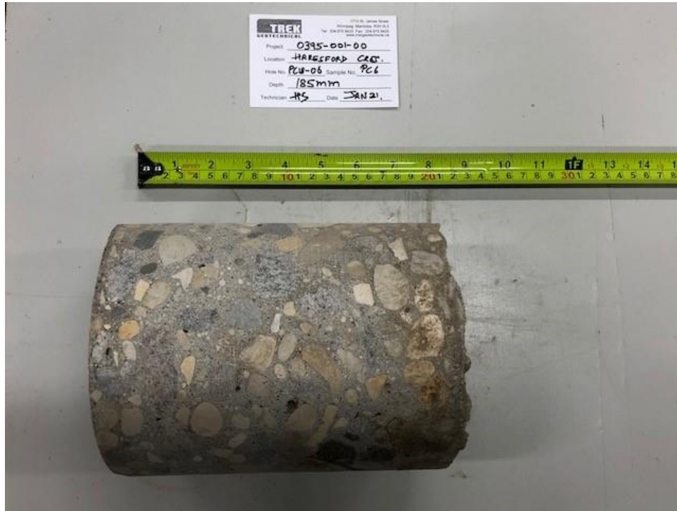
Photo 3: Pavement Core Sample at Test Hole PC18-06
