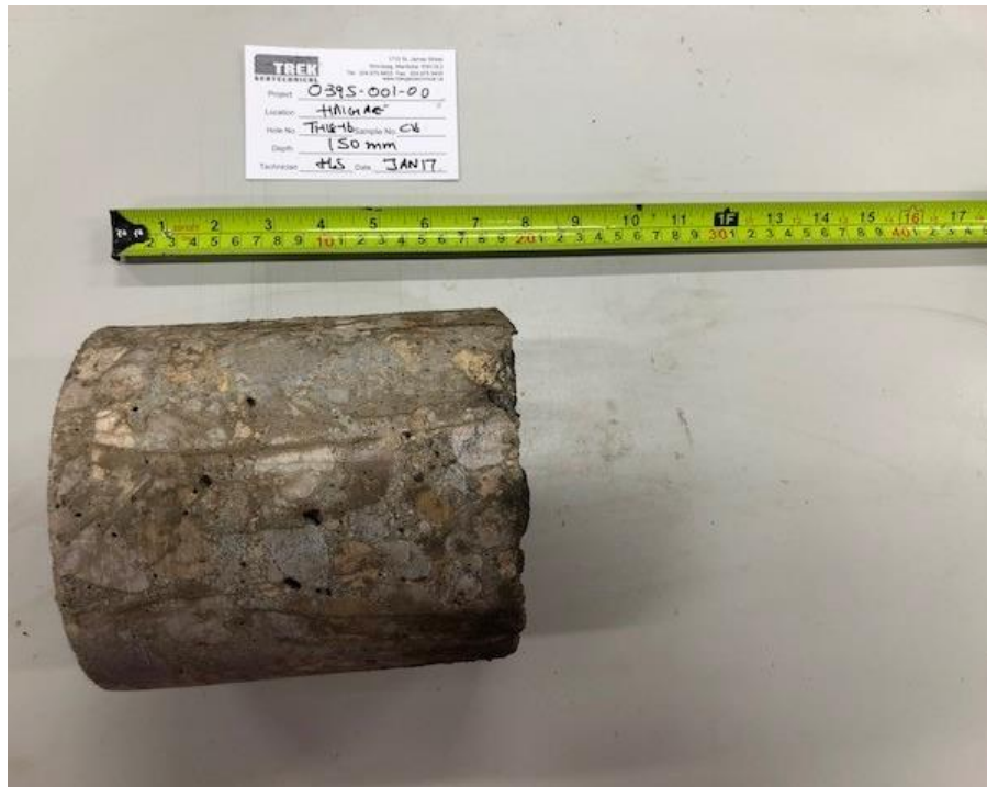
Photo 4: Pavement Core Sample at Test Hole TH17-16
