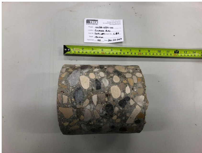
Photo 6: Pavement Core Sample at Test Hole TH17-14
