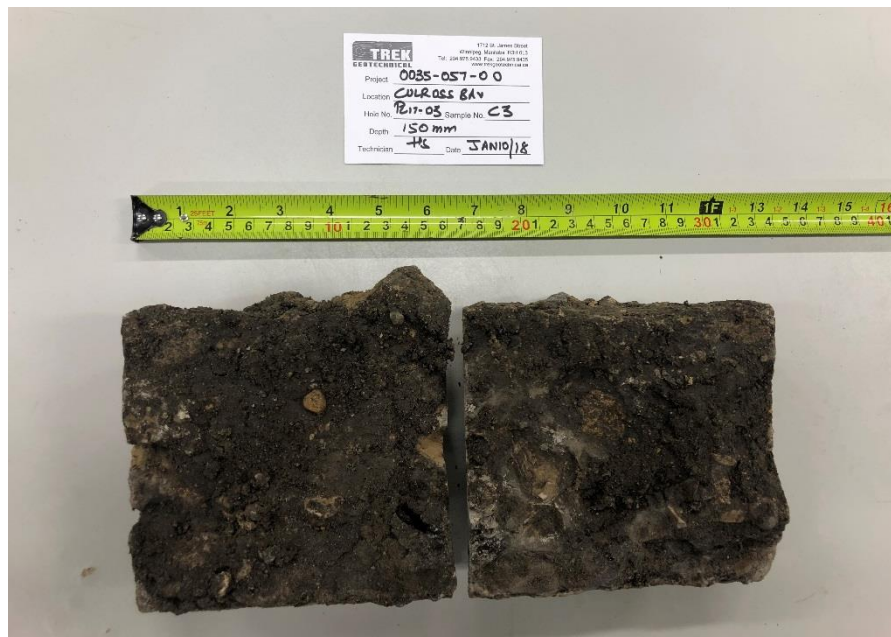
Photo 10: Pavement Core Sample at Pavement Hole PC17-03
