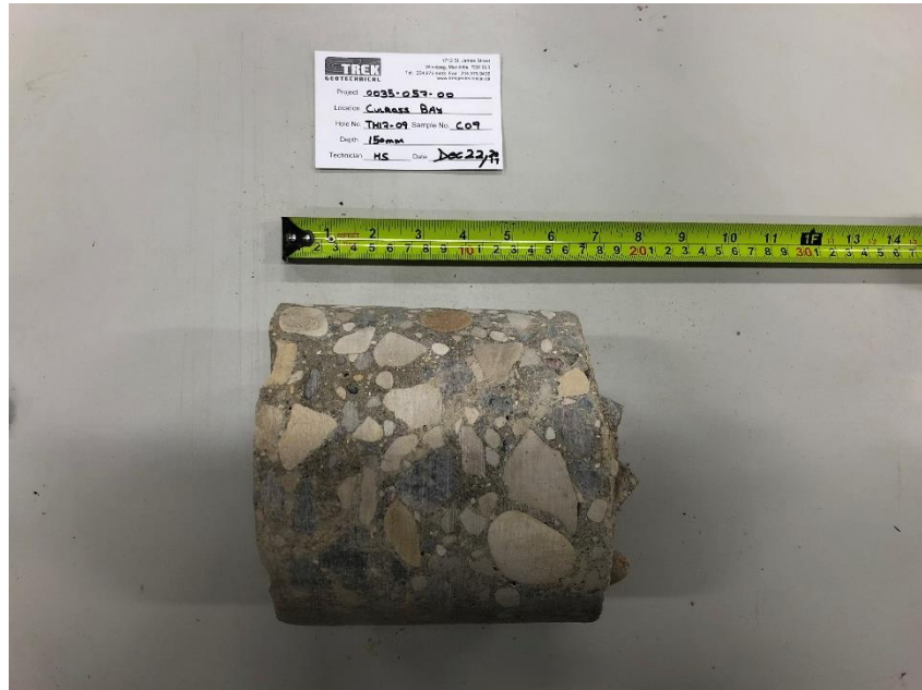
Photo 1: Pavement Core Sample at Test Hole TH17-09
