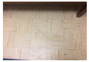
Photo #8: Asbestos-containing floor itles within the staff room and childrens readinfg room.
