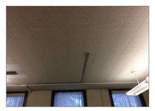
Photo #1: Non-asbestos acoustic ceiling tiles within the basement washrooms and meeting room.
