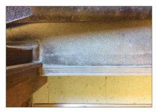
Photo #3: Non-asbestos vinyl sheet flooring with rubber backing within bathrooms.
