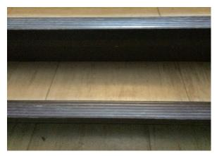
Photo #9: Asbestos-containing vinyl floor tiles within the back stairwell.
