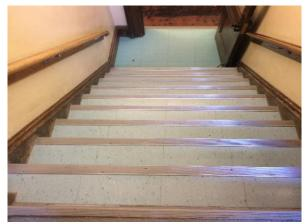
Photo #6: Non-asbestos floor tiles installed after 2000 within the stairwell.
