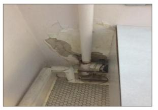
Photo #2: 6 SF of damaged plaster wall finish within the basement women's washroom.
