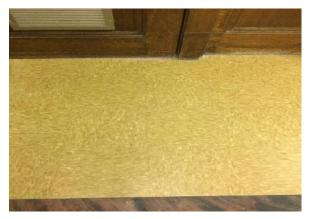
Photo #7: Non-asbesots repalcement tiles installed after 2000.
