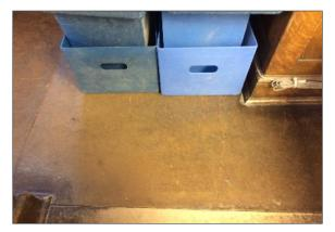
Photo #4: Non-asbestos battleship flooring within the storage mezzanine.
