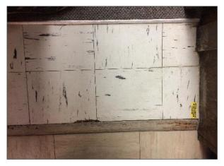
Photo #5: Asbestos-containing green and white floor tiles under carpet within the main floor library.
