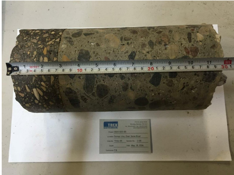
Photo 5: Pavement Core Sample at Test Hole TH16-05
