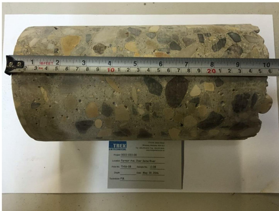
Photo 8: Pavement Core Sample at Test Hole TH16-08
