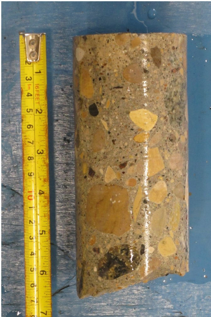
Figure 13 – Core no. P1, east pier
