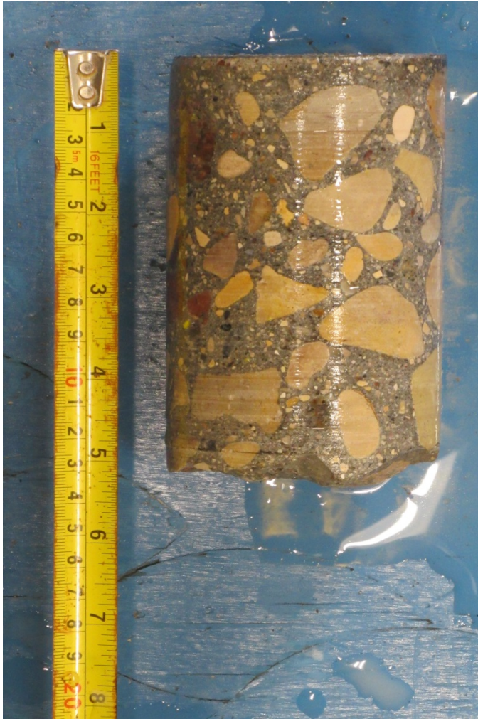
Figure 21 – Core no. A1, east abutment
