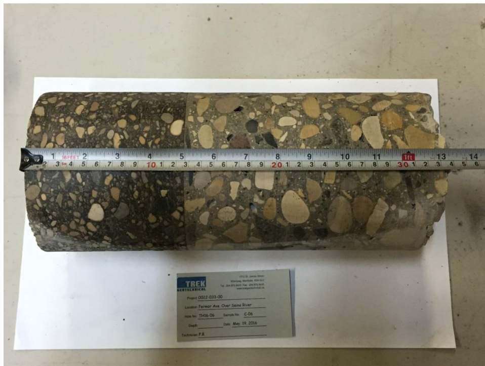
Photo 6: Pavement Core Sample at Test Hole TH16-06
