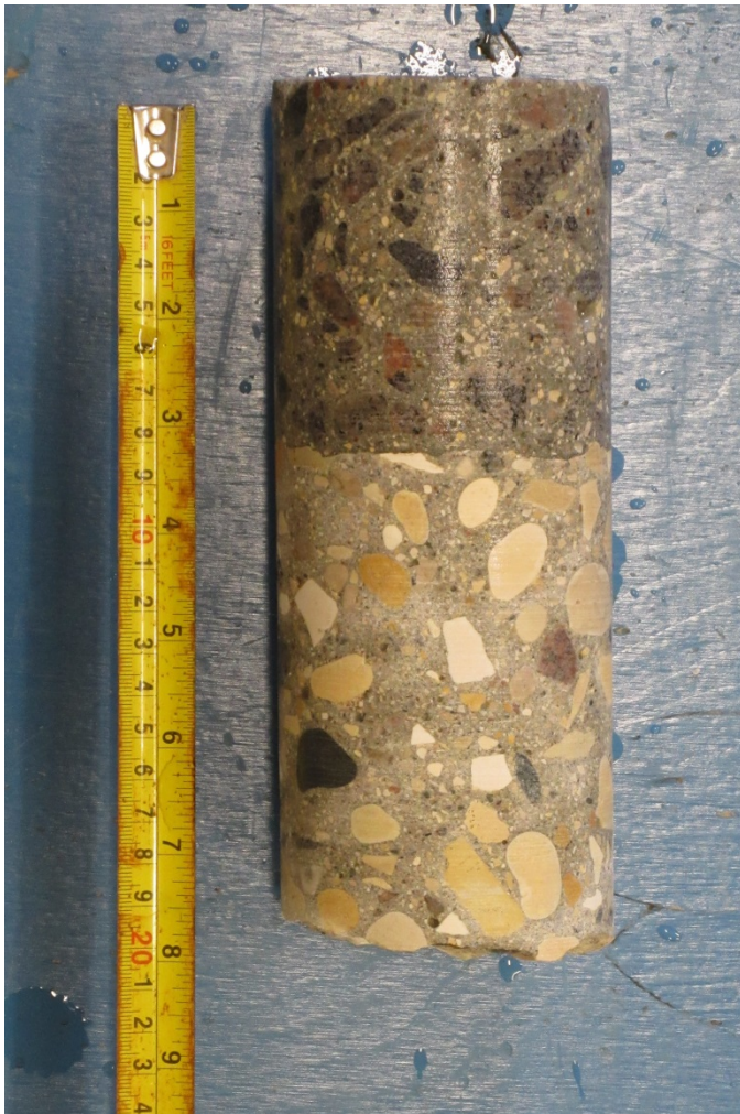
Figure 5 – Core no. D5, eastbound curb lane
