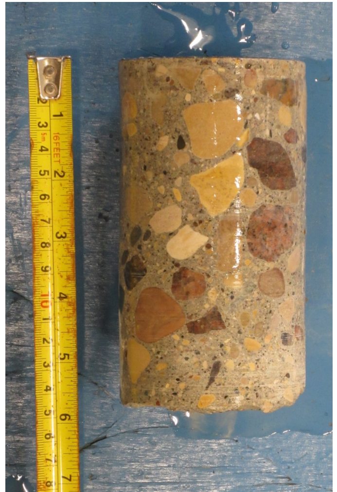
Figure 14 – Core no. P2, east pier
