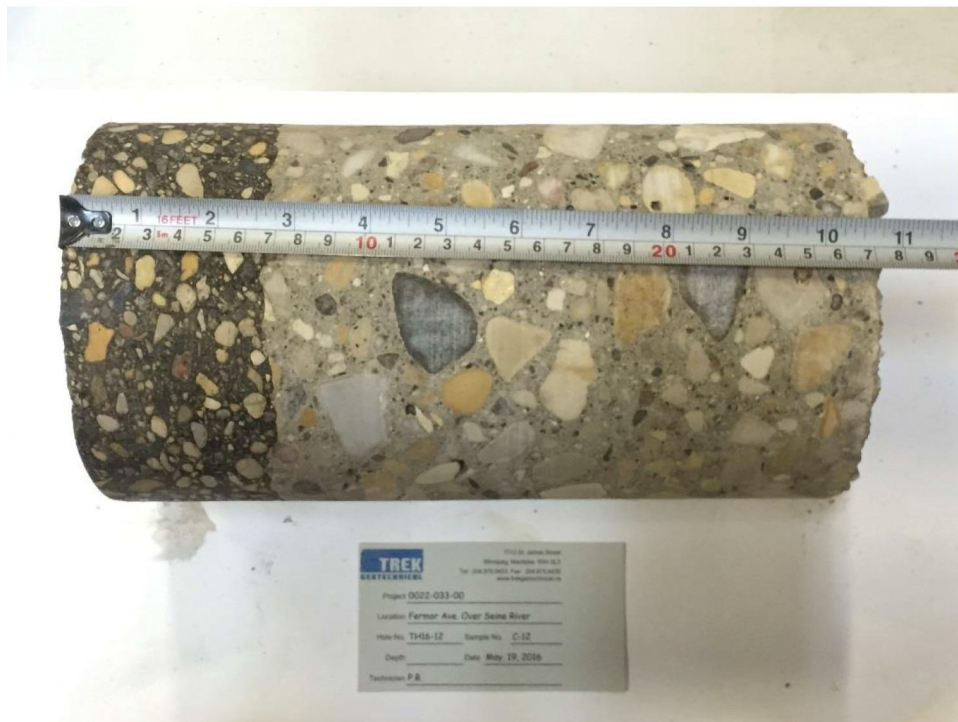
Photo 12: Pavement Core Sample at Test Hole TH16-12
