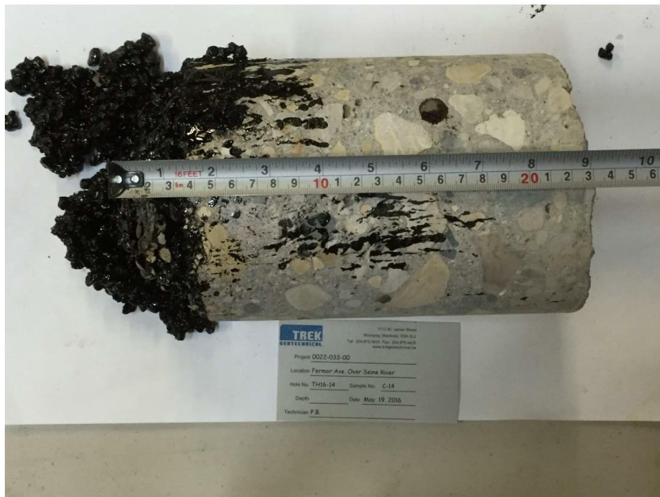
Photo 14: Pavement Core Sample at Test Hole TH16-14
