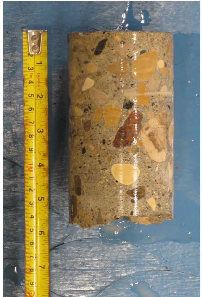
Figure 18 – Core no. P6, west pier
