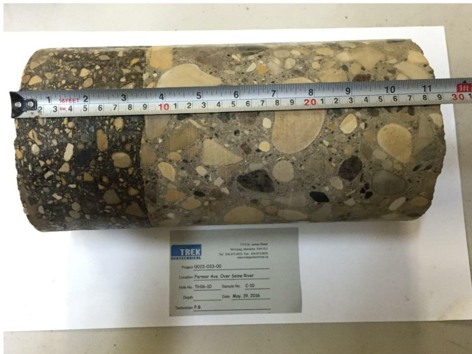
Photo 10: Pavement Core Sample at Test Hole TH16-10
