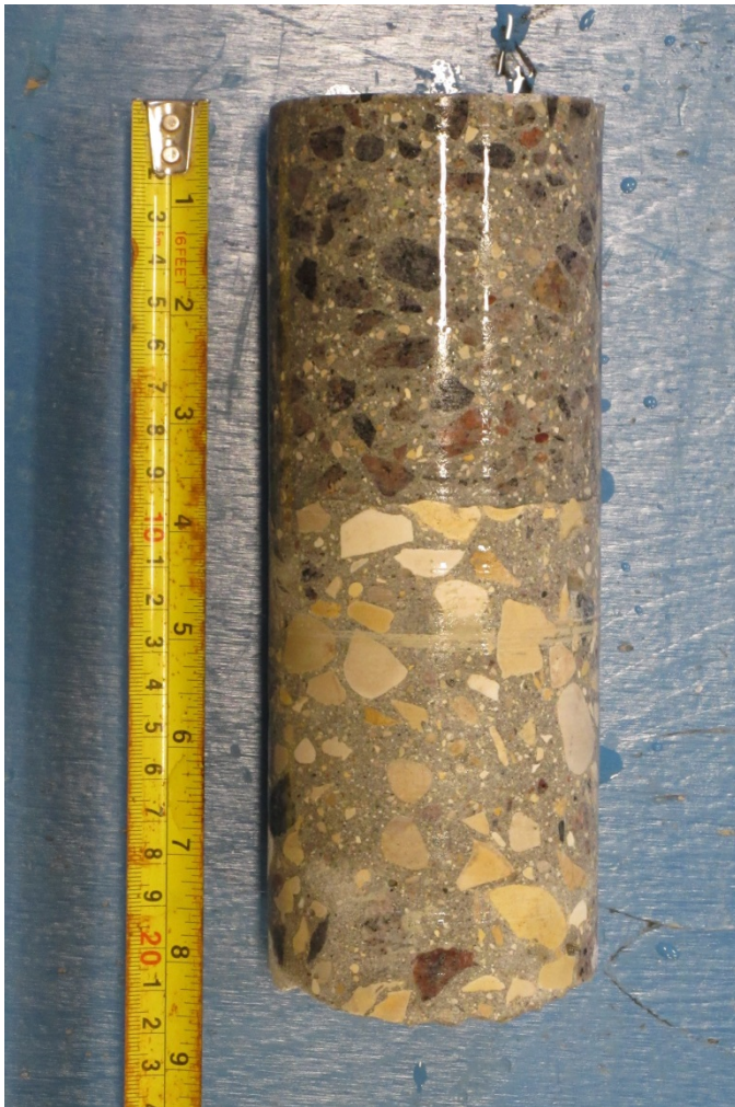
Figure 3 – Core no. D3, eastbound curb lane
