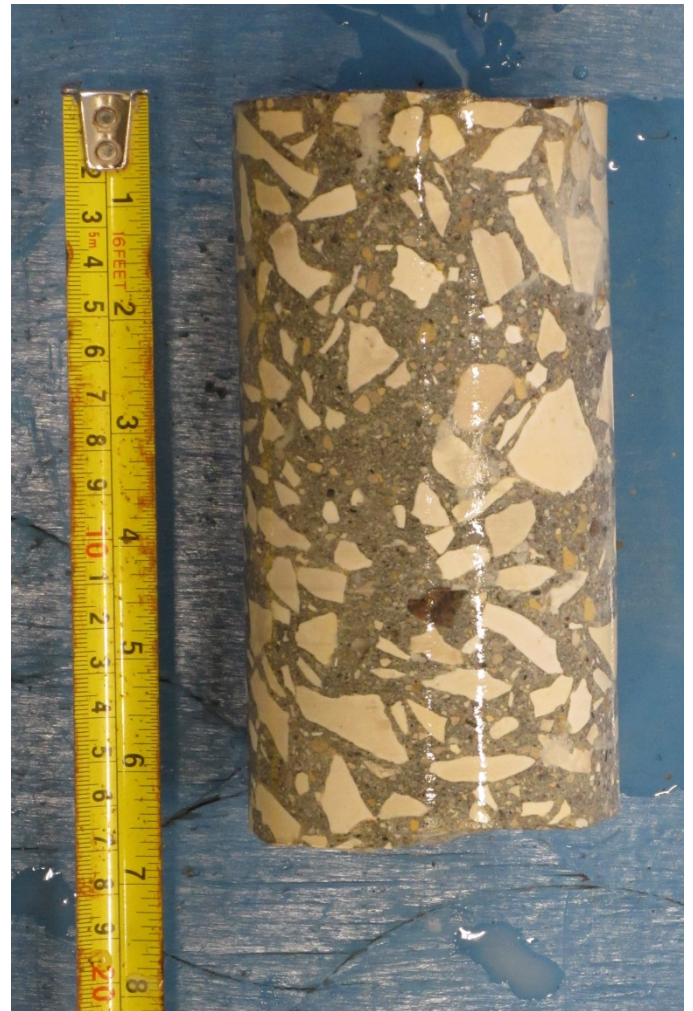
Figure 20 – Core no. P8, west pier
