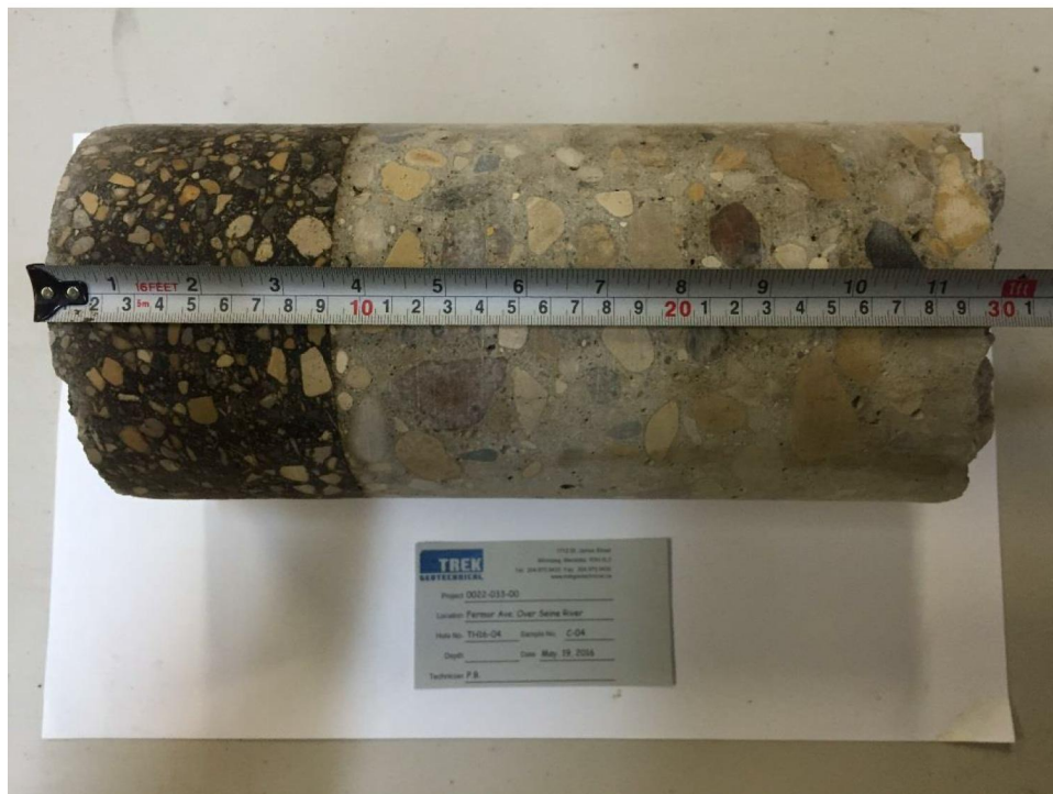
Photo 4: Pavement Core Sample at Test Hole TH16-04
