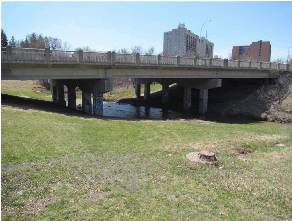
Photo No. 2 Downstream side of Fermor Avenue Crossing
