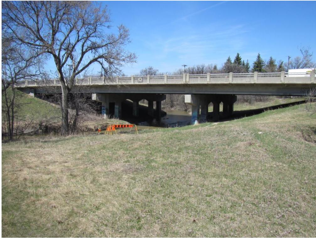
Photo No. 3 Upstream side of Fermor Avenue Crossing
