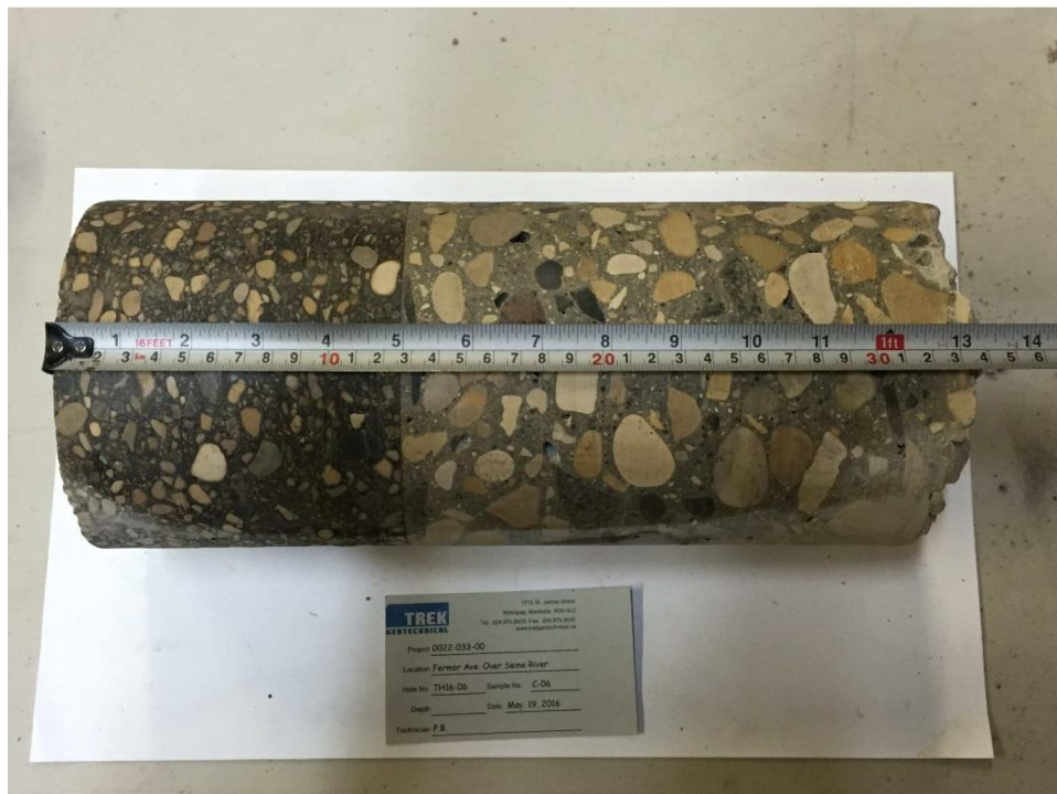
Photo 6: Pavement Core Sample at Test Hole TH16-06
