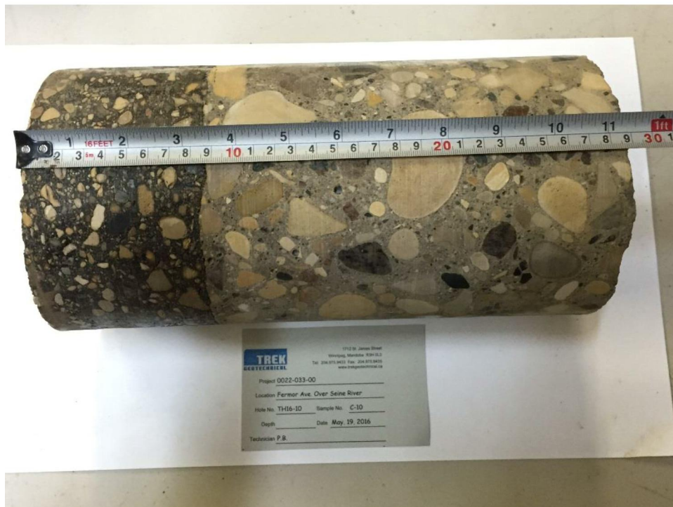
Photo 10: Pavement Core Sample at Test Hole TH16-10
