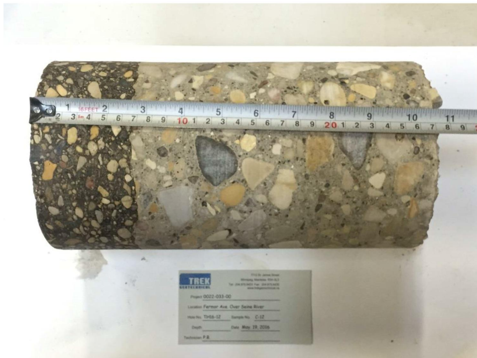
Photo 12: Pavement Core Sample at Test Hole TH16-12
