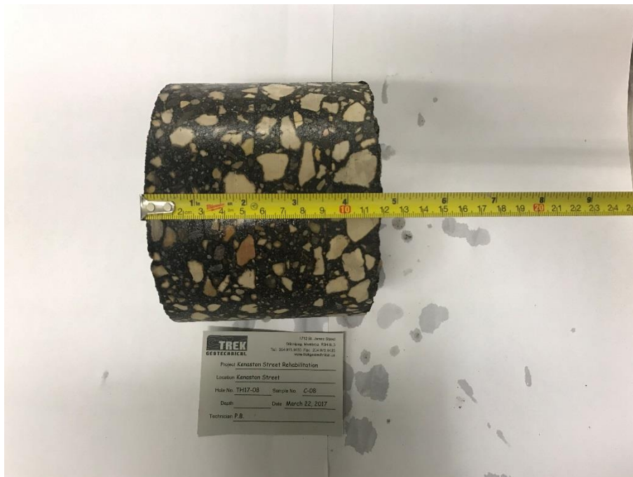
Photo 6: Pavement Core Sample at Test Hole TH17-08
