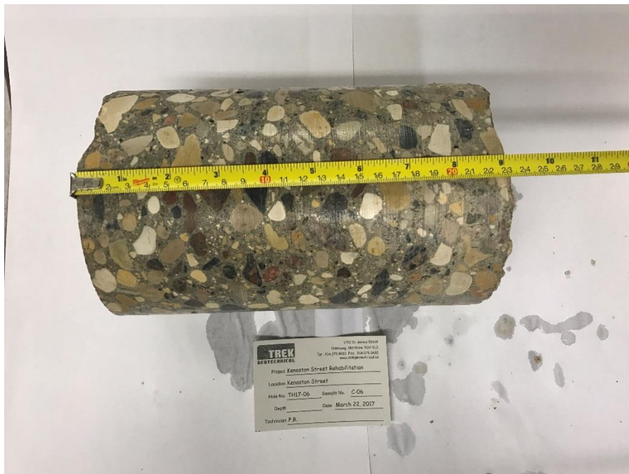
Photo 4: Pavement Core Sample at Test Hole TH17-06
