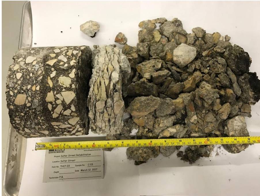
Photo 3: Pavement Core Sample at Test Hole TH17-03
