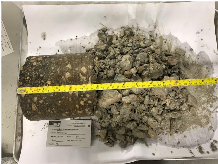
Photo 4: Pavement Core Sample at Test Hole TH17-04
