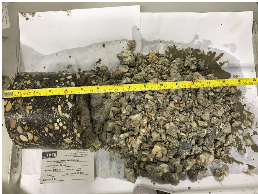
Photo 2: Pavement Core Sample at Test Hole TH17-02
