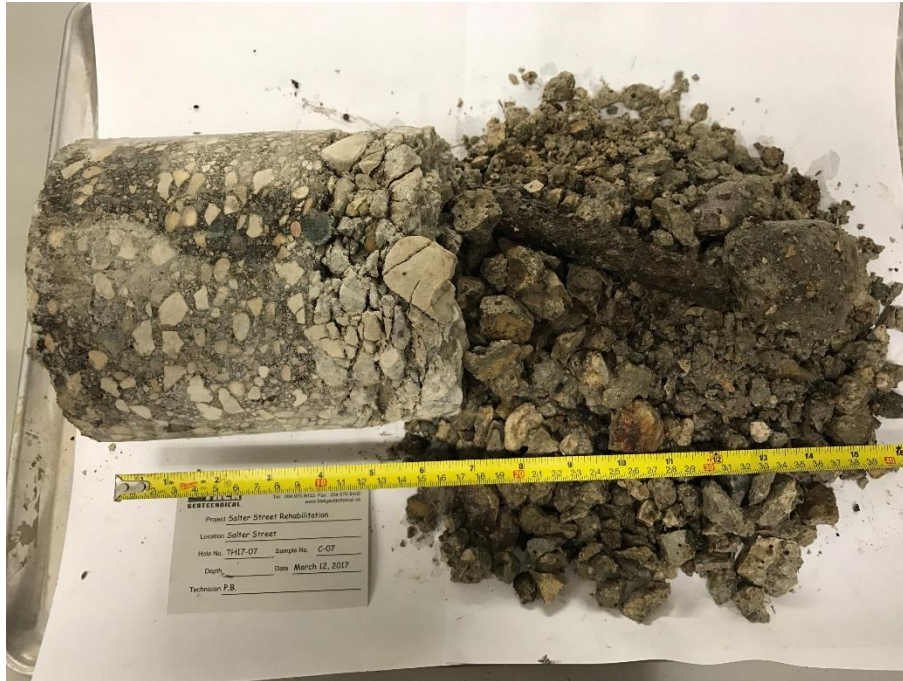
Photo 7: Pavement Core Sample at Test Hole TH17-07
