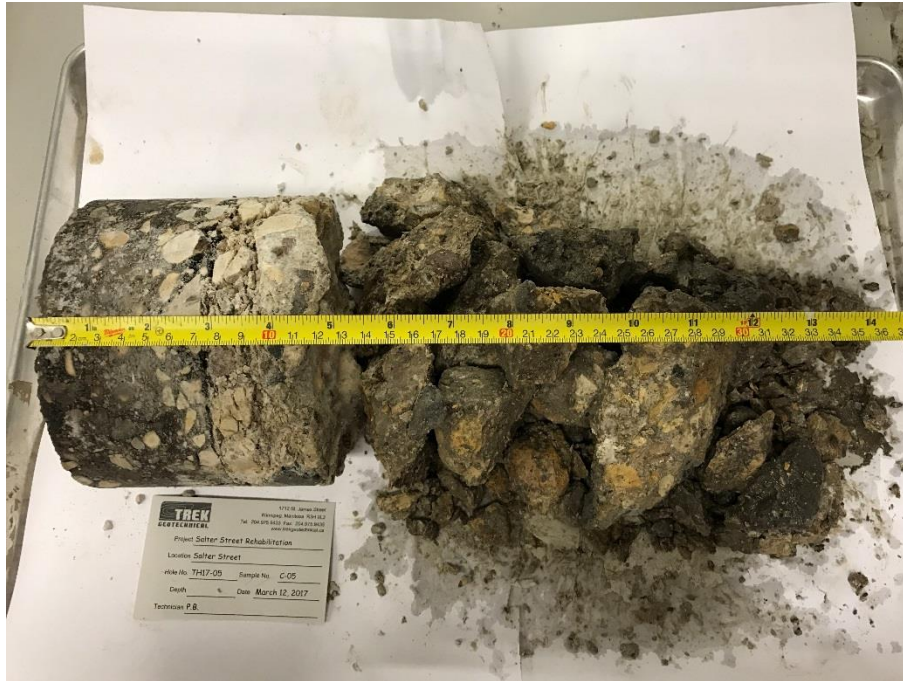
Photo 5: Pavement Core Sample at Test Hole TH17-05
