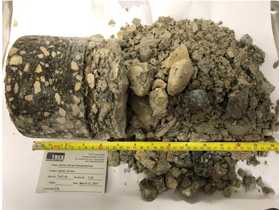
Photo 1: Pavement Core Sample at Test Hole TH17-01
