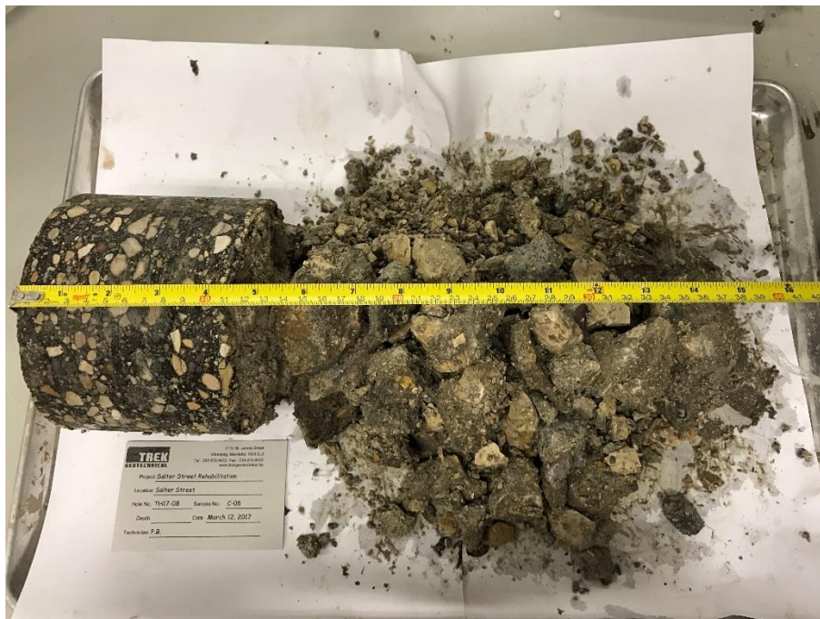
Photo 8: Pavement Core Sample at Test Hole TH17-08
