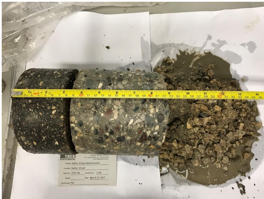
Photo 6: Pavement Core Sample at Test Hole TH17-06
