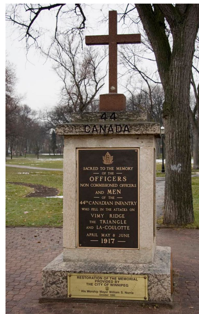
Vimy Ridge Monument To be removed and relocated onto new base. To be restored as required. Contractor is responsible for the care and safety of the monument during construction.
