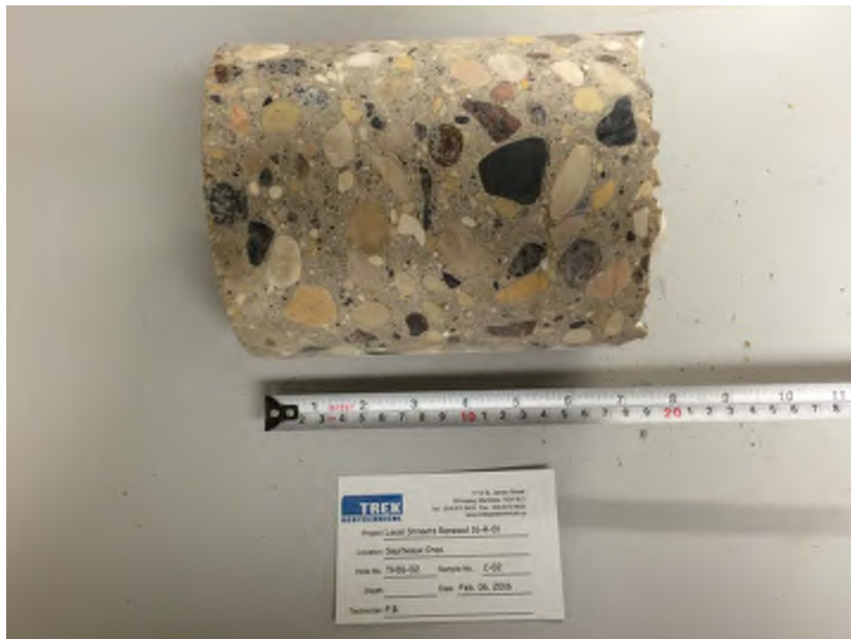
Photo 2: Pavement Core Sample at Test Hole TH16-02
