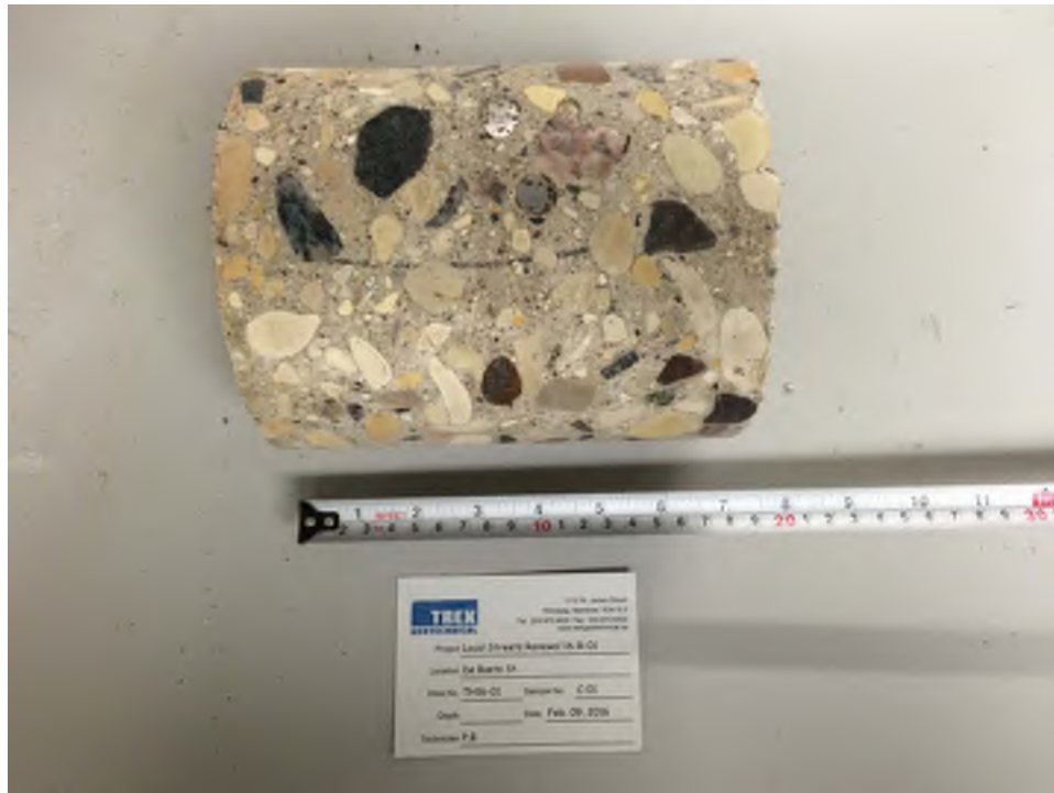
Photo 1: Pavement Core Sample at Test Hole TH16-01
