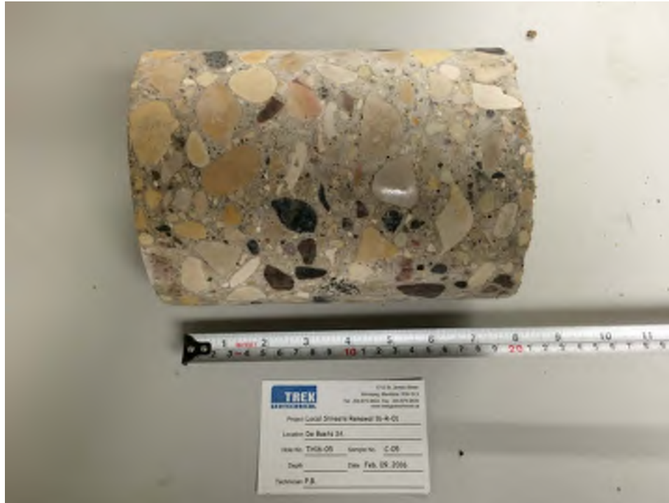
Photo 5: Pavement Core Sample at Test Hole TH16-05
