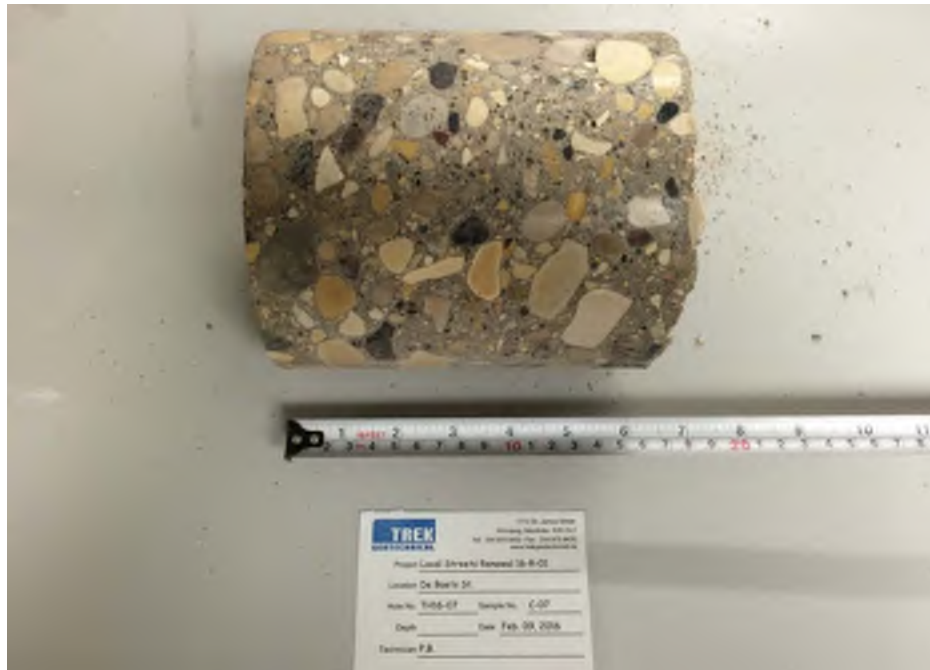
Photo 7: Pavement Core Sample at Test Hole TH16-07
