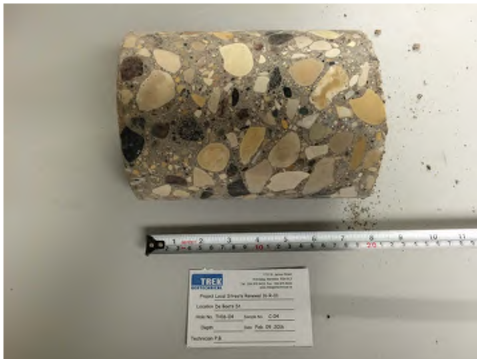
Photo 4: Pavement Core Sample at Test Hole TH16-04
