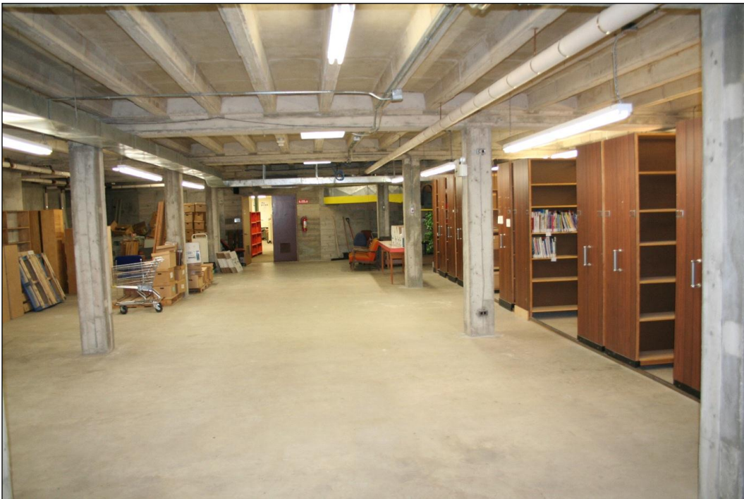
Plate 12 – St. Vital Library, 6 Fermor Avenue, basement, west end storage area, 2013. (M. Peterson, 2013.)
