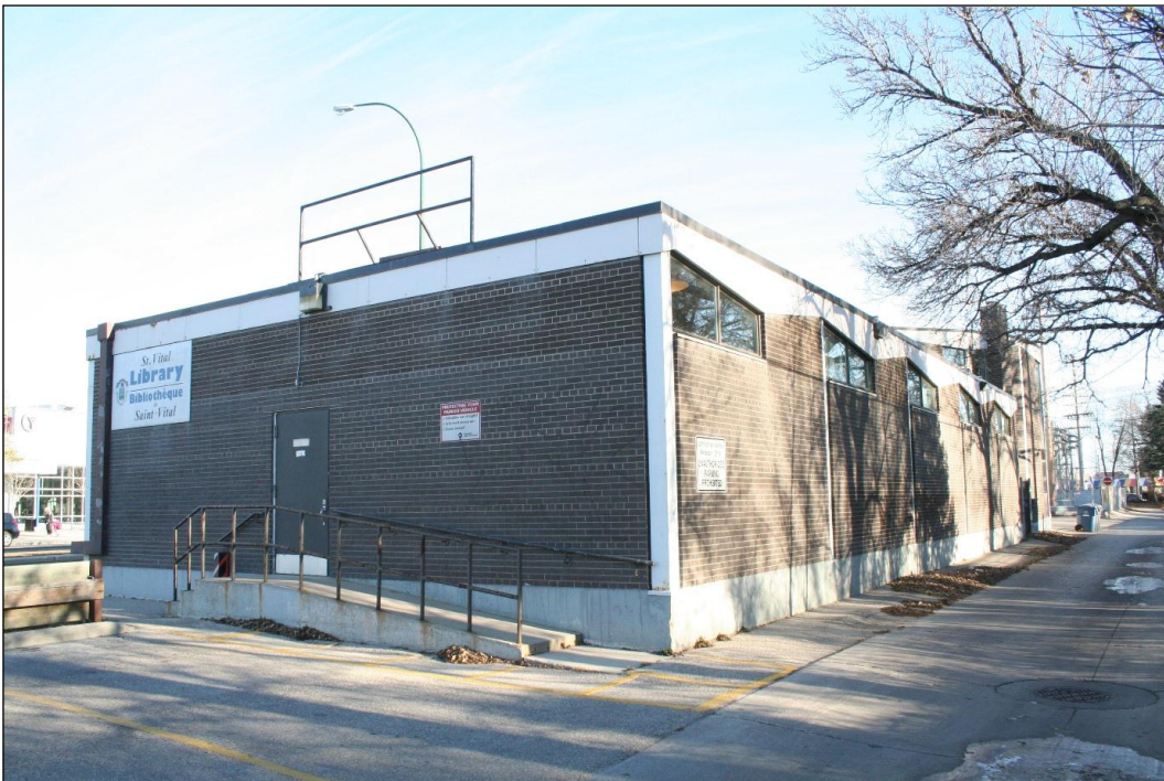
Plate 4 – St. Vital Library, 6 Fermor Avenue, west and south façade, 2013. ( M. Peterson, 2013. )
