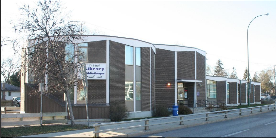
Plate 5 – St. Vital Library, 6 Fermor Avenue, front (north) façade, 2013. ( M. Peterson, 2013. )
