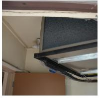
Overhead air-condition unit reduces headroom clearance
