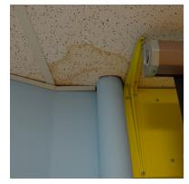
Water staining on acoustic ceiling
