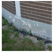
Paint finish peeling off concrete foundation
