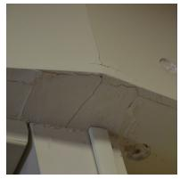
Damage to GWB bulkhead and un-patched plugs
