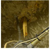
Ceiling penetration infilled with wood
