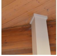
Roof decking separated from beam
