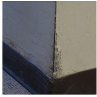
Damage to GWB at base of wall
