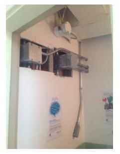
Figure 1: Junction Boxes & Extensions on Rear of Panelboards A & B
