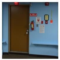
Step up and non-compliant door release hardware on door
