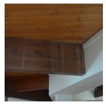
Water staining on roof structure
