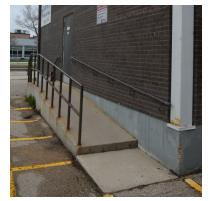
Concrete base at ramp fallen away
