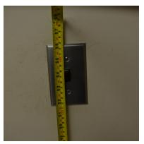
Light switch positioned too high, outside of barrier free acceptable range
