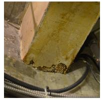
Damage on underside of GWB
