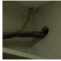
Penetrations into adjacent boiler room required to fire stopped
