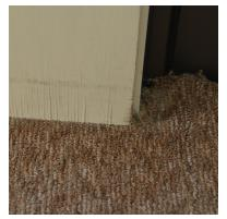
Damage at base of column due to water
