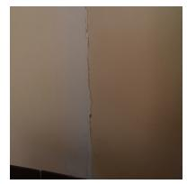
Cracking in GWB along exterior wall
