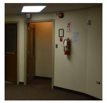
Non-fire rated door into stairwell at basement level
