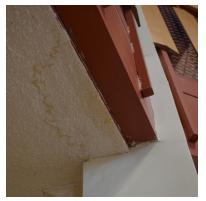
Water staining at underside of mezzanine structure
