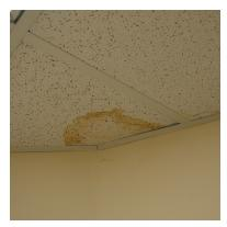
Water staining on acoustic ceiling
