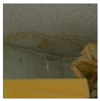
Water staining on acoustic ceiling
