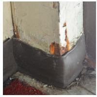
Damage at base of wall adjacent to exterior door
