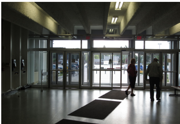
Above: Vestibule with automatic sliding door system and door operator
