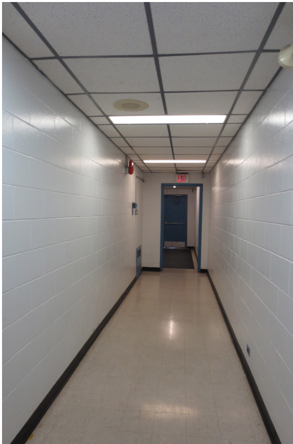
Corridor E19 leading to the east exit
