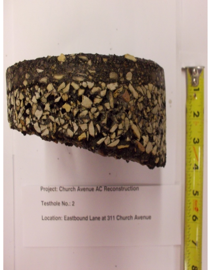
Photo 2: C02: Eastbound lane at 311 Church Avenue, 1.0 m from curb
