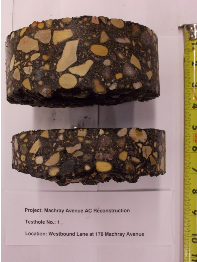
Photo 1: TH01: Westbound lane at 178 Machray Avenue, 1.0 m from curb
