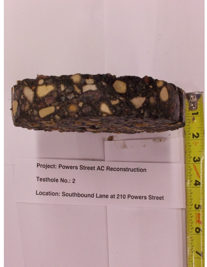
Photo 2: TH02: Southbound lane at 210 Powers Street, 1.5 m from curb
