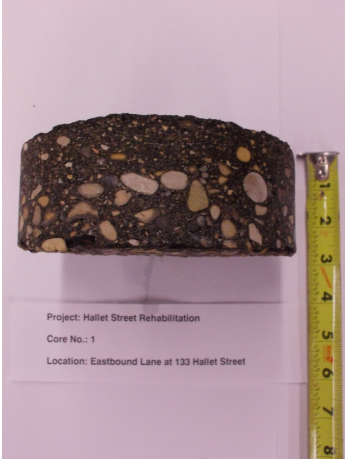
Photo 1: C01: Eastbound lane at 133 Hallet Street, 0.9 m from curb
