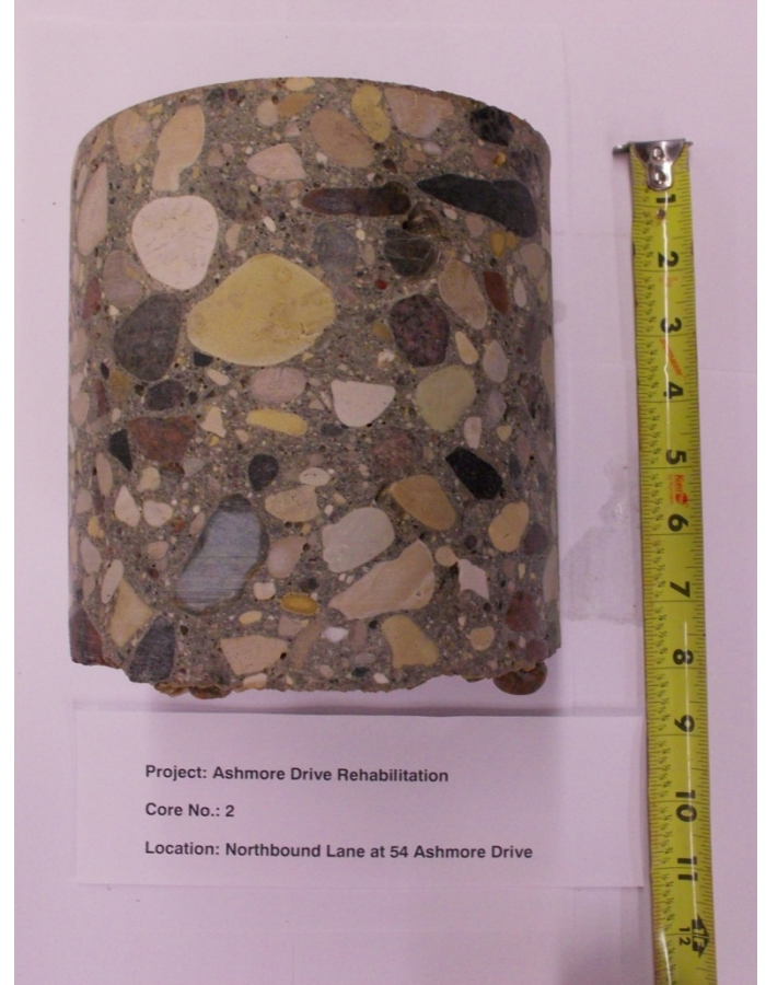
Photo 2: C02: Northbound lane at 54 Ashmore Drive, 1.0 m from curb
