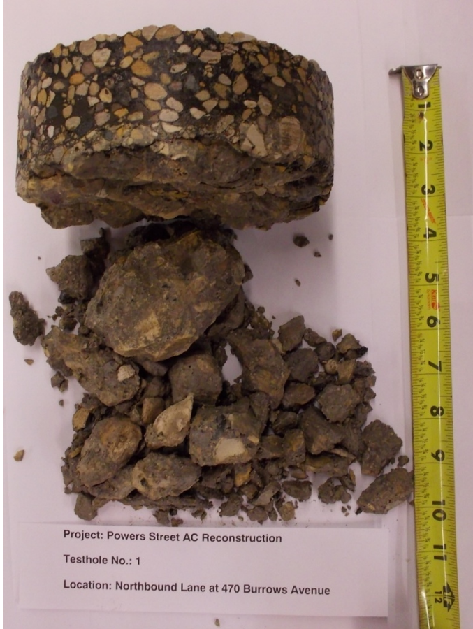
Photo 1: TH01: Northbound lane at 470 Burrows Avenue, 1.0 m from curb
