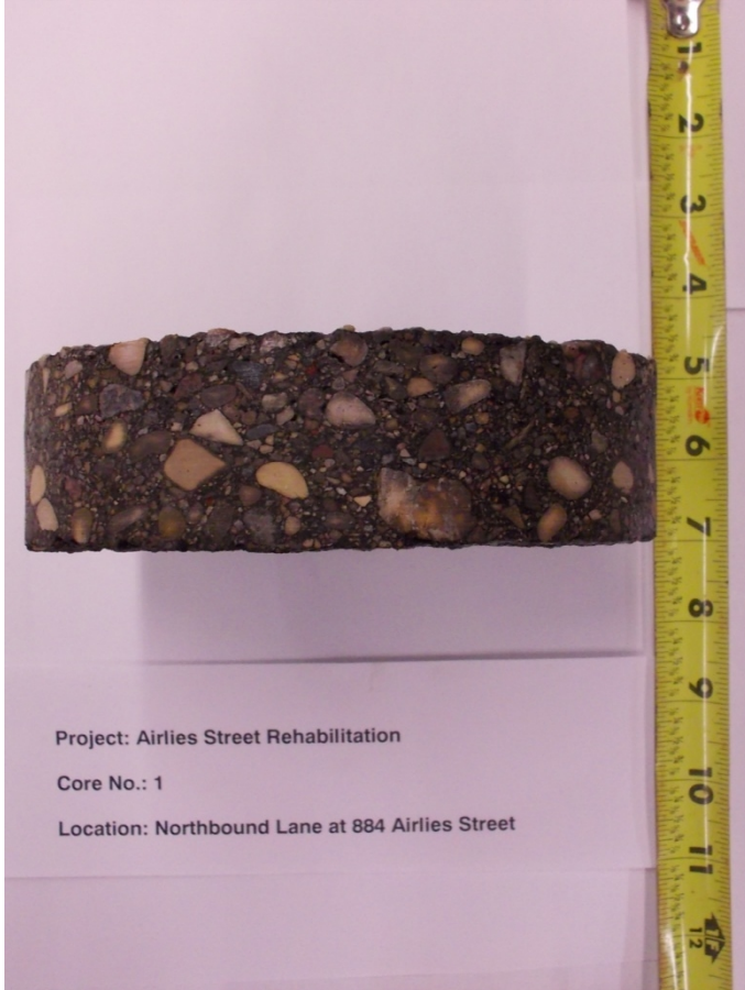
Photo 1: C01: Northbound lane at 884 Airlies Street, 1.0 m from curb
