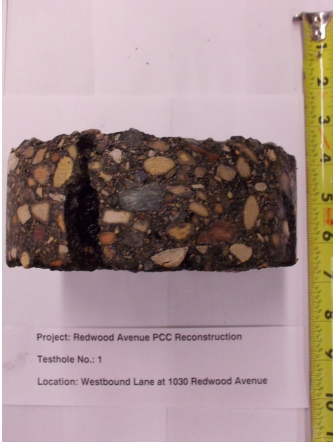
Photo 1: TH01: Westbound lane at 1030 Redwood Avenue, 1.0 m from curb
