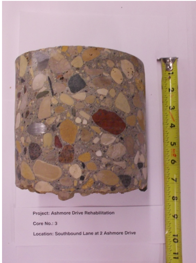
Photo 3: C03: Southbound lane at 2 Ashmore Drive, 1.5 m from curb
