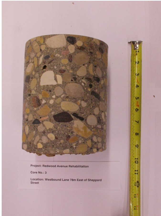
Photo 3: C03: Westbound lane 78 m east of Sheppard Street, 1.8 m from curb
