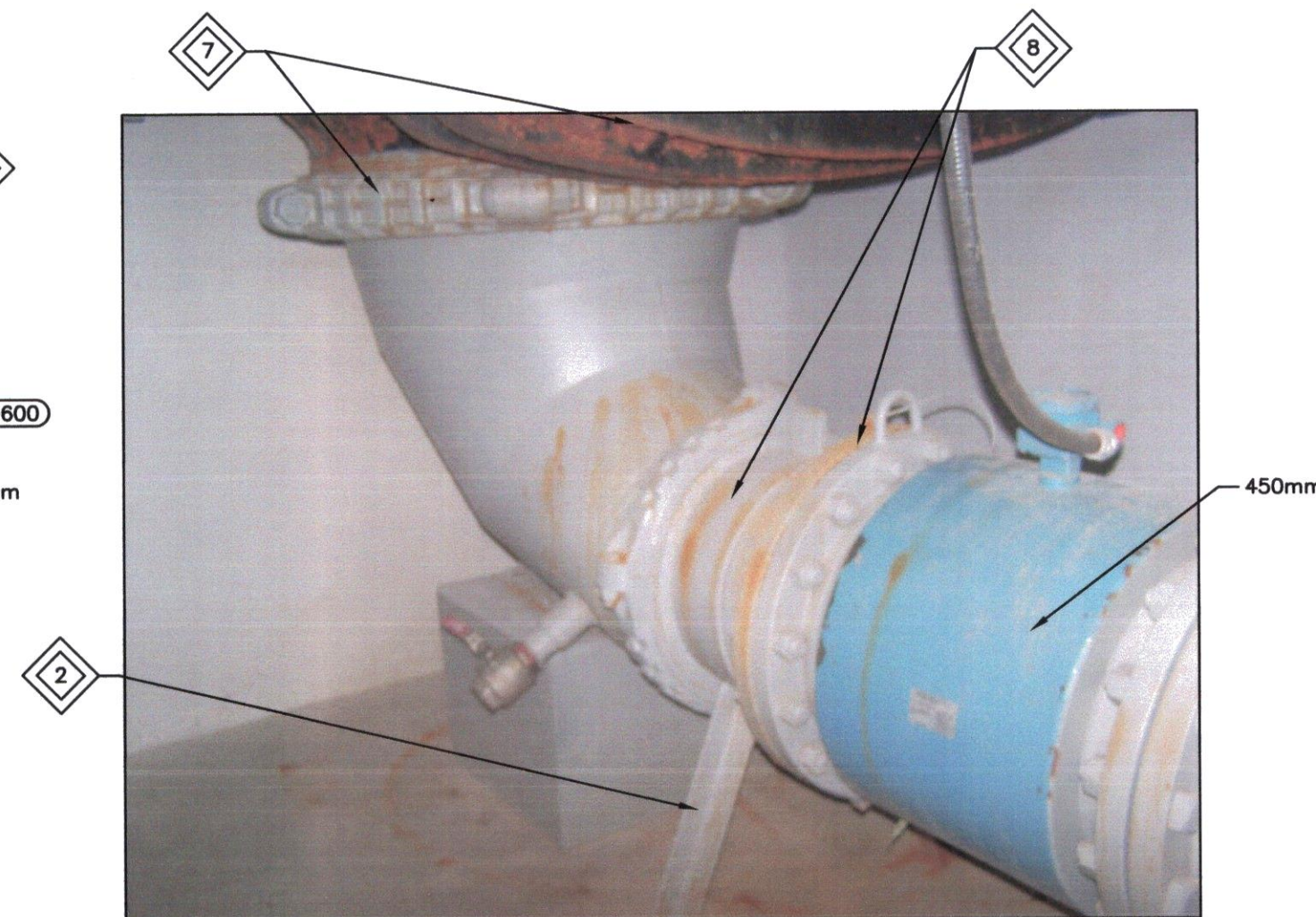
5 SHUTDOWN 6 - DEMOLITION VALVE FM-03 M2
