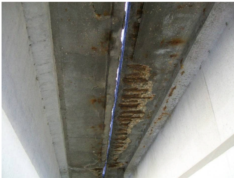
NORTHBOUND BRIDGE EAST SOFFIT
