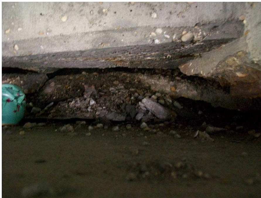
CONDITION OF THE SOUTH ABUTMENT SEAT
