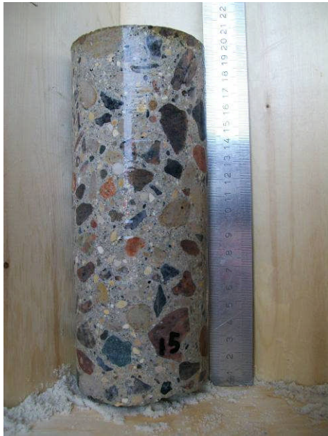
SPAN 1 Core No. 15
