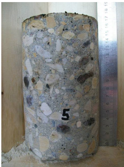
SPAN 3 Core No. 5
