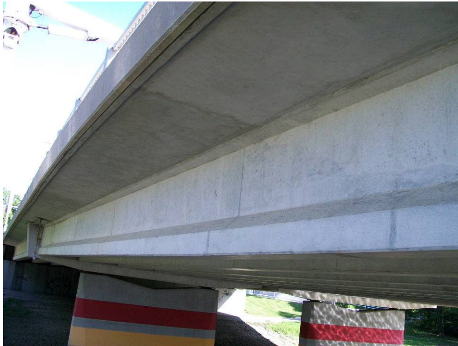
SOUTHBOUND BRIDGE WEST SOFFIT
