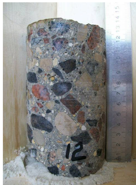
SPAN 4 Core No. 12
