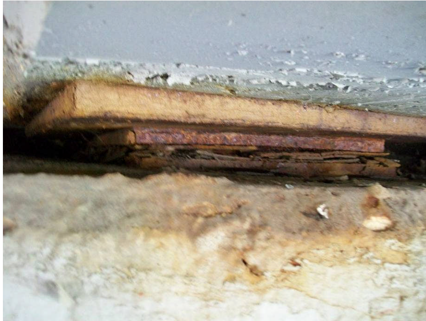
CONDITION OF THE BRIDGE BEARING ON THE NORTH ABUTMENT
