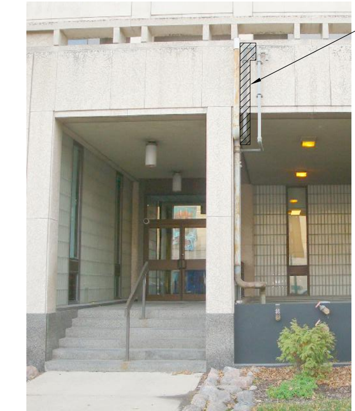
NOTE: PHOTO TAKEN OUTDOORS AT STREET LEVEL. PHOTO SCALE: NTS EXTERIOR RELIEF VENT
