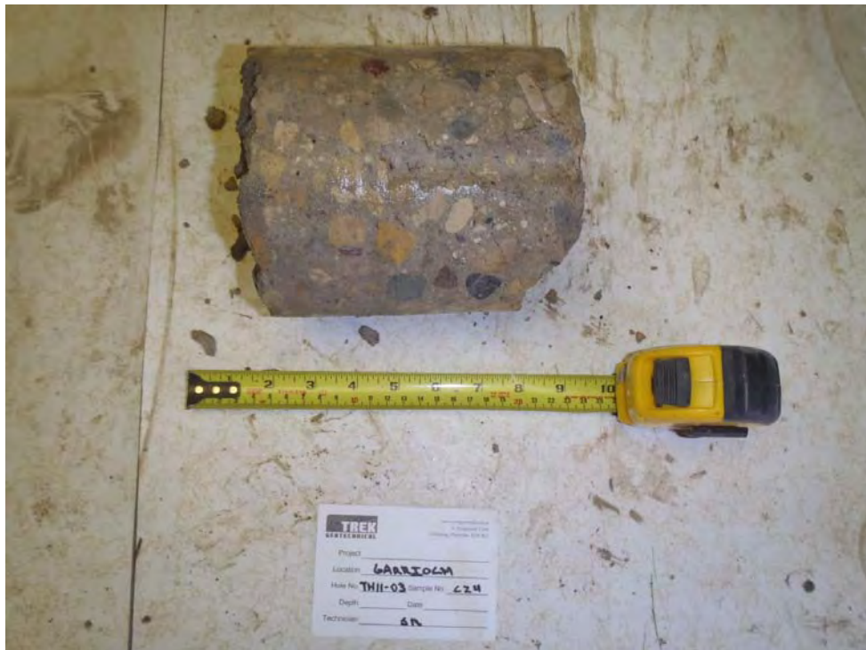
Photo 6: Concrete core sample from TH11-03
