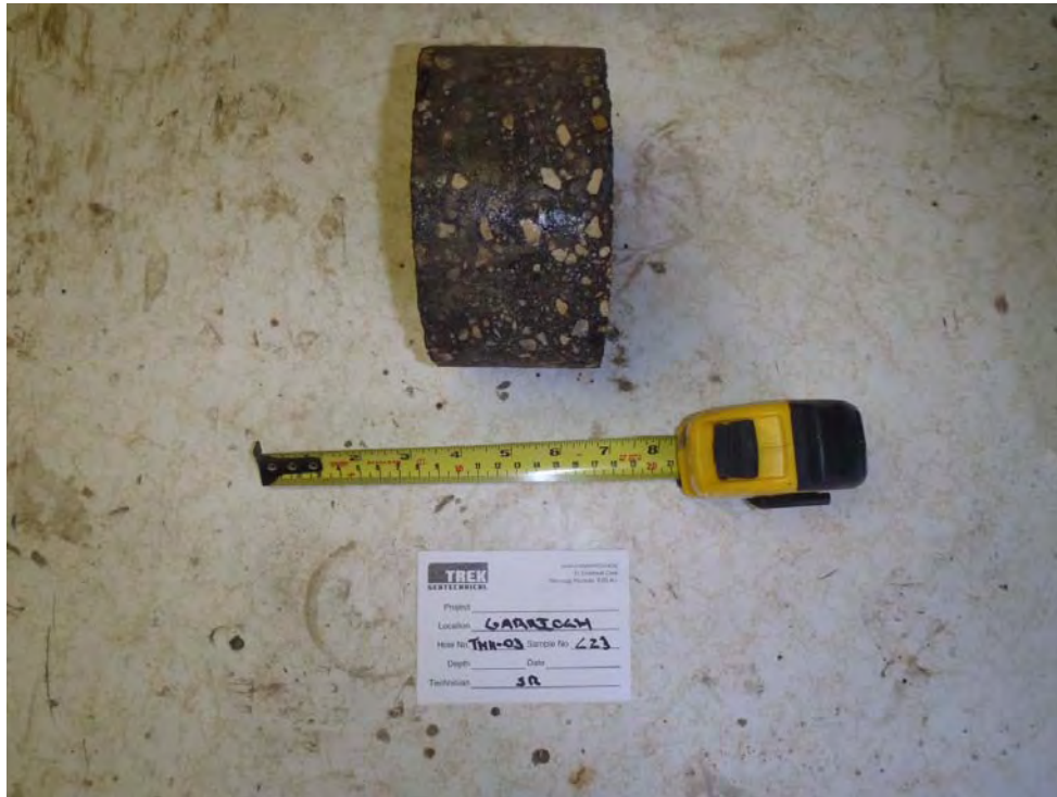
Photo 5: Asphalt core sample from TH11-03
