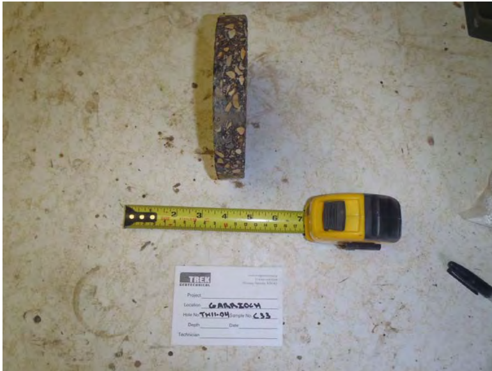
Photo 7: Asphalt core sample from TH11-04
