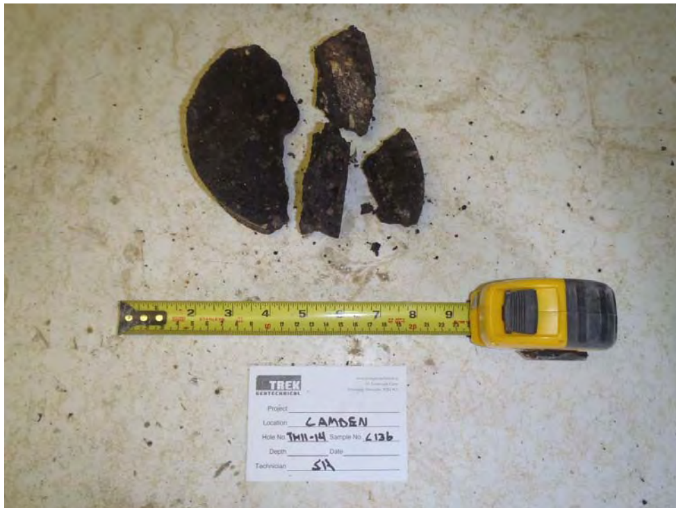
Photo 24: Asphalt core sample from TH11-14
