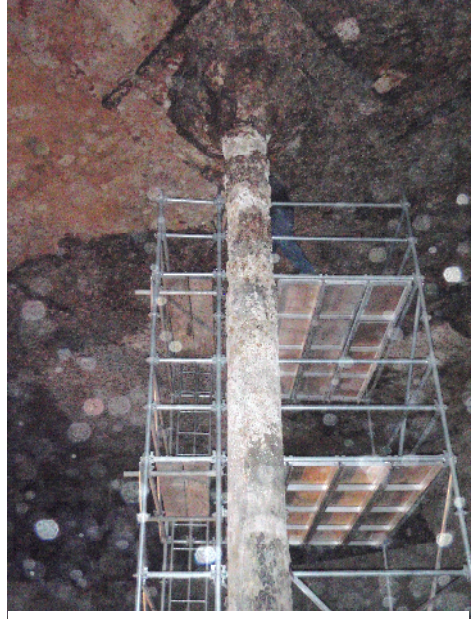
Column with Several Scraped Rings for Circumference Measurements
