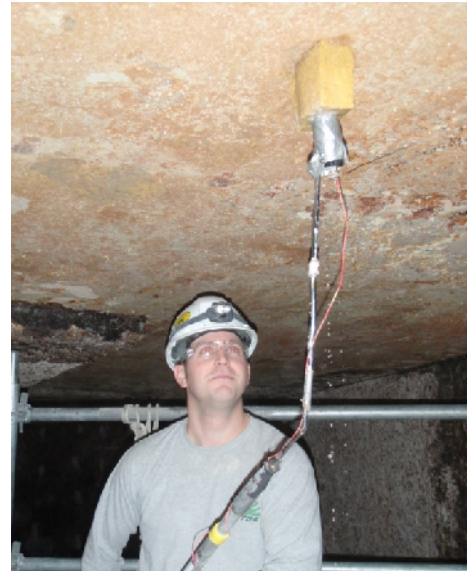
Half-Cell Measurements on Ceiling
