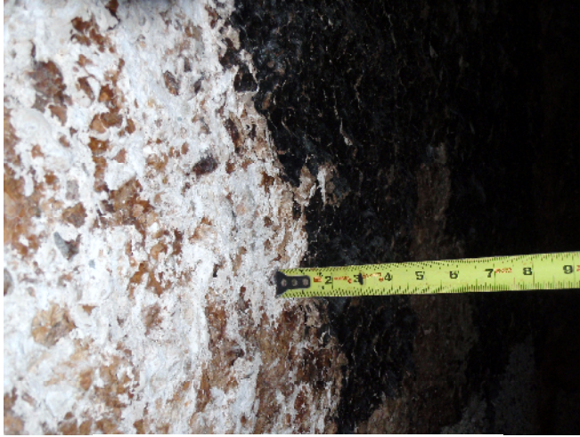
Scraped and Unscraped Level 5
