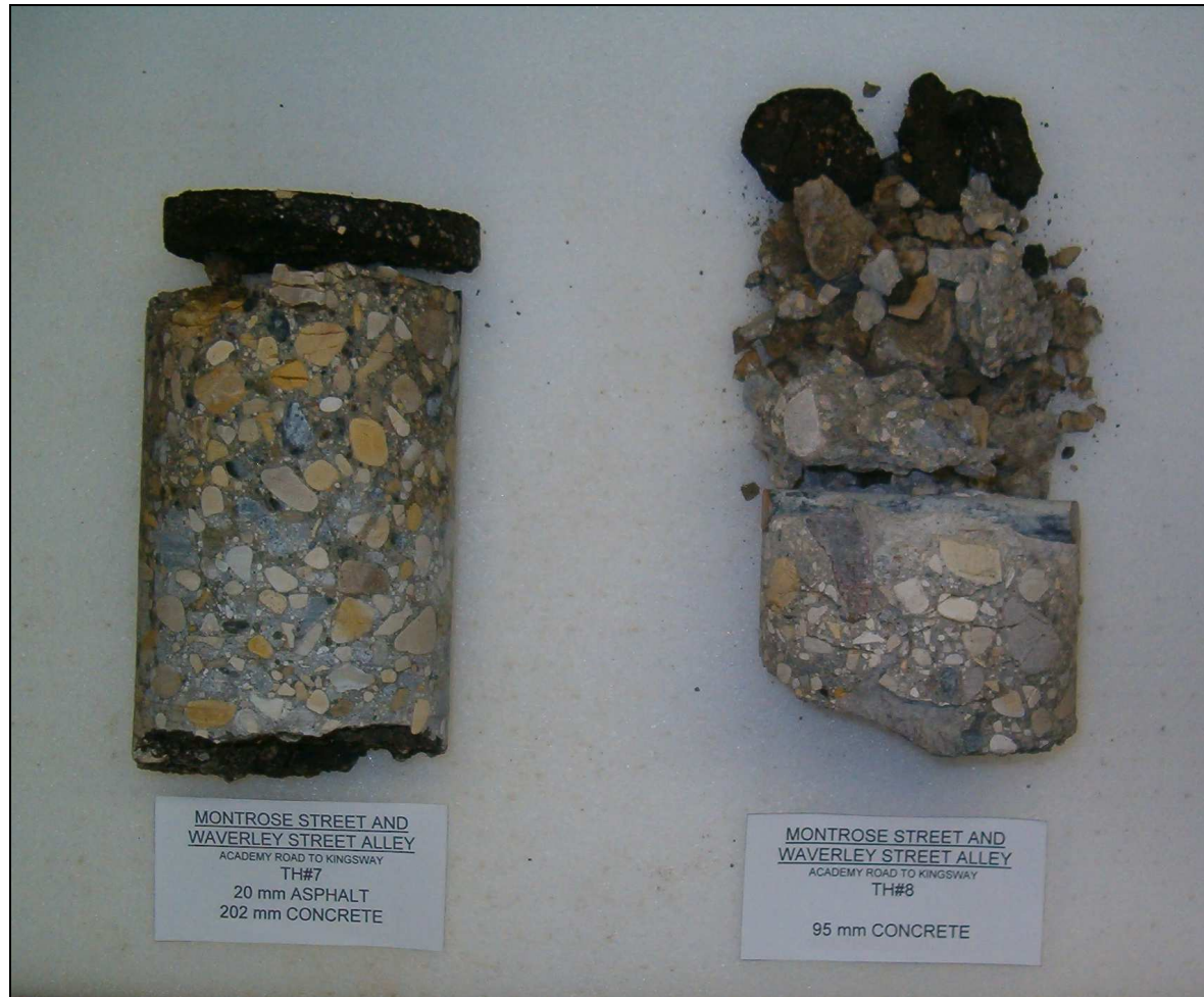
Montrose Street and Waverley Street Alley Academy Road to Kingsway
