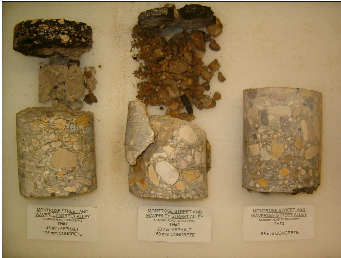
Montrose Street and Waverley Street Alley Academy Road to Kingsway
