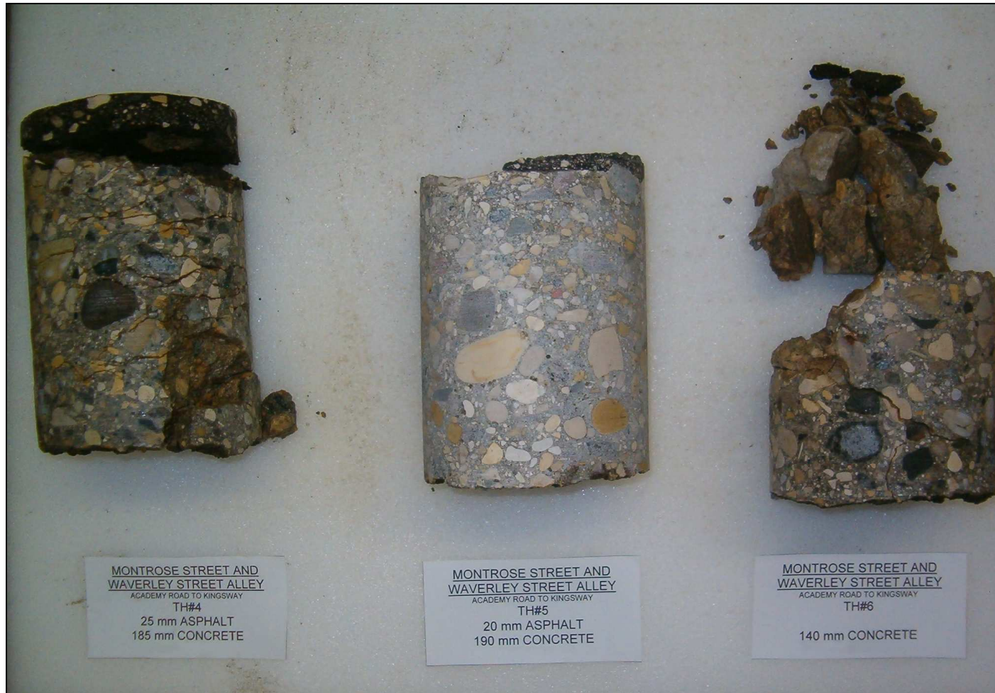
Montrose Street and Waverley Street Alley Academy Road to Kingsway
