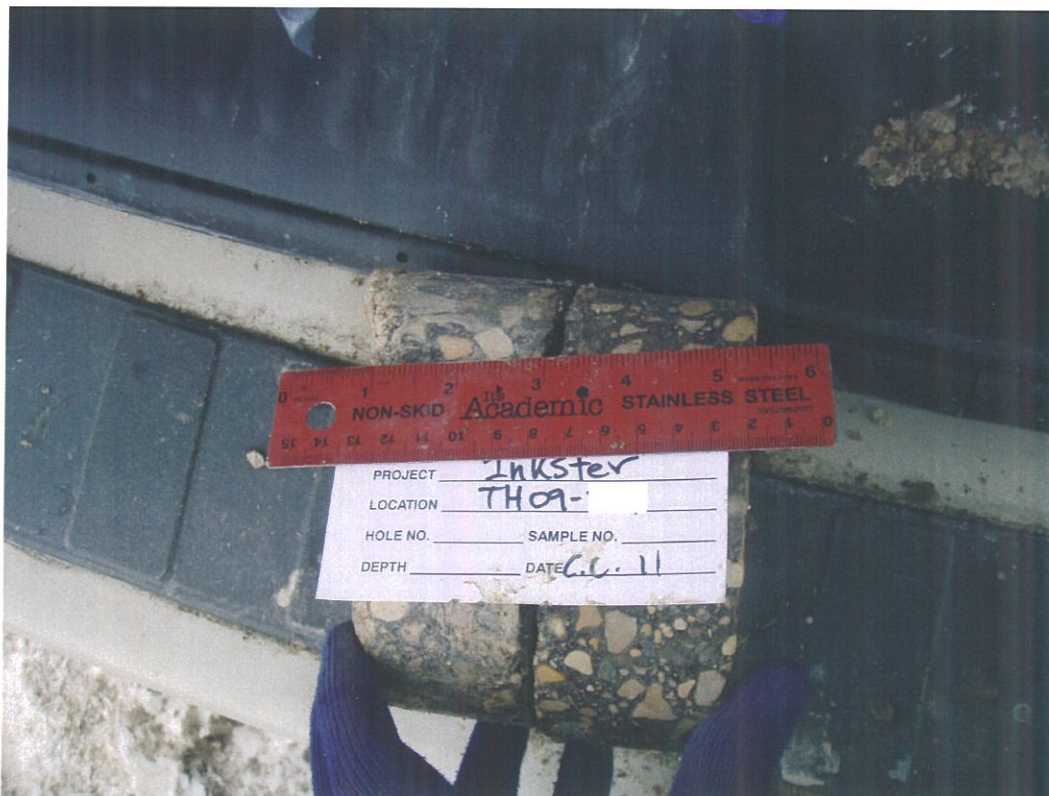
Photo 26: Core sample from TH-09-38 (incorrectly labeled in photo)
