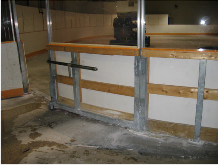
VA9: Back View of Double Leaf Equipment Gate Framework
