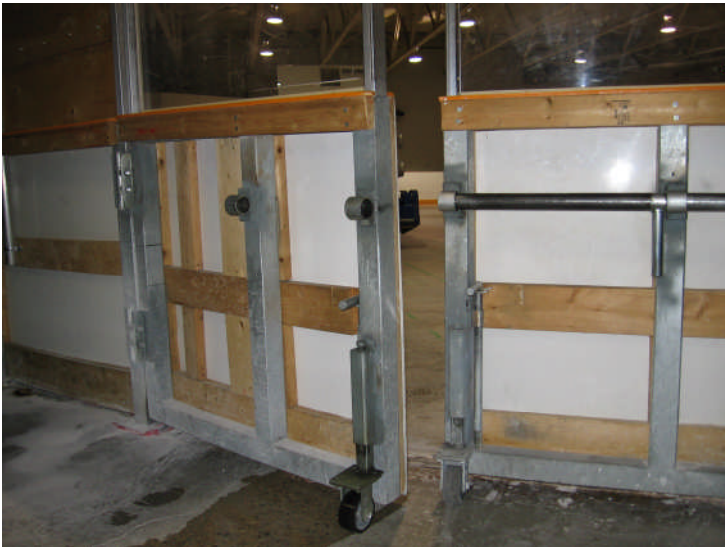
VA11: Back View of Double Leaf Equipment Gate Casters
