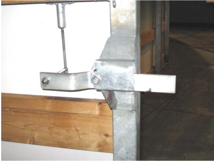
VA 5: Player's Gate Latch Detail
