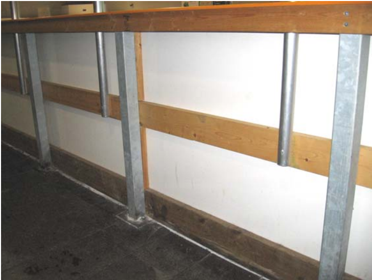
VA 3: Back View of Rink Board Wood Framework
