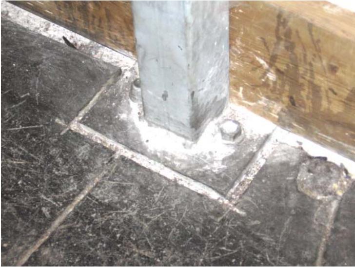
VA 1: Top View of Rink Board Steel Posts/Base Plates
