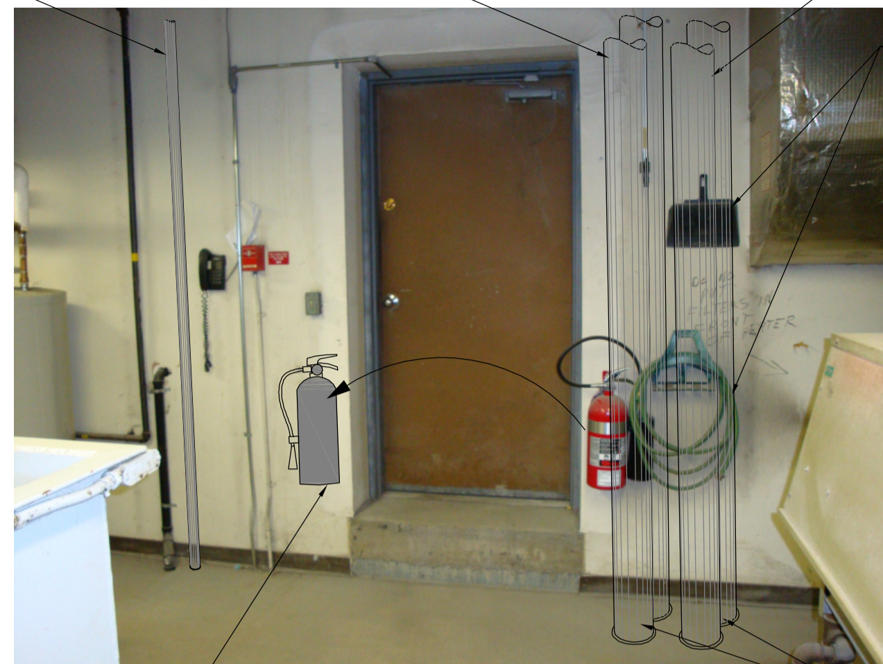
RELOCATE EXISTING FIRE EXTINGUISHER AND MOUNTING BRACKET
