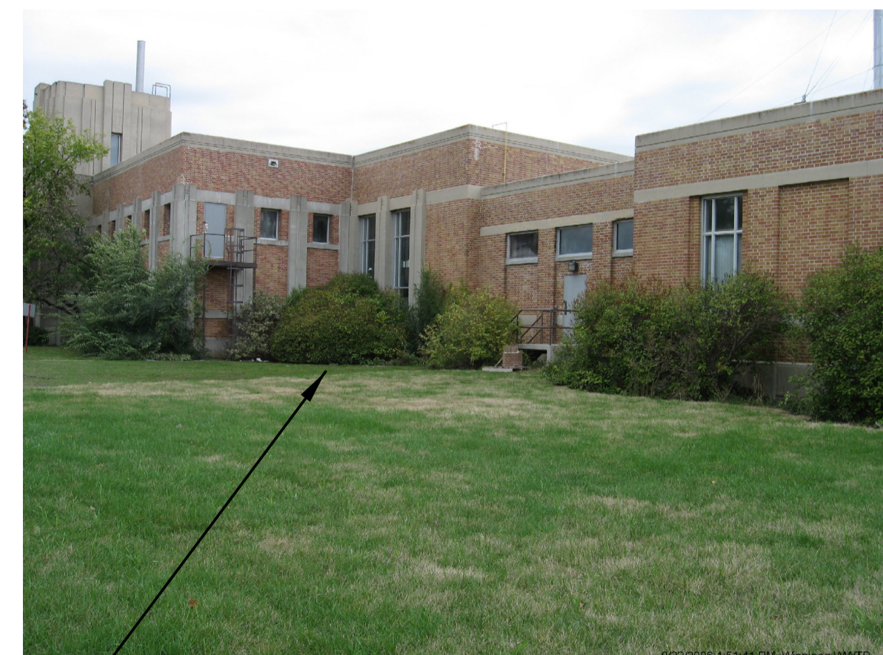
EXISTING SITE AND SHRUB DEMOLITION REQUIRED
