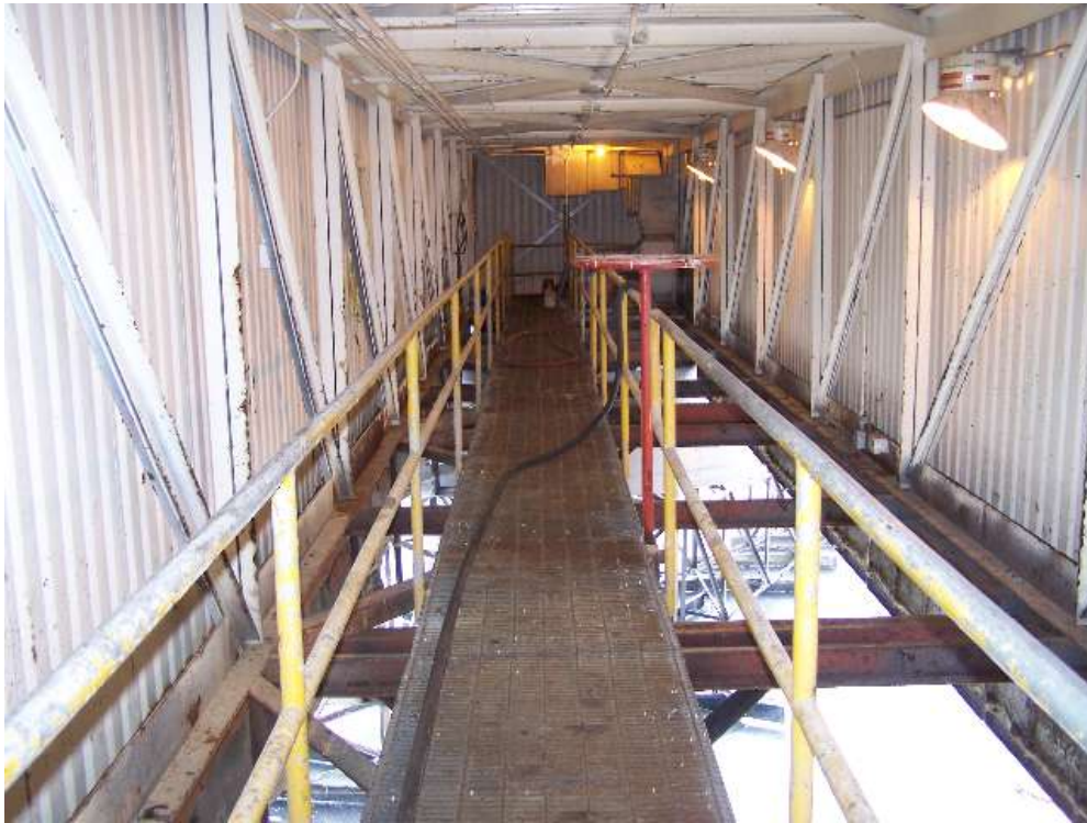
Photo 3-14 Clarifier Walkway & Enclosure
