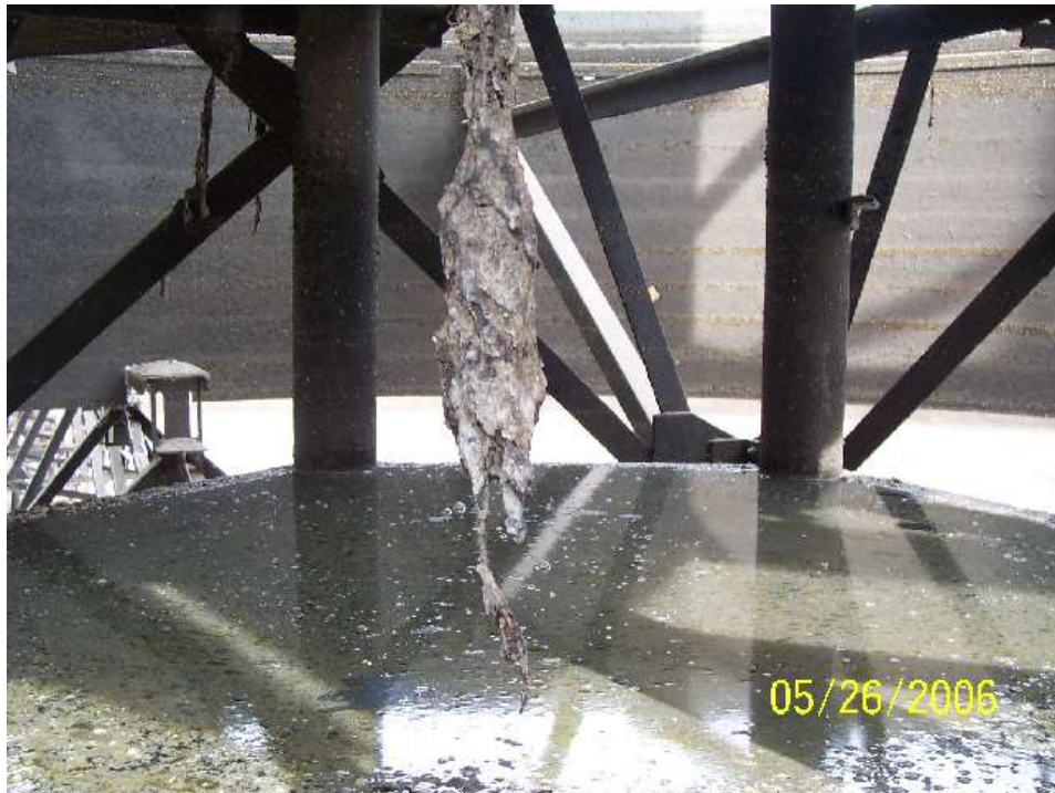
Photo 3-2 Top of Concrete Clarifier Influent Pipe/Base
