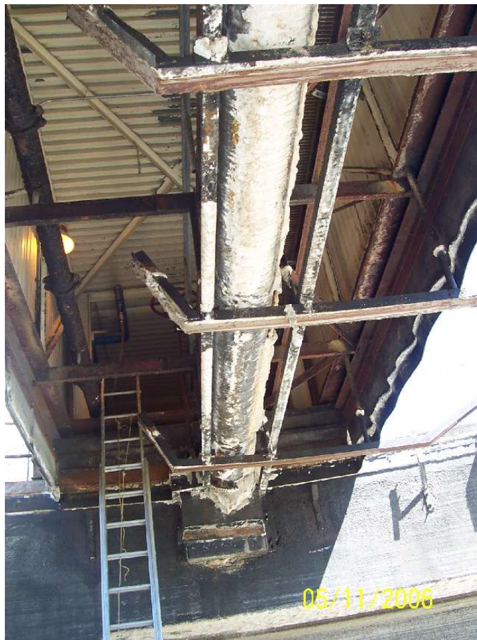
Photo 1-2 Scum Trough & Discharge Box
