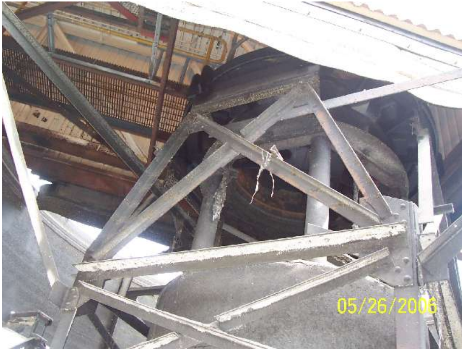
Photo 3-1 Concrete Clarifier Influent Pipe/Base
