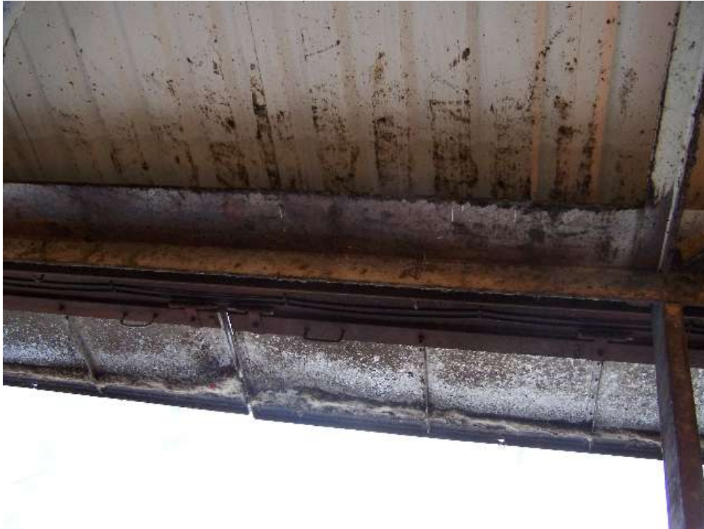
Photo 3-15 Enclosure Hinged Scum Blade Access Panels
