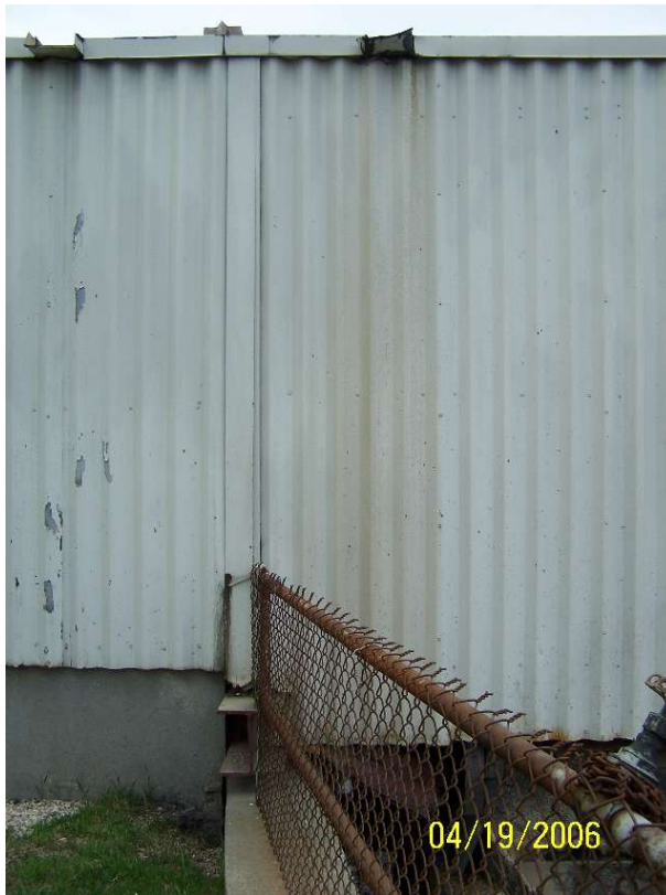
Photo 2-4 Clarifier Walkway Enclosure Connection
