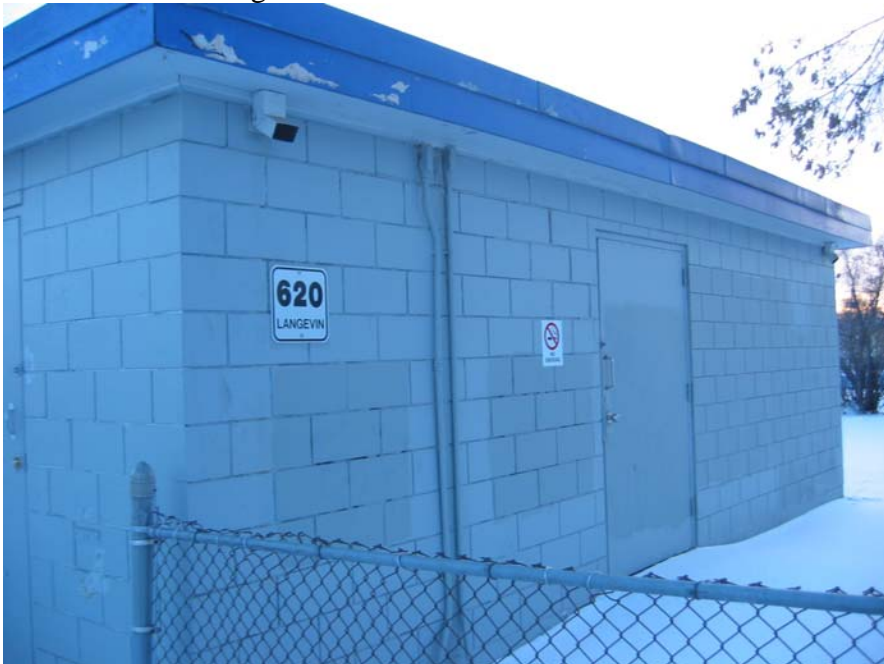
West side of building – view from NE corner looking south.
