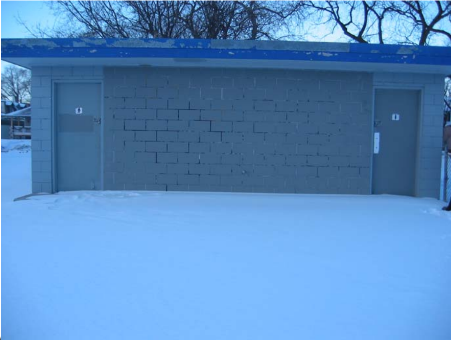
East side of building
