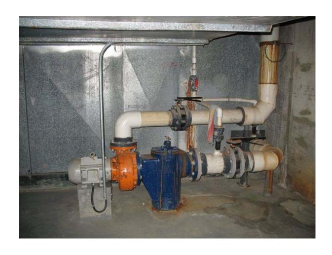
EKW- PHOTO 12: EXISTING PUMP AND FILTER. NOTE: EQUIPMENT TO BE REPLACED UNDER THIS CONTRACT.
