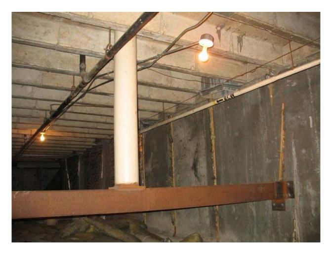
EKW- PHOTO 15: STRUCTURAL STEEL SUPPORT FOR EXISTING MAST SPANNING TUNNEL AREA OF BASEMENT BELOW THE EXISTING WATERSLIDE.NOTE: MAST TO BE REMOVED, STRUCTURAL SUPPORT MAY BE RETAINED IF SUITABLE.
