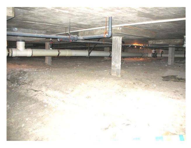
EKW- PHOTO 13: EXISTING MAKE UP WATER FROM UNDERSIDE OF POOL. NOTE: EXISTING SCH 40 PVC PIPING TO BE REPLACED WITH NEW SCH 80 PVC PIPING UNDER THIS CONTRACT.
