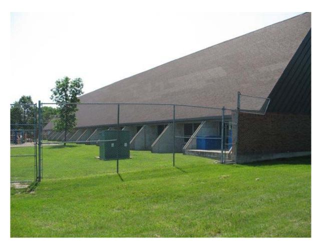
EKW- PHOTO 4: ELMWOOD KILDONAN POOL, NORTH WALL FACING THE PLAYGOUND AREA. NOTE: THE CONCRETE BUTTRESSES ARE IN LINE WITH THE INTERIOR WOOD BEAM FRAMING.
