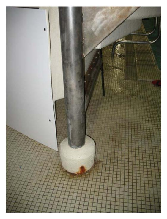
EKW-PHOTO 10: SUPPORT MAST FOR EXISTING SPIRAL STAIR TO BE DEMOLISHED AND REMOVED UNDER THIS CONTRACT. POOL DECK FINISHES TO BE RESTORED.
