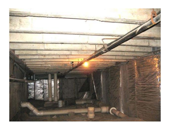
EKW- PHOTO 14: EXISTING RETURN WATER FROM SLIDE CONNECTING TO MAKE UP WATER FROM POOL RUNS TO PUMP INLET. NOTE: EXISTING SCH 40 PVC PIPING TO BE REPLACED WITH NEW SCH 80 PVC PIPING UNDER THIS CONTRACT.
