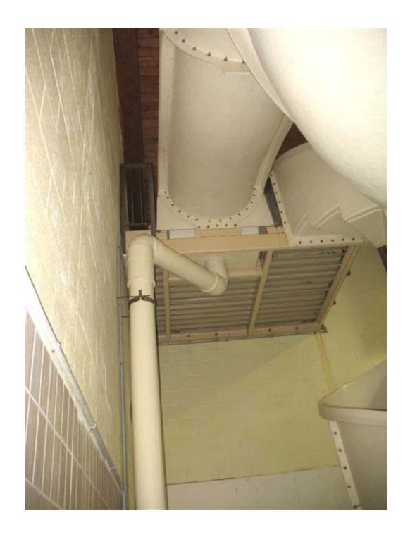
EKW- PHOTO 8: VIEW FROM UNDERSIDE OF THE EXISTING ACCESS PLATFORM. THIS PLATFORM IS TO BE DEMOLISHED AND REMOVED UNDER THIS CONTRACT. NOTE THE PRESENT LOCATION FOR THE WATER SUPPLY PIPING.
