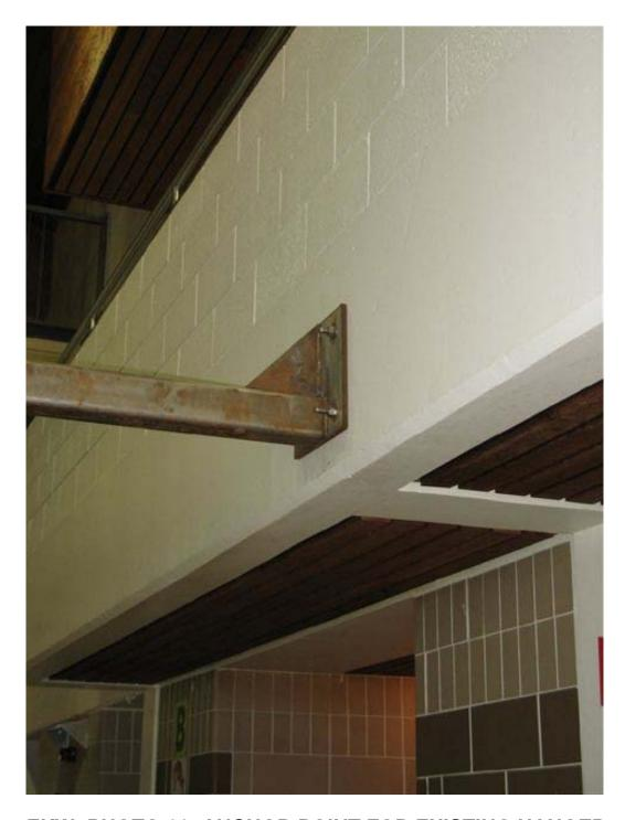
EKW- PHOTO 11: ANCHOR POINT FOR EXISTING HANGER SUPPORTING SECTION OF WATERSLIDE. THE HANGER IS TO BE REMOVED UNDER THIS CONTRACT AND THE WALL FINISH RESTORED.
