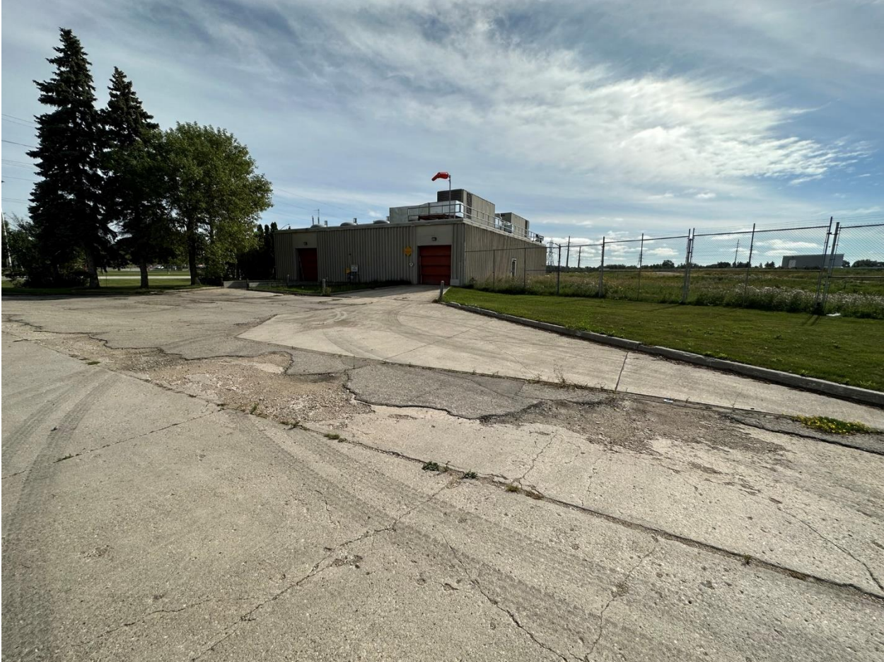
Figure 18: Site access, looking east.
