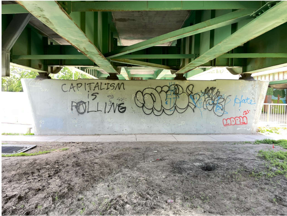
Photo 43 - Pier 8 NB, north face
