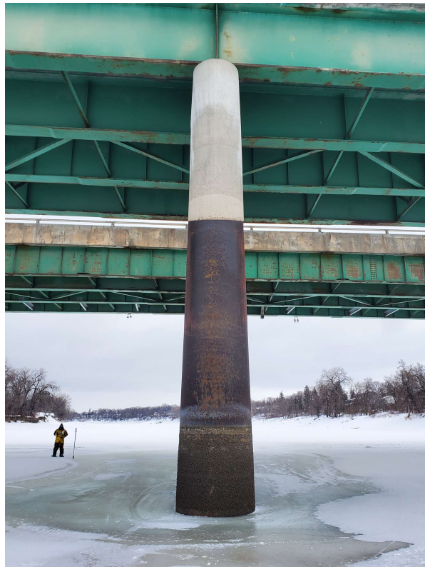
Photo 20 - Pier 5 West End 10 of 22
