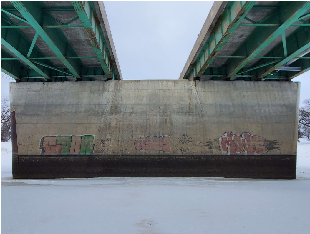
Photo 05 - Pier 4 South Face
