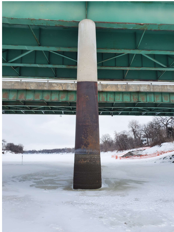
Photo 30 - Pier 6 West End 15 of 22
