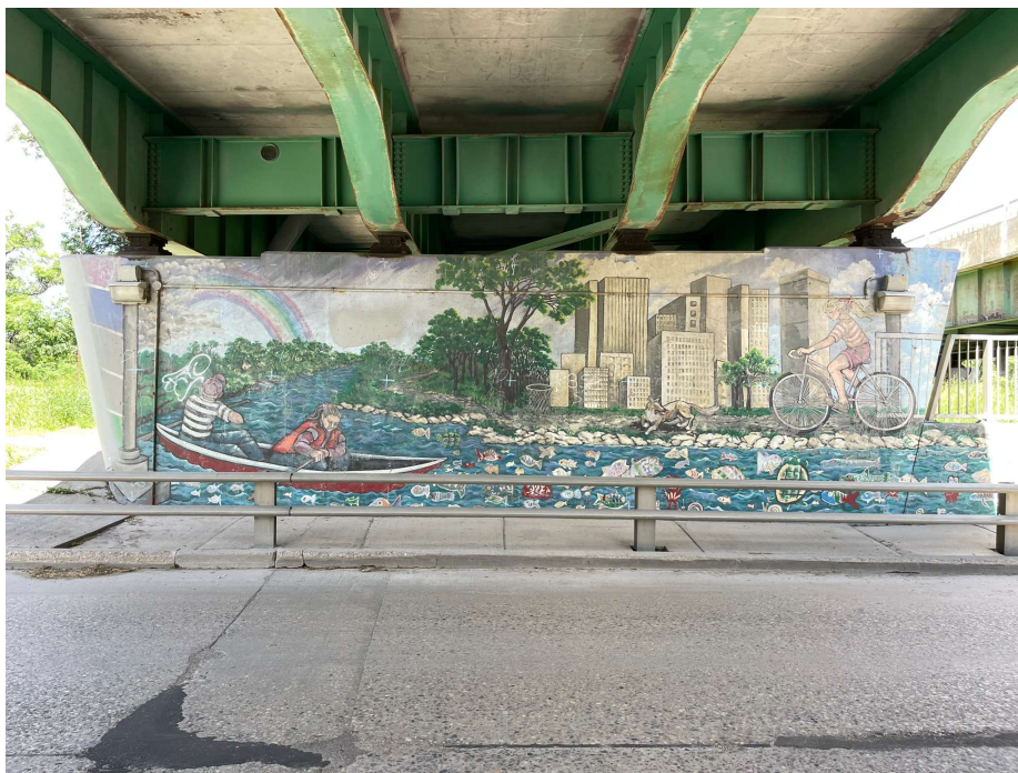
Photo 46 - Pier 8 SB, south face
