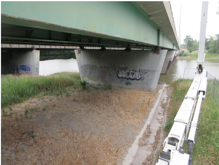
Photo 36 - Pier 3 SB North Face
