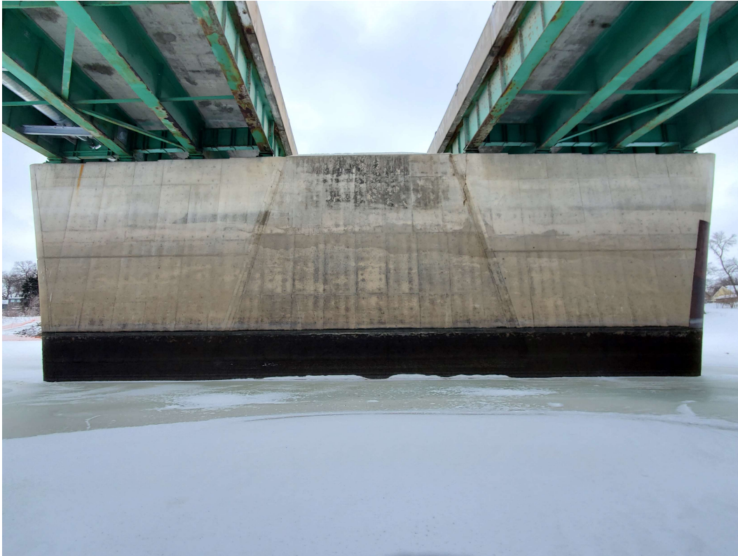
Photo 11 - Pier 5 North Face
