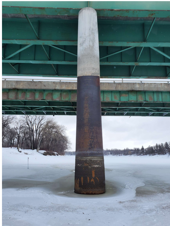
Photo 10 - Pier 4 West End 5 of 22
