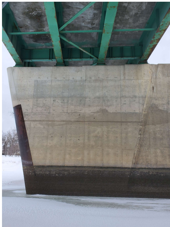
Photo 18 - Pier 5 South Face West Section 9 of 22
