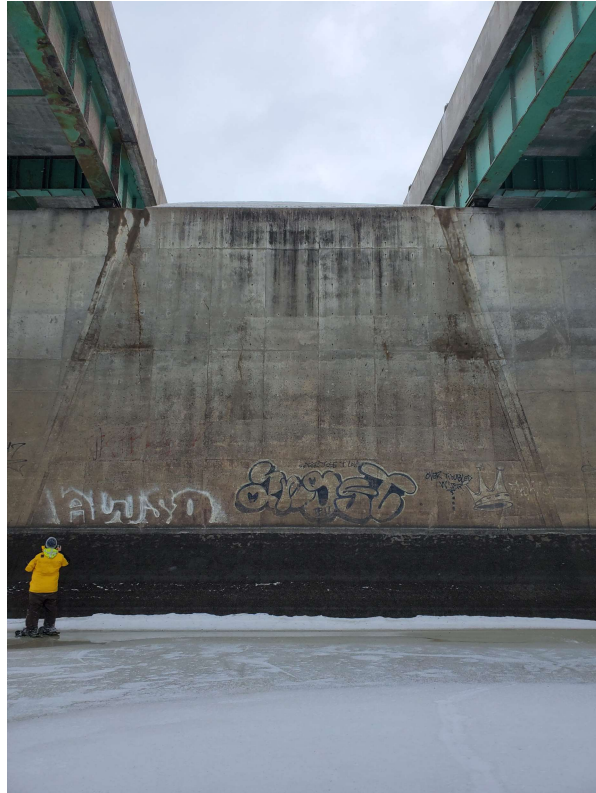
Photo 03 - Pier 4 North Face Middle Section
