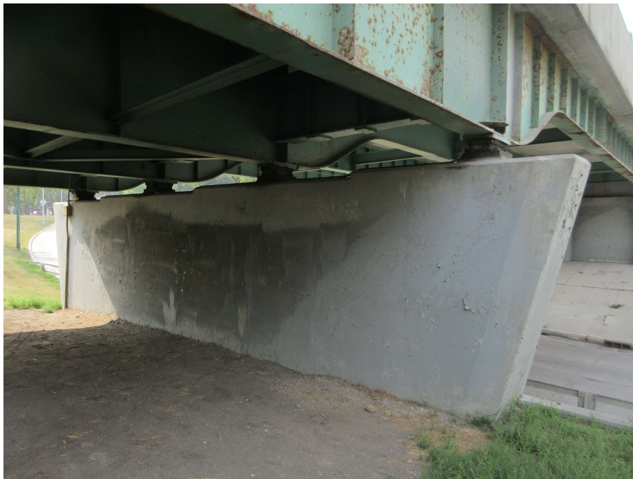
Photo 30 - Pier 1 SB South Face
