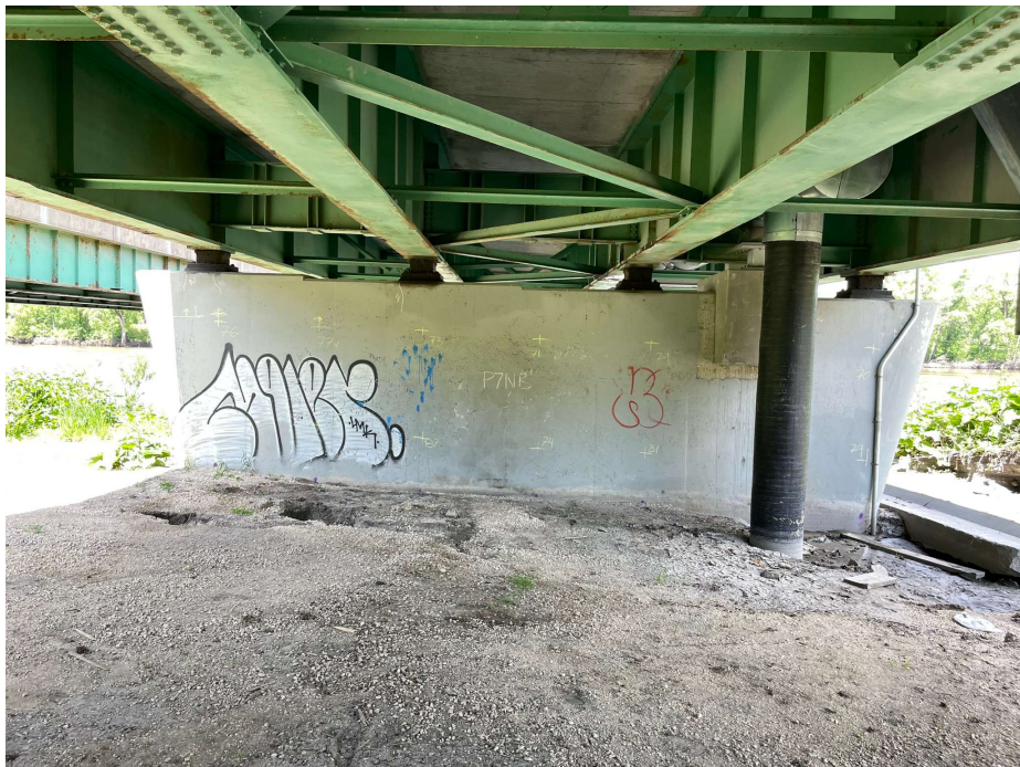
Photo 40 - Pier 7 NB, south face, note recent modification from forced main sewer
