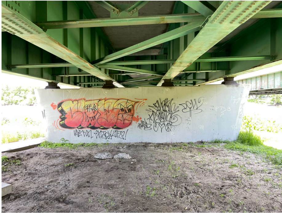
Photo 41 - Pier 7 SB, south face
