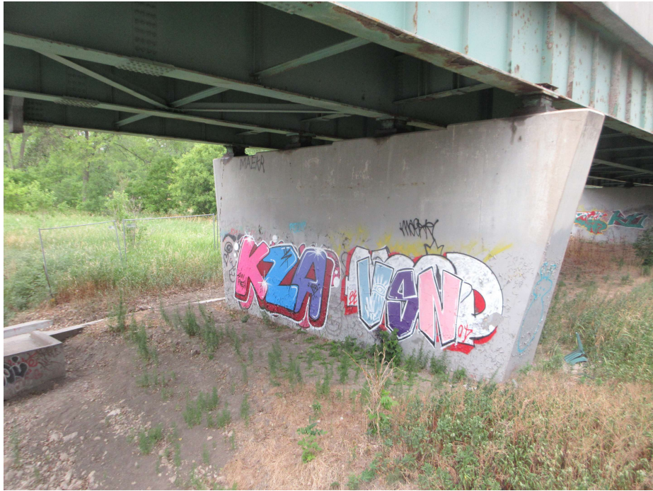
Photo 37 - Pier 3 SB South Face
