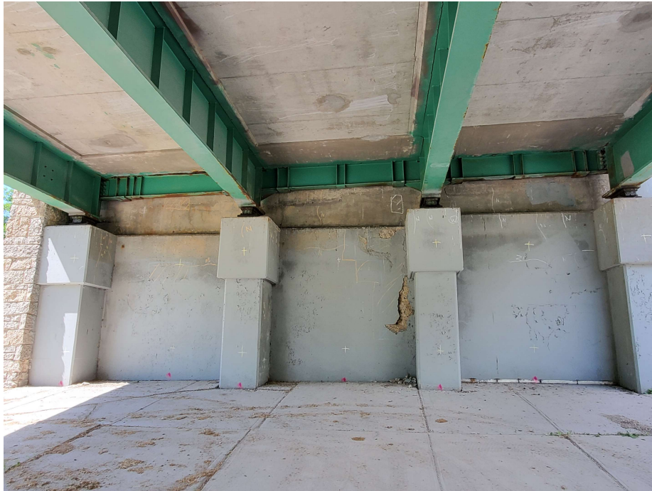
Photo 03 - North abutment SB Lanes
