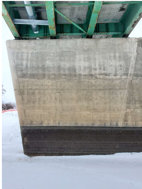
Photo 22 - Pier 6 North Face East Section 11 of 22
