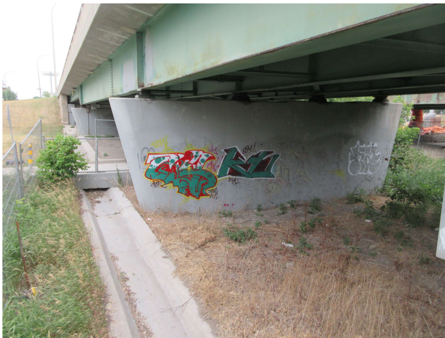
Photo 34 - Pier 2 SB South face
