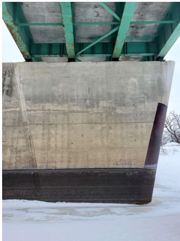
Photo 24 - Pier 6 North Face West Section 12 of 22
