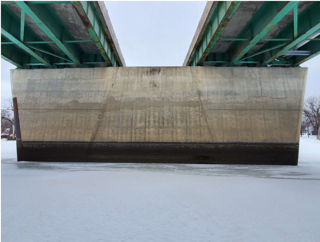
Photo 15 - Pier 5 South Face
