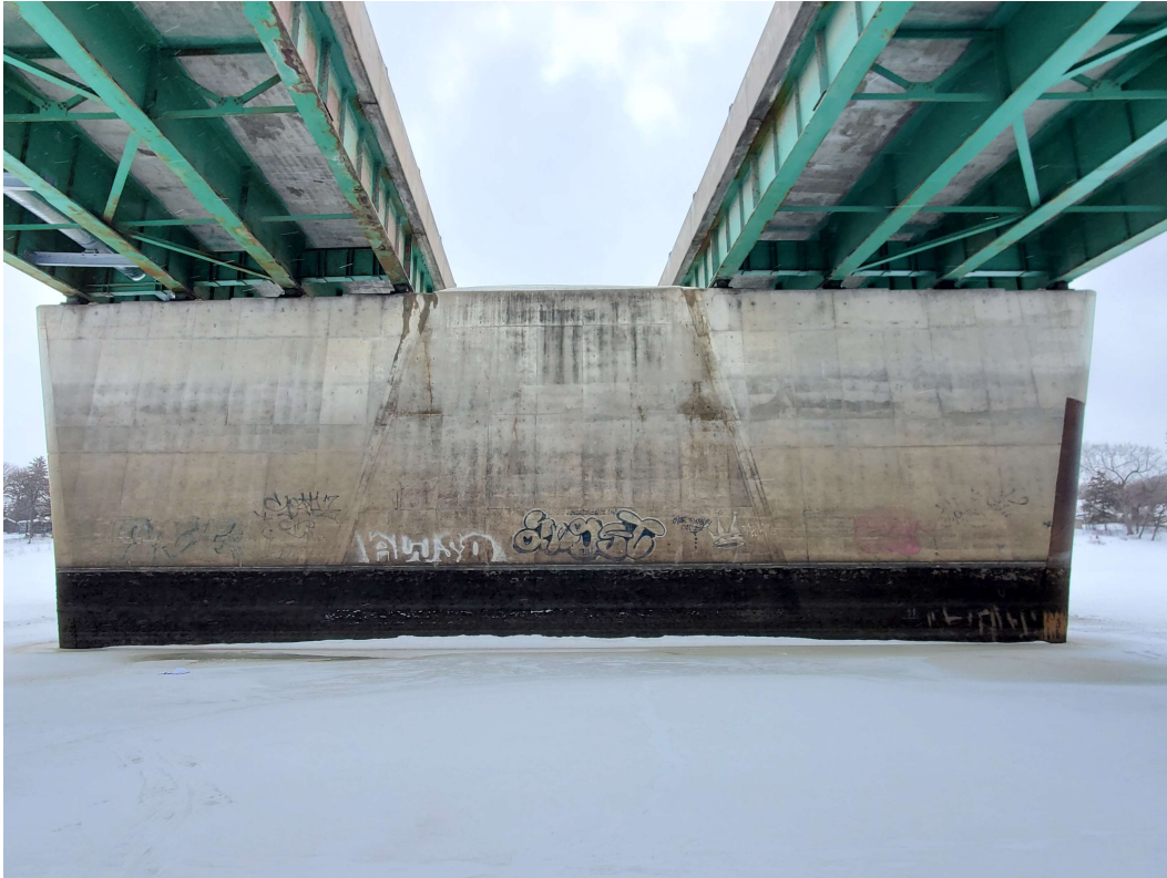
Photo 01 - Pier 4 North Face
