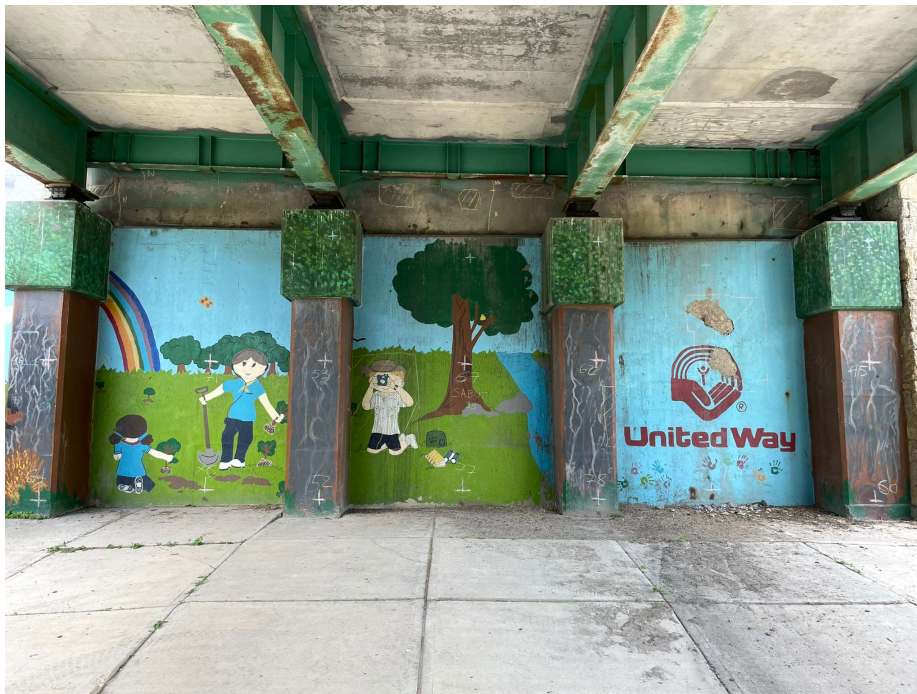
Photo 18 - South abutment wall, SB
