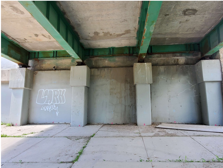
Photo 02 - North abutment NB Lanes
