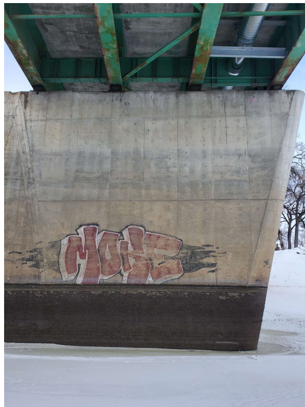
Photo 06 - Pier 4 South Face East Section 3 of 22
