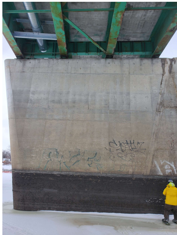
Photo 02 - Pier 4 North Face East Section 1 of 22
