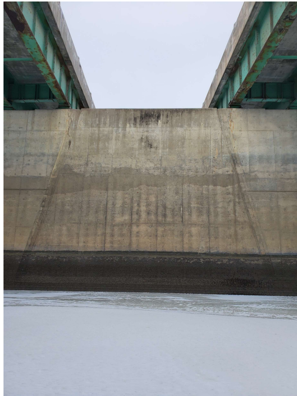
Photo 17 - Pier 5 South Face Middle Section
