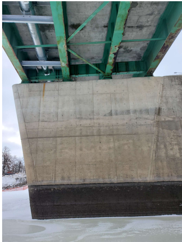
Photo 12 - Pier 5 North Face East Section 6 of 22
