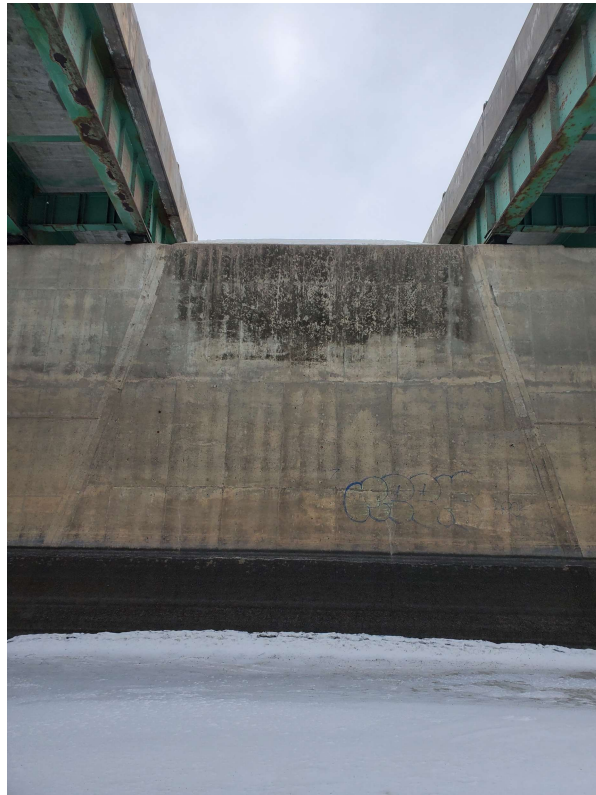
Photo 23 - Pier 6 North Face Middle Section
