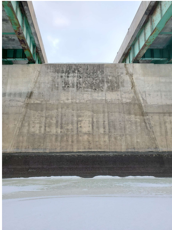
Photo 13 - Pier 5 North Face Middle Section
