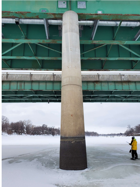
Photo 19 - Pier 5 East End
