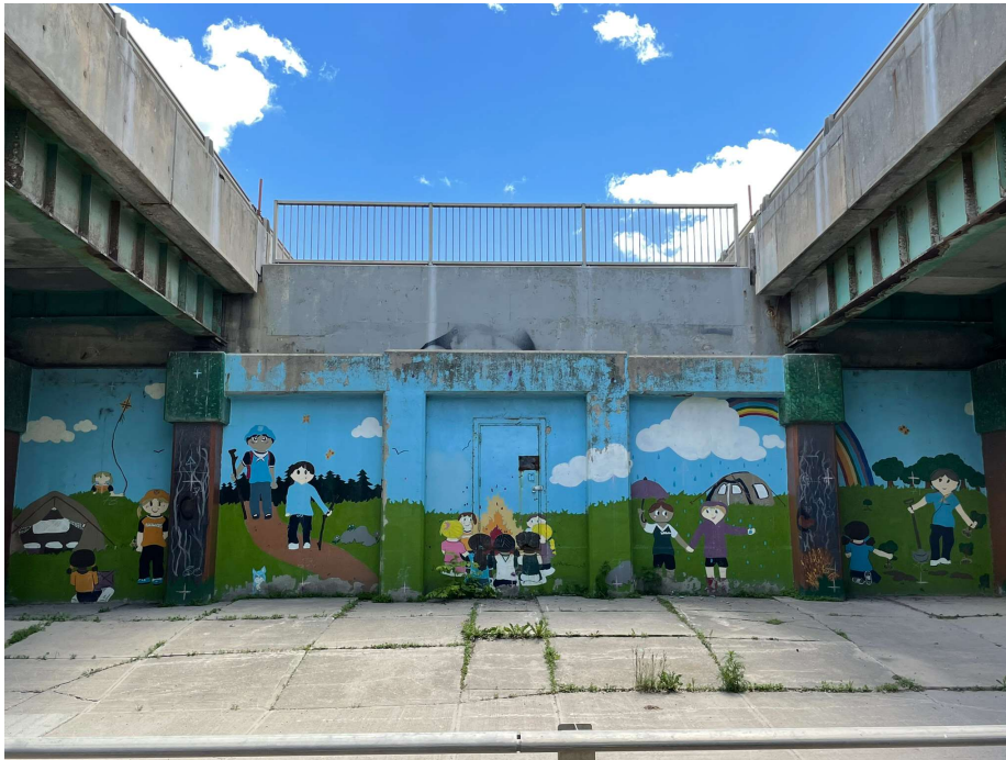
Photo 16 - South abutment wall, between NB and SB lanes
