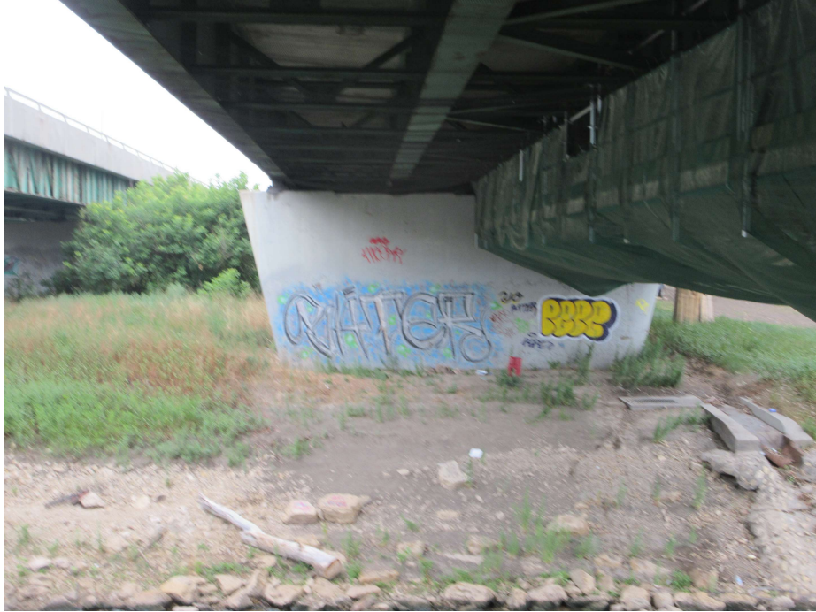
Photo 35 - Pier 3 NB South Face
