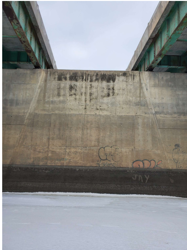
Photo 27 - Pier 6 South Face Middle Section
