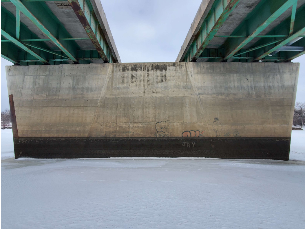
Photo 25 - Pier 6 South Face
