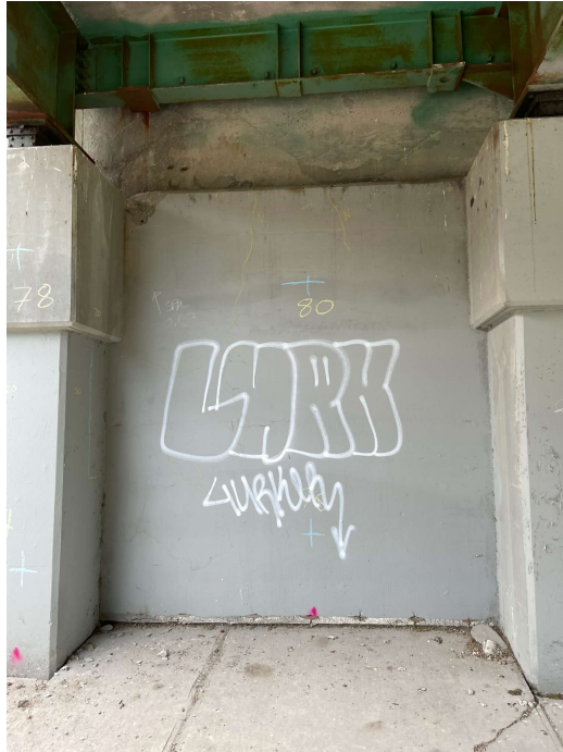
Photo 11 - North abutment, Column 7-8 (under NB lanes), narrow vertical cracking on abutment wall refacing and small localized spall near top of Column 7
