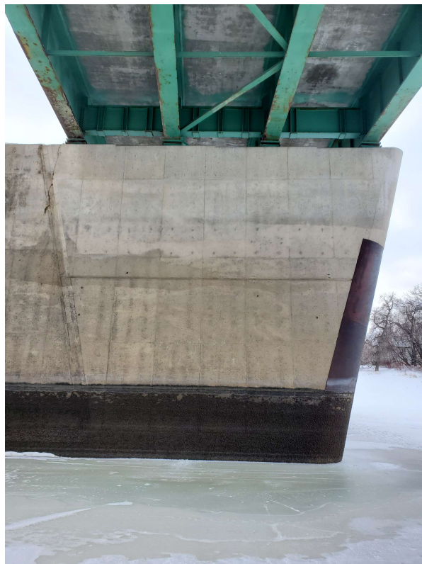
Photo 14 - Pier 5 North Face West Section 7 of 22
