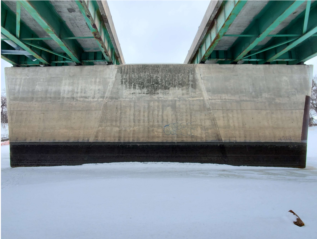
Photo 21 - Pier 6 North Face
