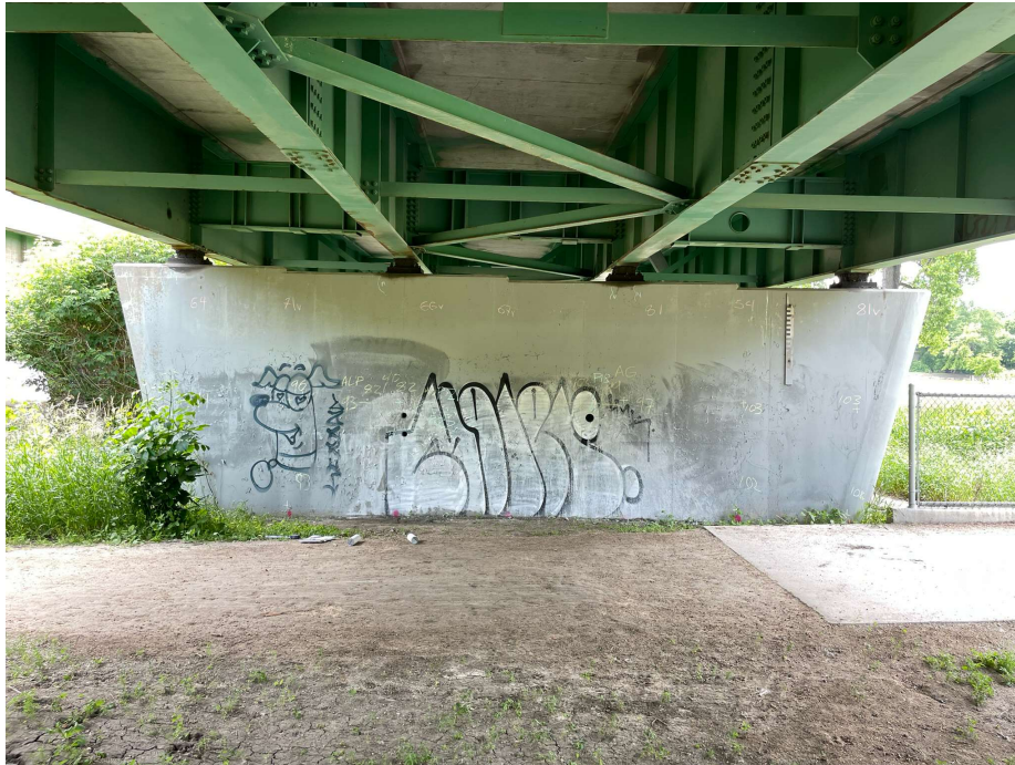
Photo 33 - Pier 2 SB, north face
