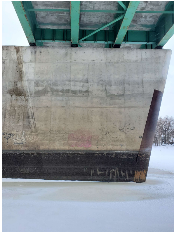
Photo 04 - Pier 4 North Face West Section 2 of 22
