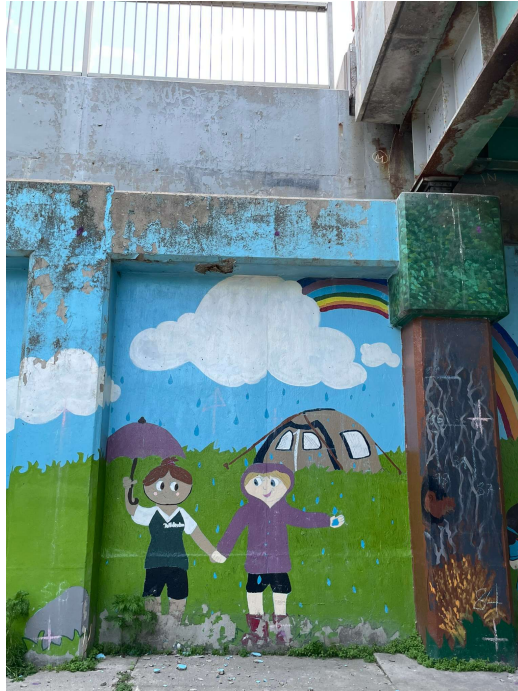
Photo 23 - South abutment wall, between NB and SB lanes, Column 6 – 7, localized spall on the underside of cap beam
