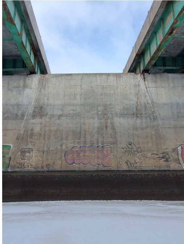
Photo 07 - Pier 4 South Face Middle Section
