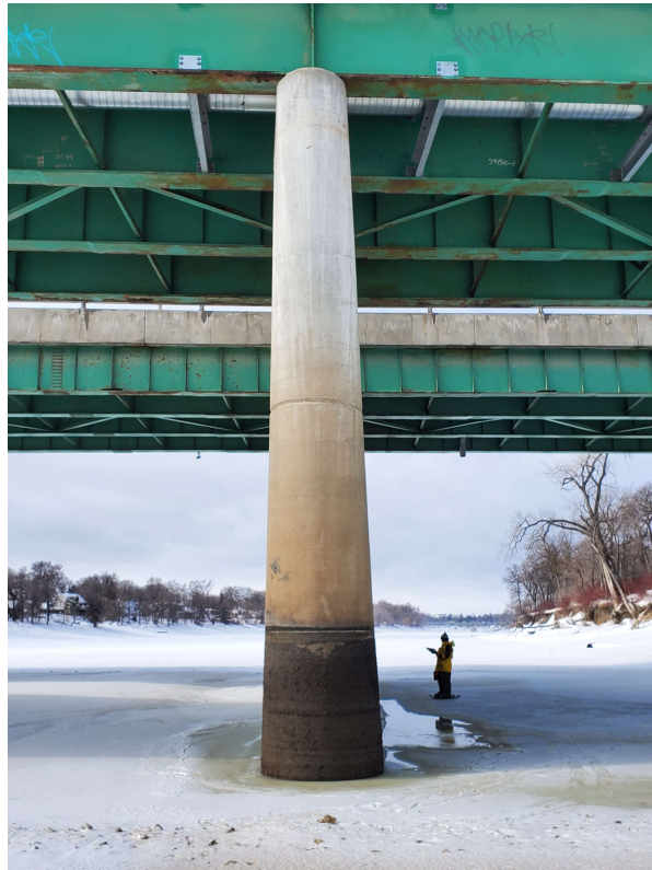
Photo 09 - Pier 4 East End
