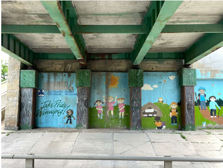
Photo 17 - South abutment wall, NB
