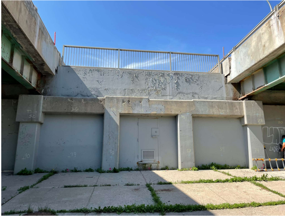
Photo 01 - North abutment wall, between NB and SB lanes
