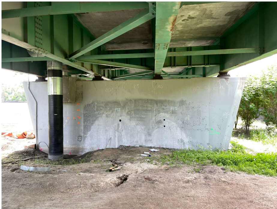
Photo 32 - Pier 2 NB, north face
