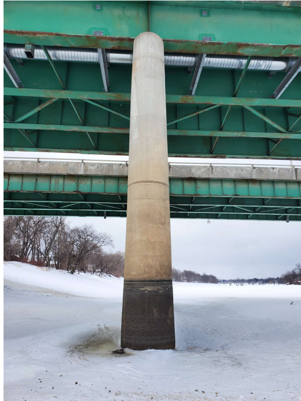
Photo 29 - Pier 6 East End
