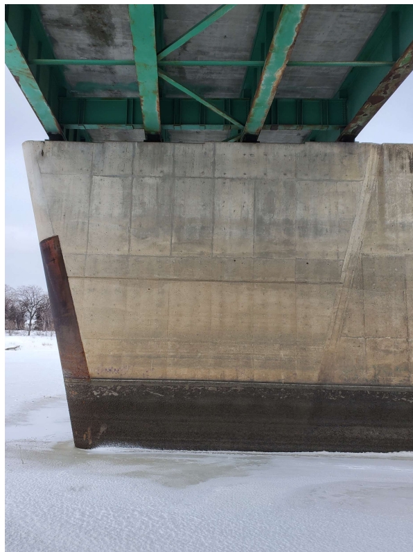
Photo 28 - Pier 6 South Face West Section 14 of 22
