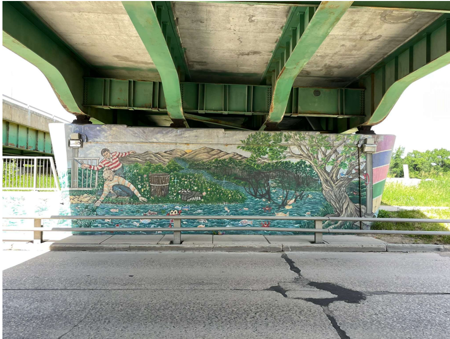
Photo 45 - Pier 8 NB, south face
