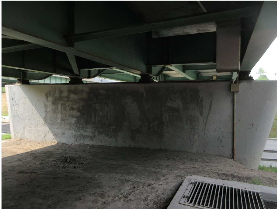
Photo 29 - Pier 1 NB South Face
