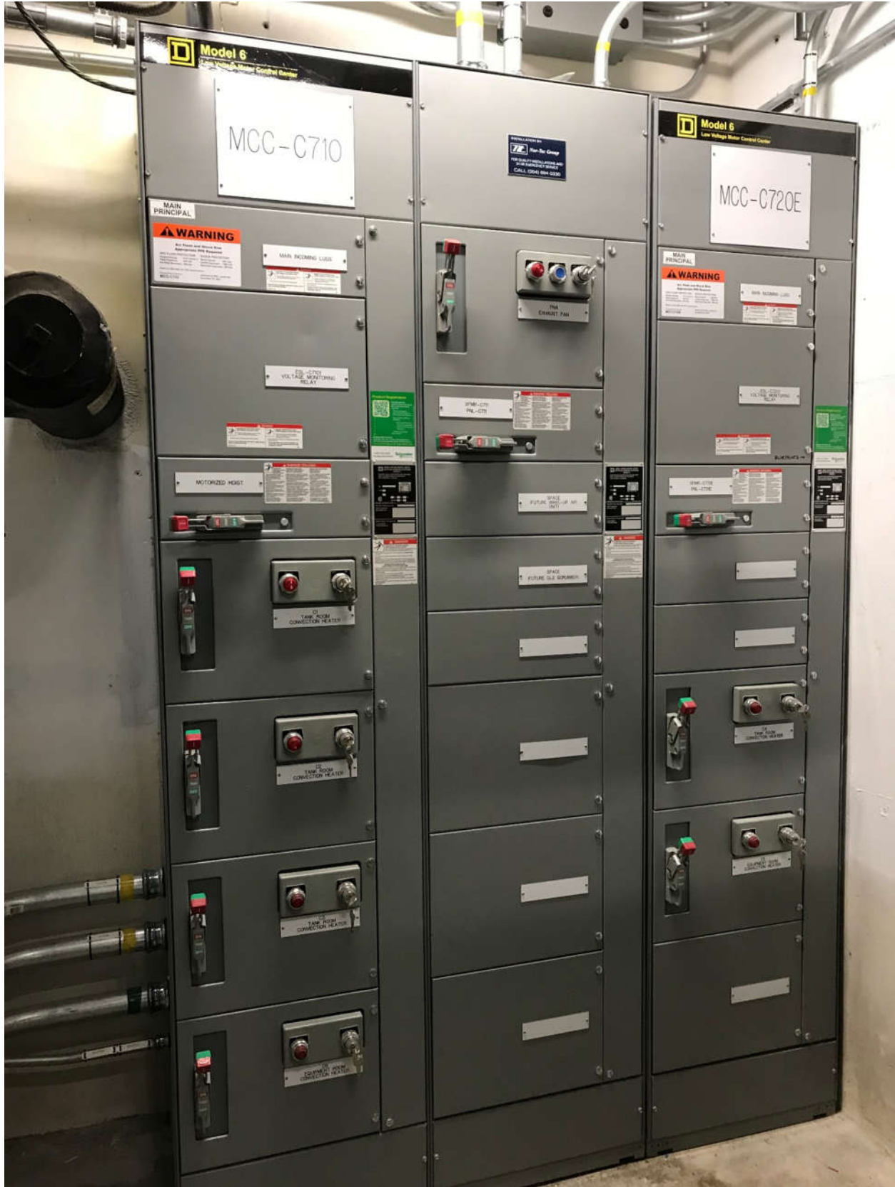
Photograph McP-1.7: McPhillips Chlorine Building 600V Motor Control Centres
