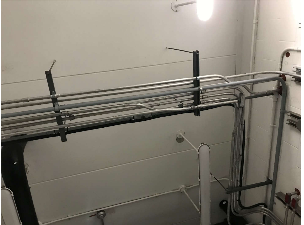
Photograph McP-1.6: McPhillips Chlorine Building Ceiling
