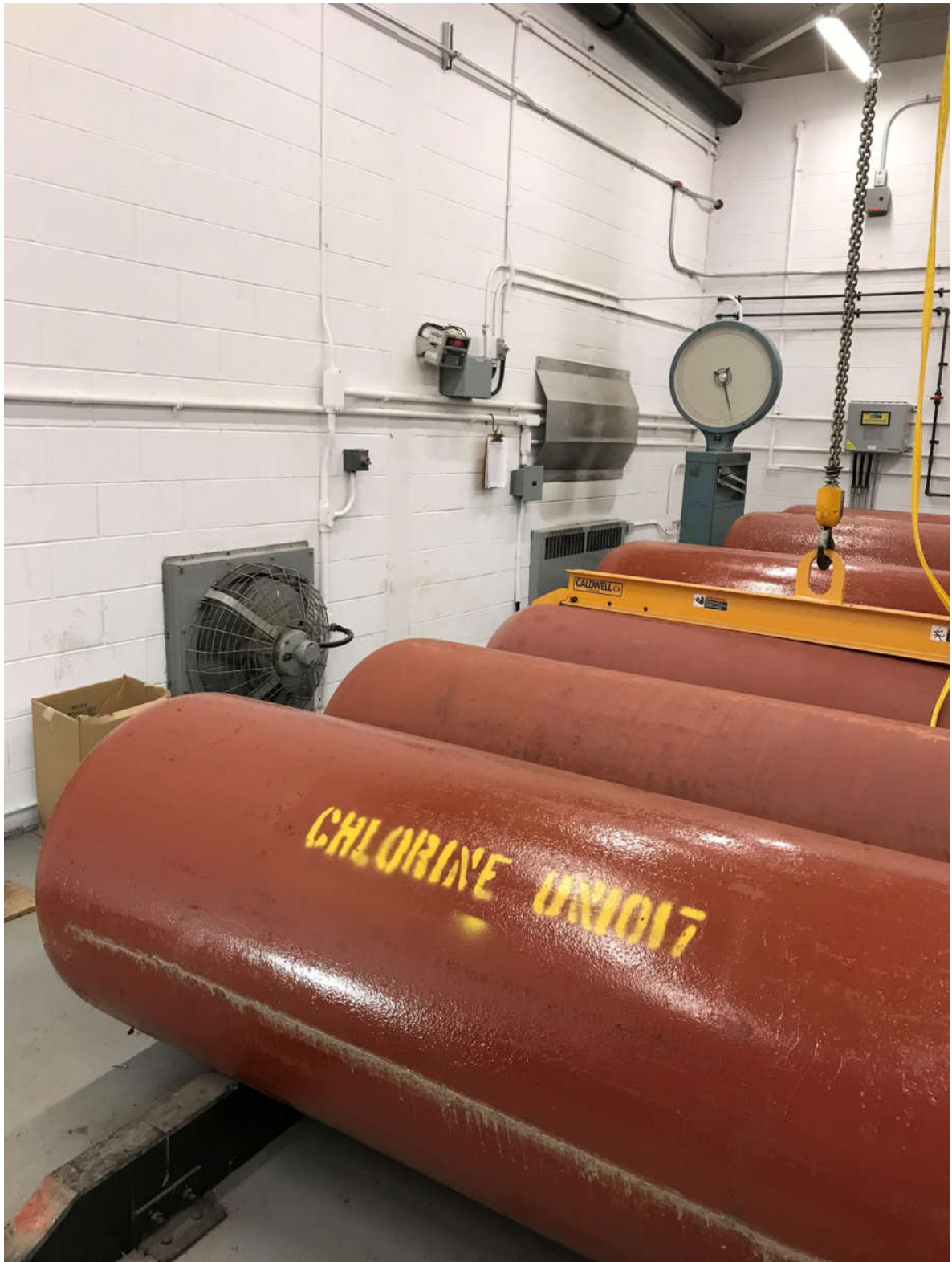
Photograph McP-1.2: McPhillips Tonner Room Looking North West
