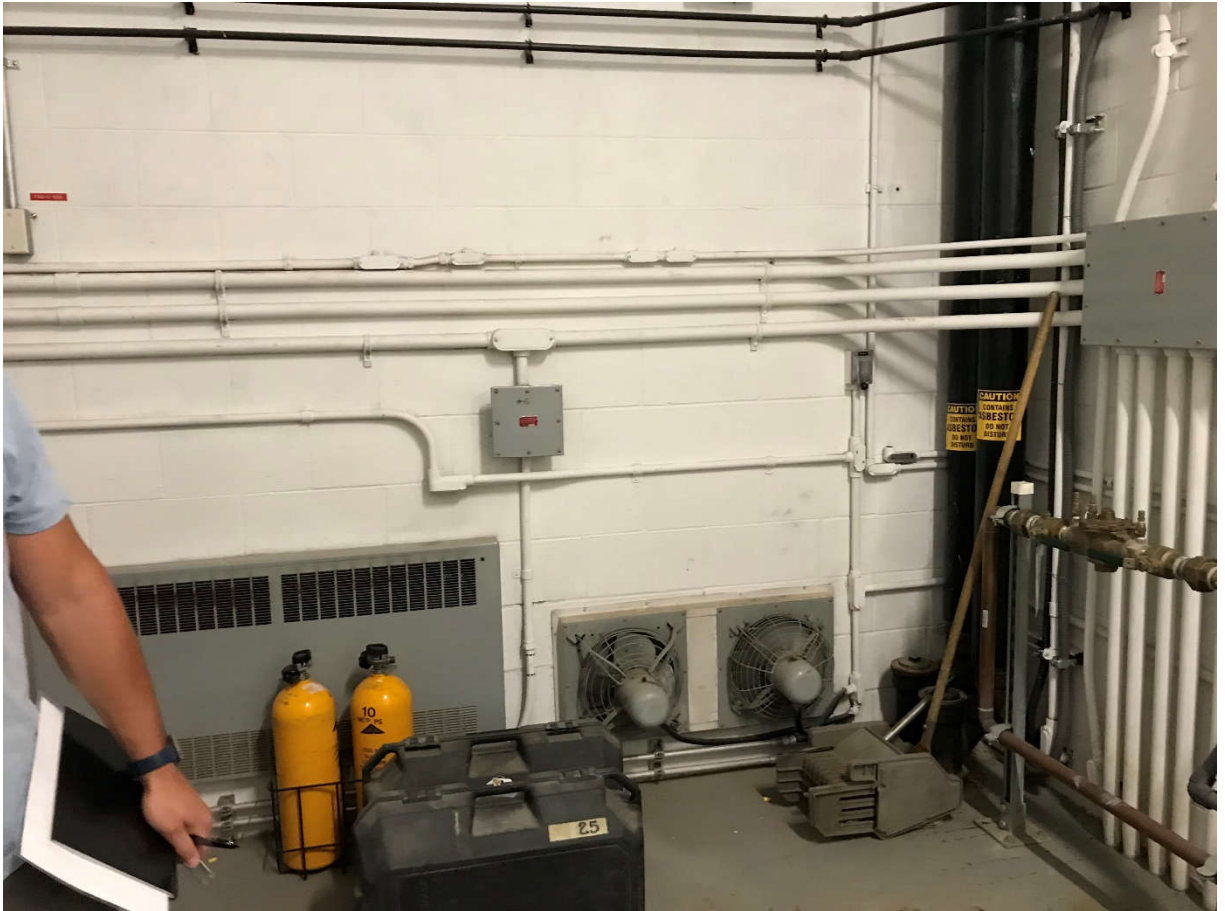
Photograph McP-1.5: McPhillips Chlorinator Room West Wall
