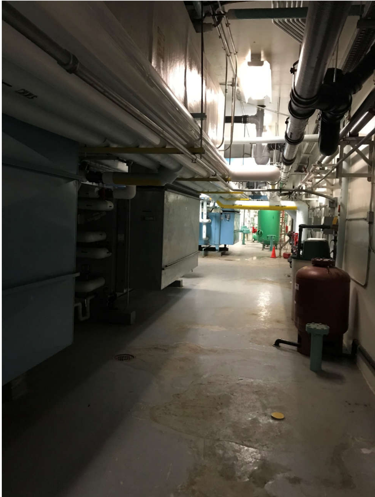
Photograph MacL-1.9: MacLean Mezzanine Level Below Tonner Room
