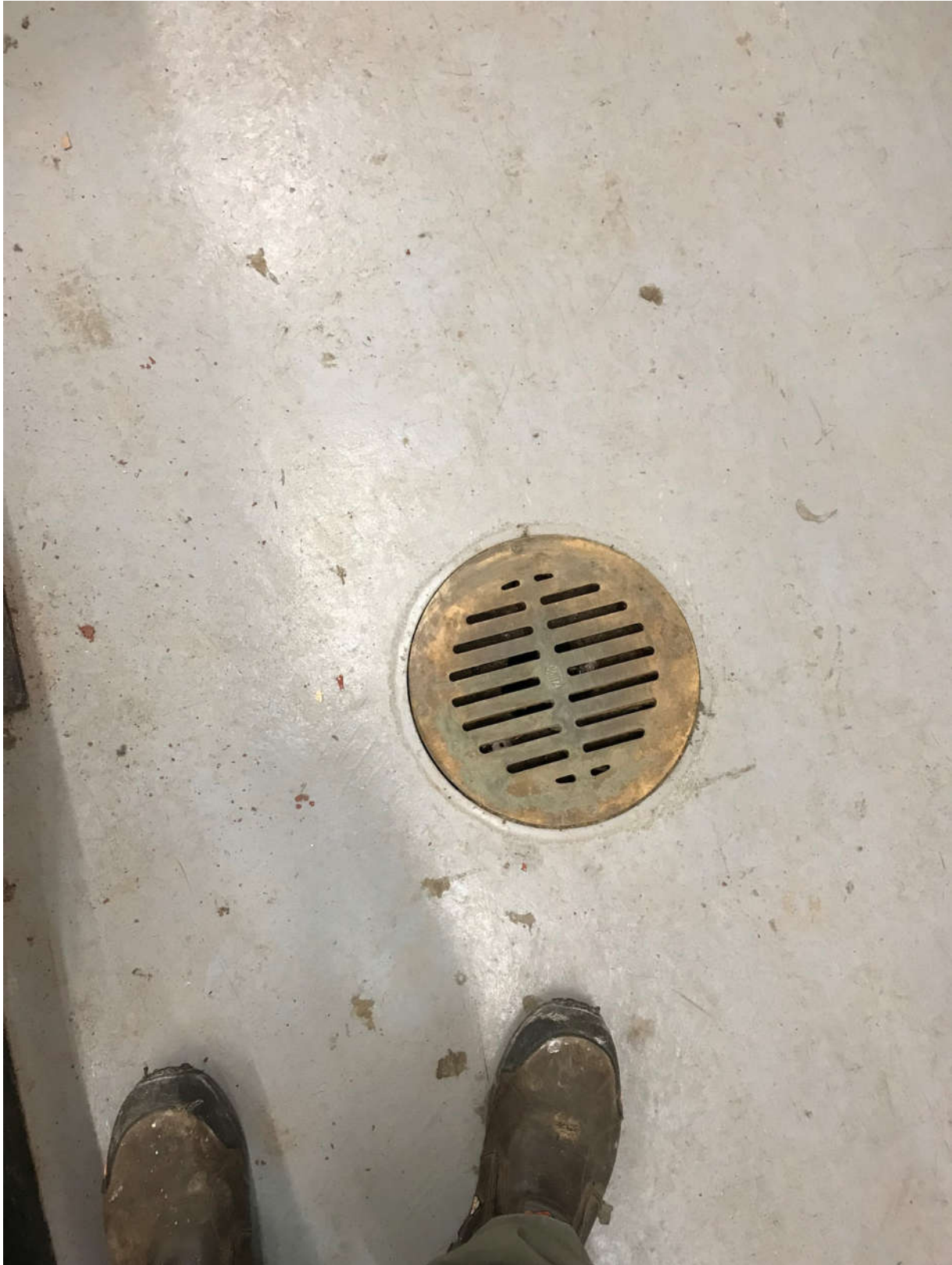
Photograph McP-1.3: McPhillips Tonner Room Typical Floor Drain
