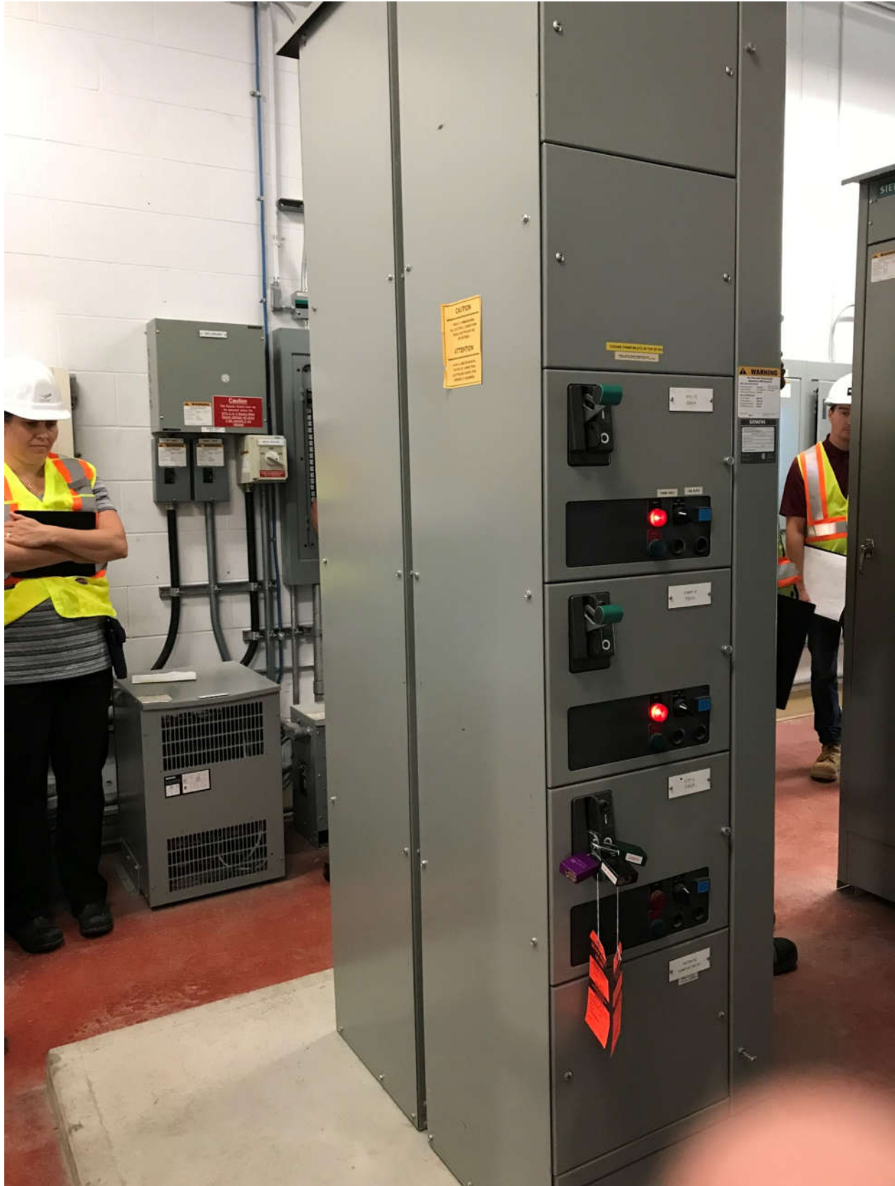
Photograph HUR-1.5: Hurst 600V Motor Control Centre
