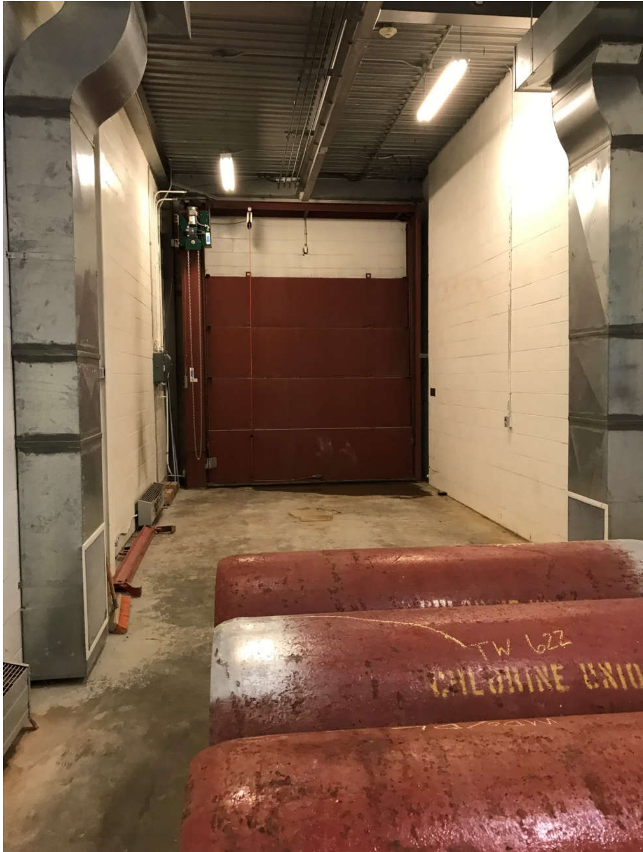
Photograph HUR-1.7: Hurst Tonner Room Looking West
