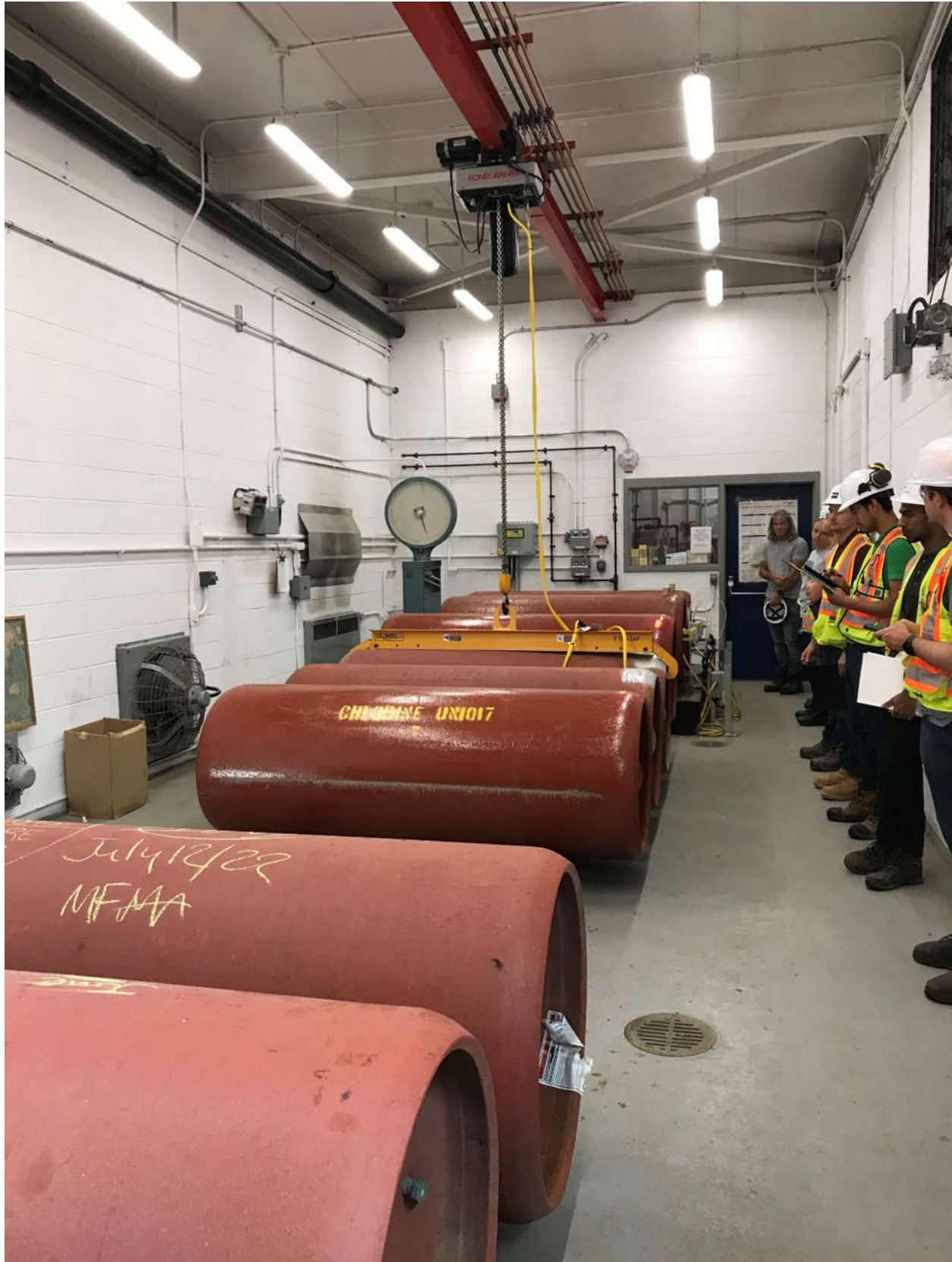
Photograph McP-1.1: McPhillips Tonner Room Looking North
