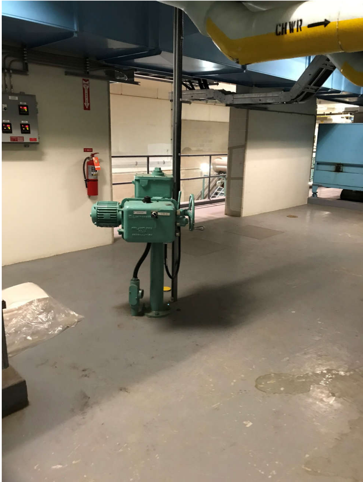
Photograph MacL-1.10: MacLean Mezzanine Level Below Tonner Room
