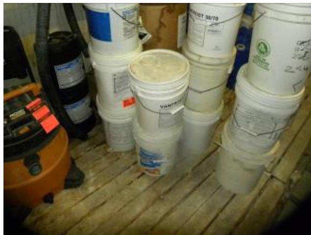
Photo #33 – View of chemical storage in the basement of the main Bonivital Pool building.
