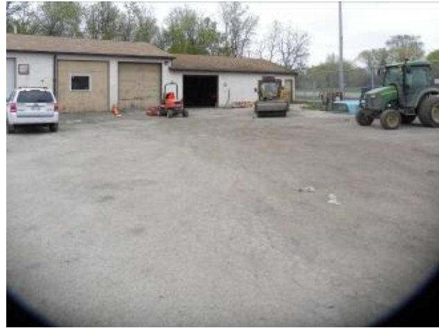
Photo #1 – View of eastern portion of the Public Works main building looking north.
