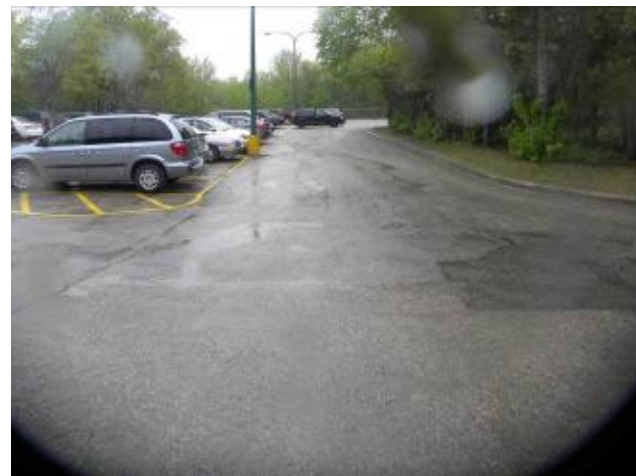
Photo #27 – View of west parking lot looking west at Bonivital Pool.
