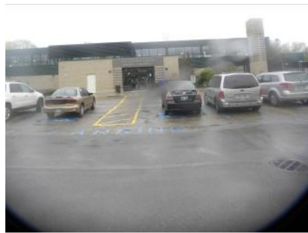
Photo #25 – View of Bonivital Pool building looking south.
