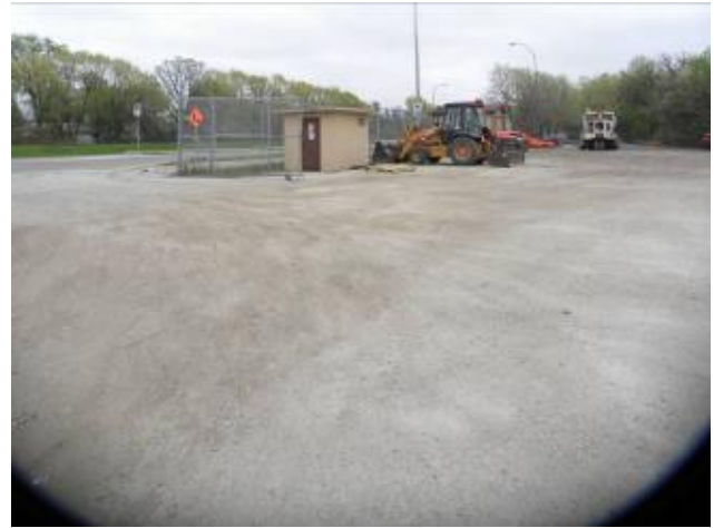
Photo #2 – View of eastern boundary of the Public Works Yard looking south.
