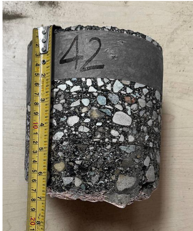
Turnbull Drive, NBL + , Core 42 (Asphalt Thk 170mm)
