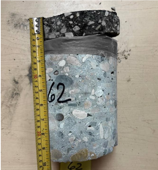
Scurfield Blvd, SBL ++ , Core 62 (Asphalt Thk 40mm, Concrete Thk 205mm)
