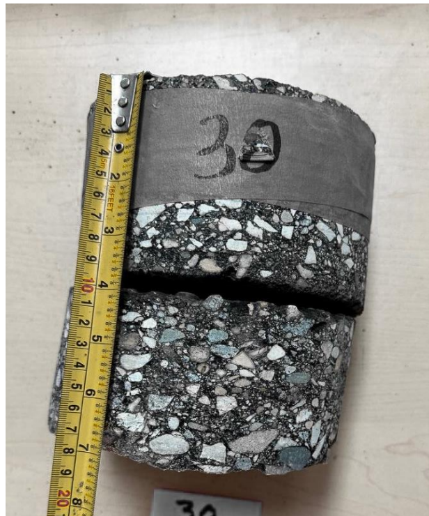
Turnbull Drive, SBL +++ , Core 30 (Asphalt Thk 170mm)
