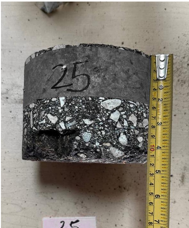
Turnbull Drive, NBL +++ , Core 25 (Asphalt Thk 140mm)
