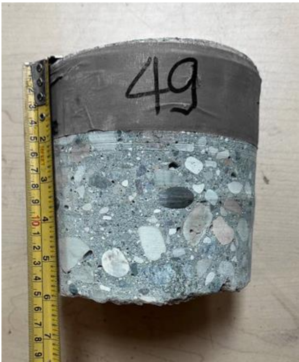
Westbourne Cr, NBL ++ , Core 49 (Concrete Thk 150mm)
