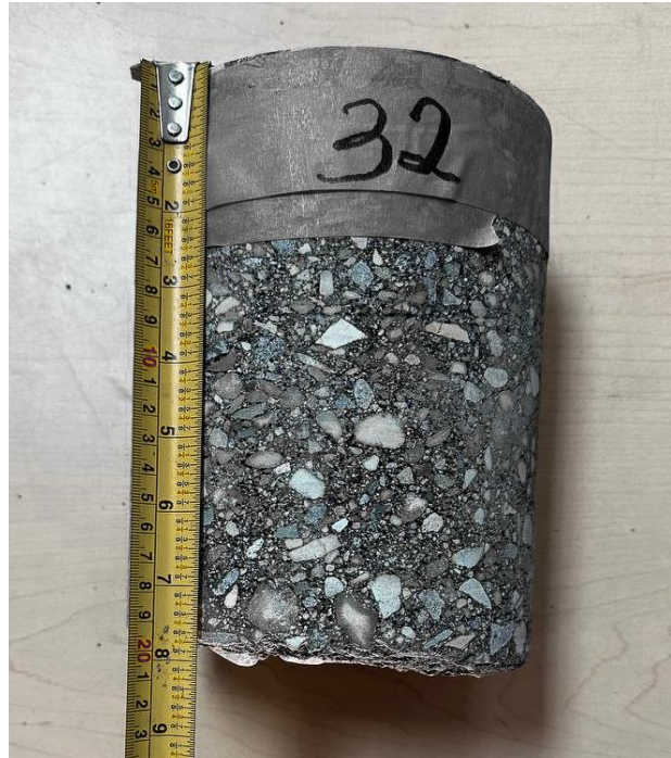
Turnbull Drive, SBL + , Core 32 (Asphalt Thk 195mm)
