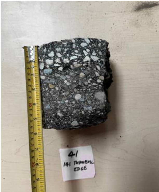
Turnbull Drive, SBL +++ , Core 41 (Asphalt Thk 145mm)
