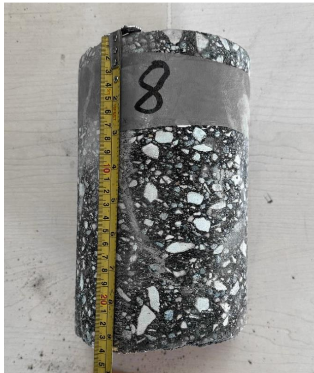
Brady Road, SBL + , Core 8 (Asphalt Thk 235mm)
