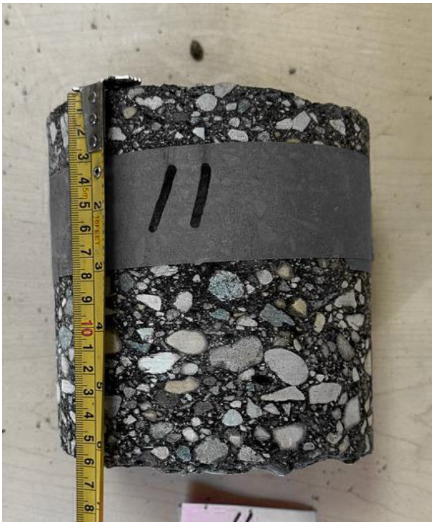
Brady Road, NBL + , Core 11 (Asphalt Thk 160mm)
