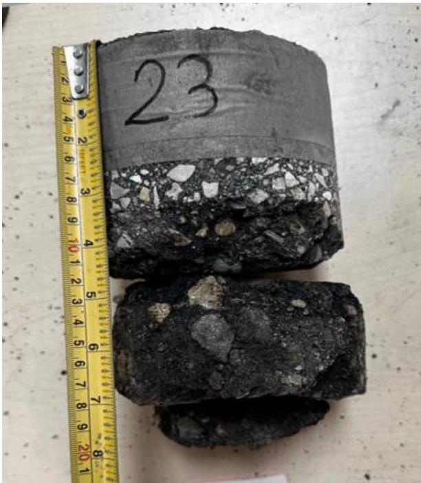
Turnbull Drive, SBL + , Core 23 (Asphalt Thk 210mm)
