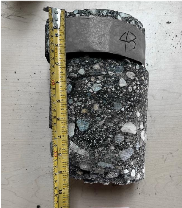
Turnbull Drive, SBL + , Core 43 (Asphalt Thk 240mm)
