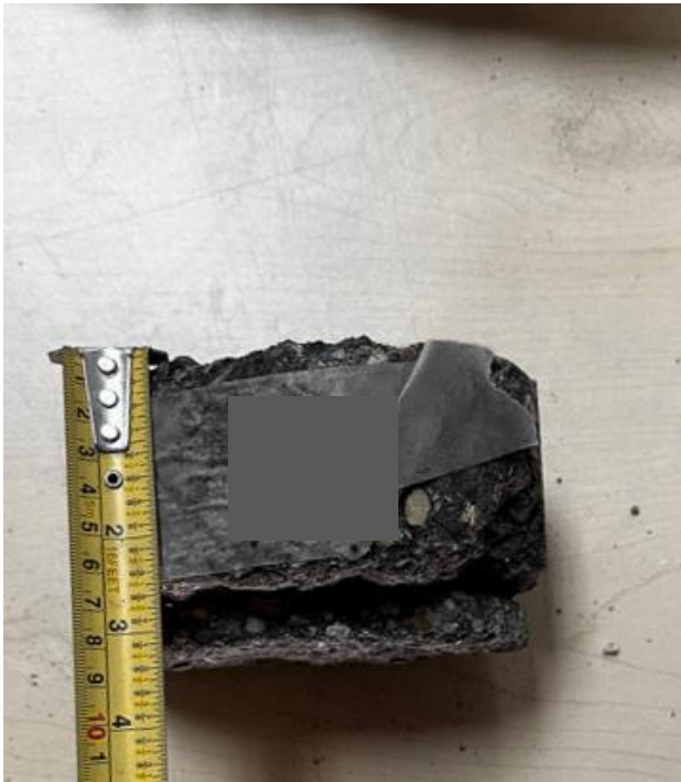
Providence PI, SBL ++ , Core 73 (Asphalt Thk 80mm)
