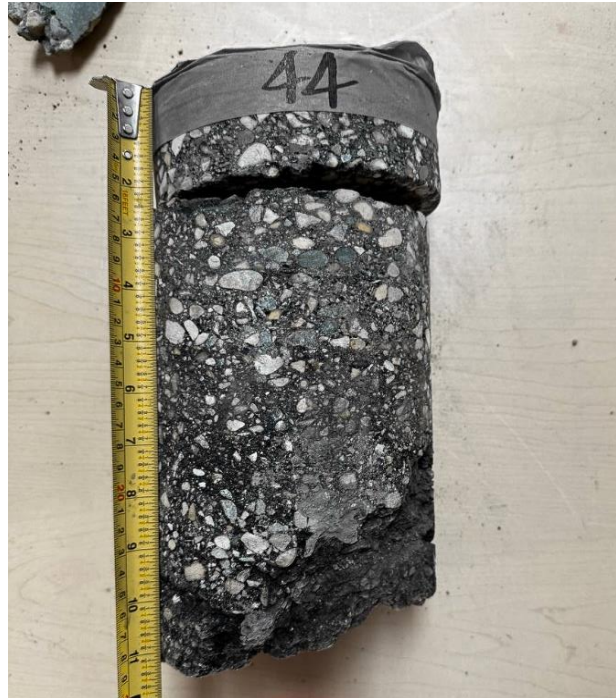
Turnbull Drive, SBL +++ , Core 44 (Asphalt Thk 275mm)
