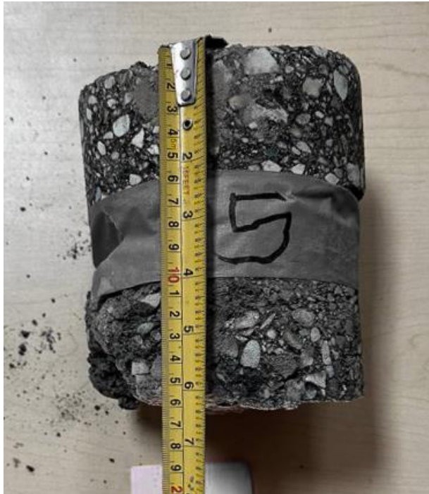
Brady Road, NBL + , Core 5 (Asphalt Thk 150mm)
