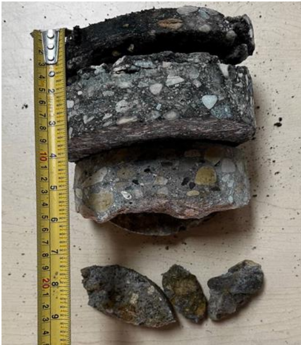
Fleetwood Rd, WBL ++ , Core 51 (Asphalt Thk 80mm, Concrete Thk 100mm)
