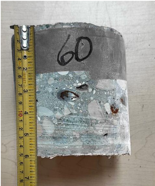
Scurfield Blvd, SBL ++ , Core 60 (Concrete Thk 145mm)
