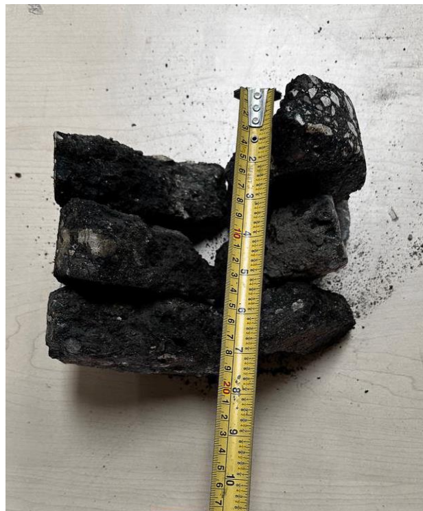
Turnbull Drive, NBL + , Core 38 (Asphalt Thk 160mm)
