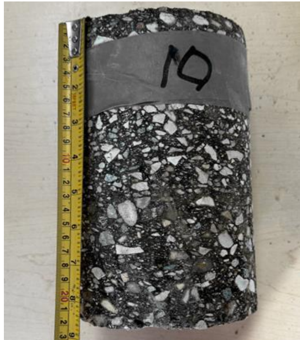
Brady Road, SBL + , Core 10 (Asphalt Thk 220mm)
