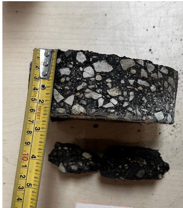
Turnbull Drive, NBL + , Core 28 (Asphalt Thk 100mm)
