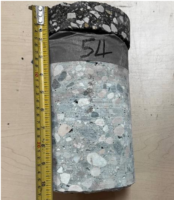
Scurfield Blvd, NBL ++ , Core 54 (Asphalt Thk 40mm, Concrete Thk 215mm)
