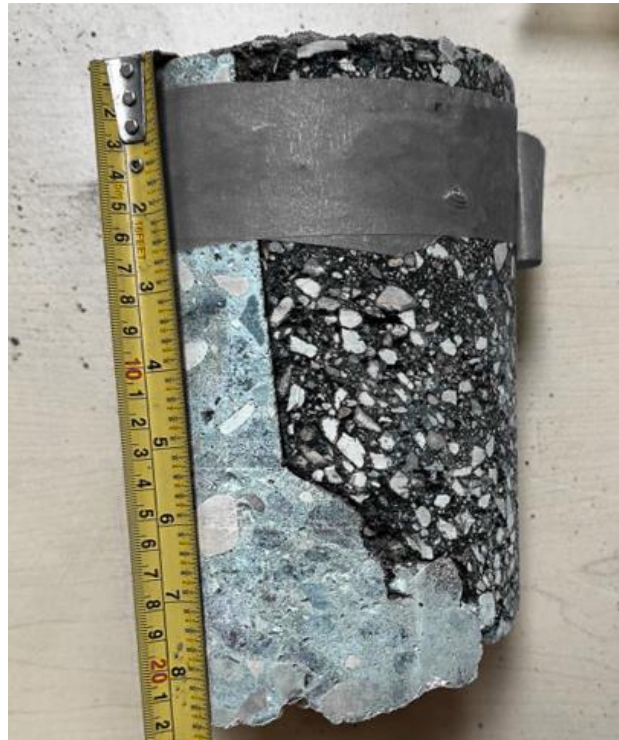
Augusta Dr, EBL ++ , Core 69 (Asphalt Thk 210mm, Concrete 210mm)
