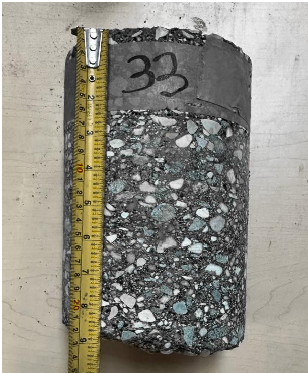
Turnbull Drive, NBL + , Core 33 (Asphalt Thk 230mm)
