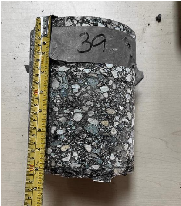
Turnbull Drive, NBL +++ , Core 39 (Asphalt Thk 205mm)
