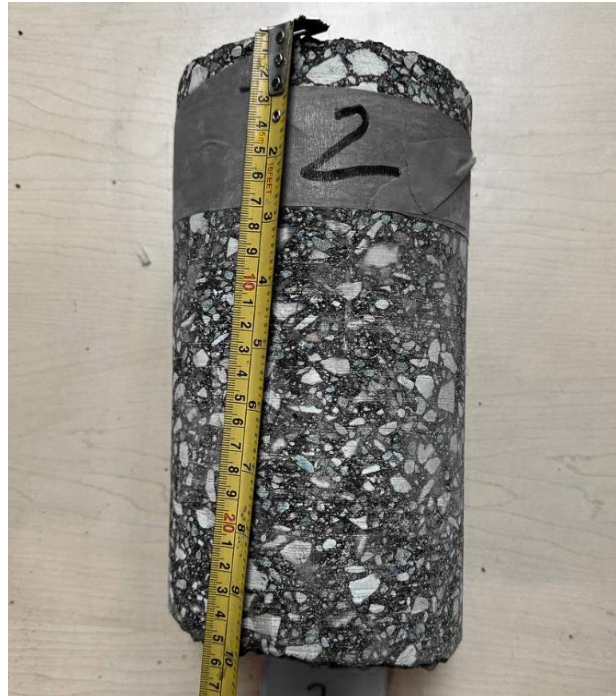
Brady Road, SBL + , Core 2 (Asphalt Thk 252mm)
