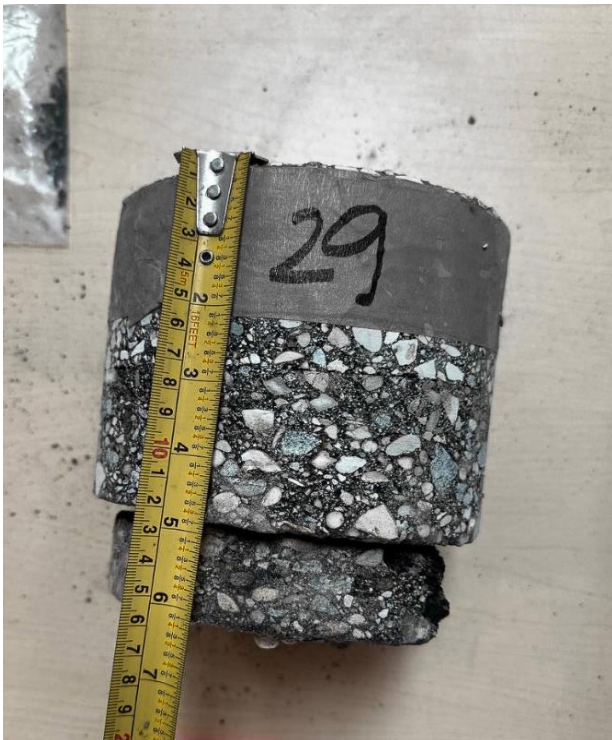
Turnbull Drive, SBL + , Core 29 (Asphalt Thk 155mm)
