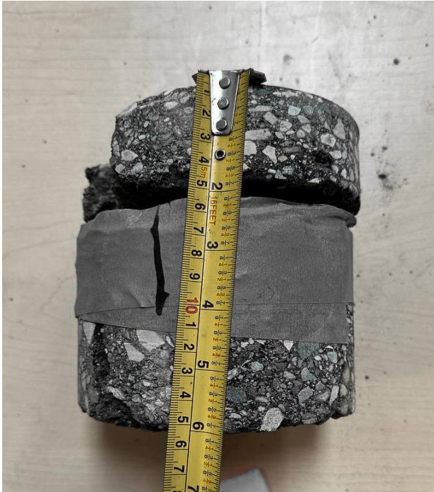
Brady Road, NBL + , Core 1 (Asphalt Thk 140mm)
