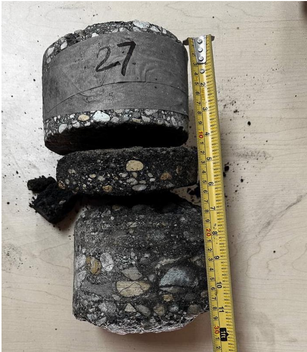
Turnbull Drive, SBL +++ , Core 27 (Asphalt Thk 270mm)
