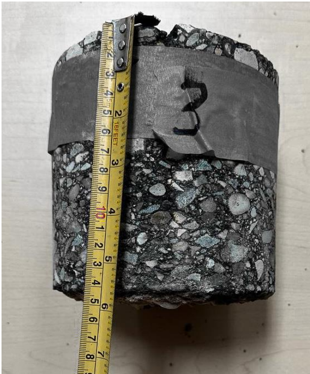
Brady Road, NBL + , Core 3 (Asphalt Thk 140mm)
