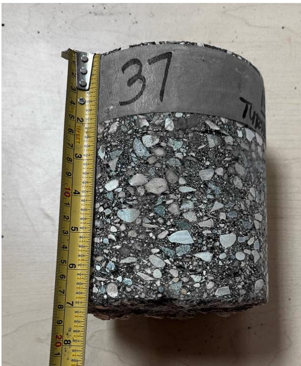
Turnbull Drive, SBL + , Core 37 (Asphalt Thk 245mm)
