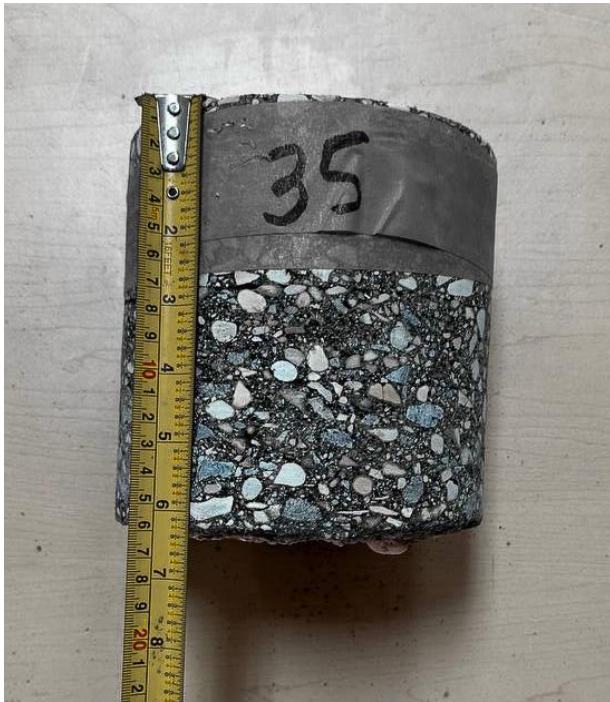
Turnbull Drive, SBL + , Core 35 (Asphalt Thk 160mm)
