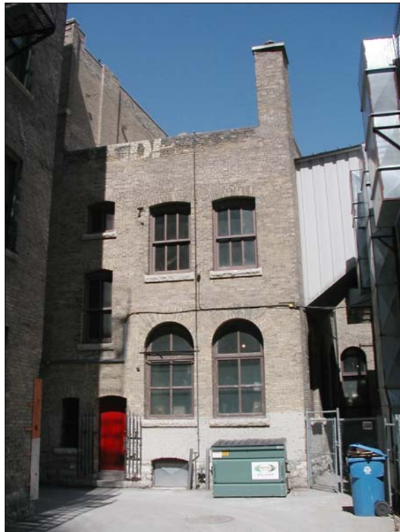
Plate 21 – Rear (south) façade. ( M. Peterson, 2003. )
