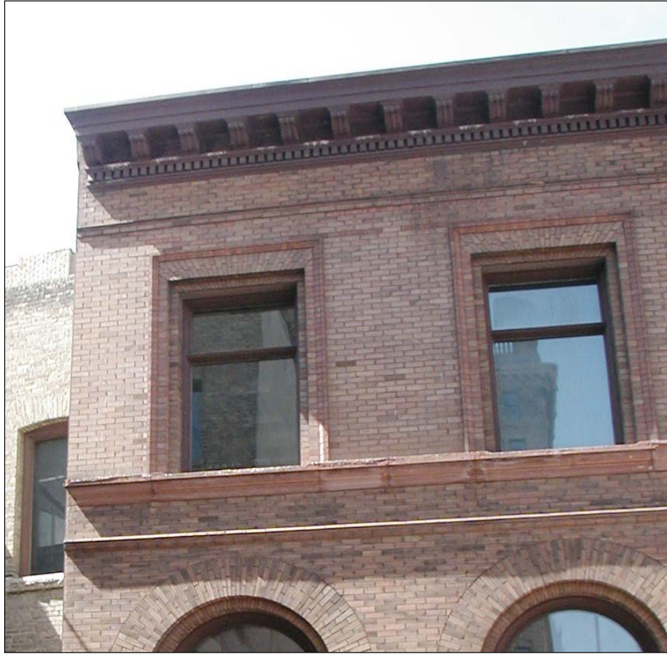
Plate 16 – Second-storey window detail. ( M. Peterson, 2003. )
