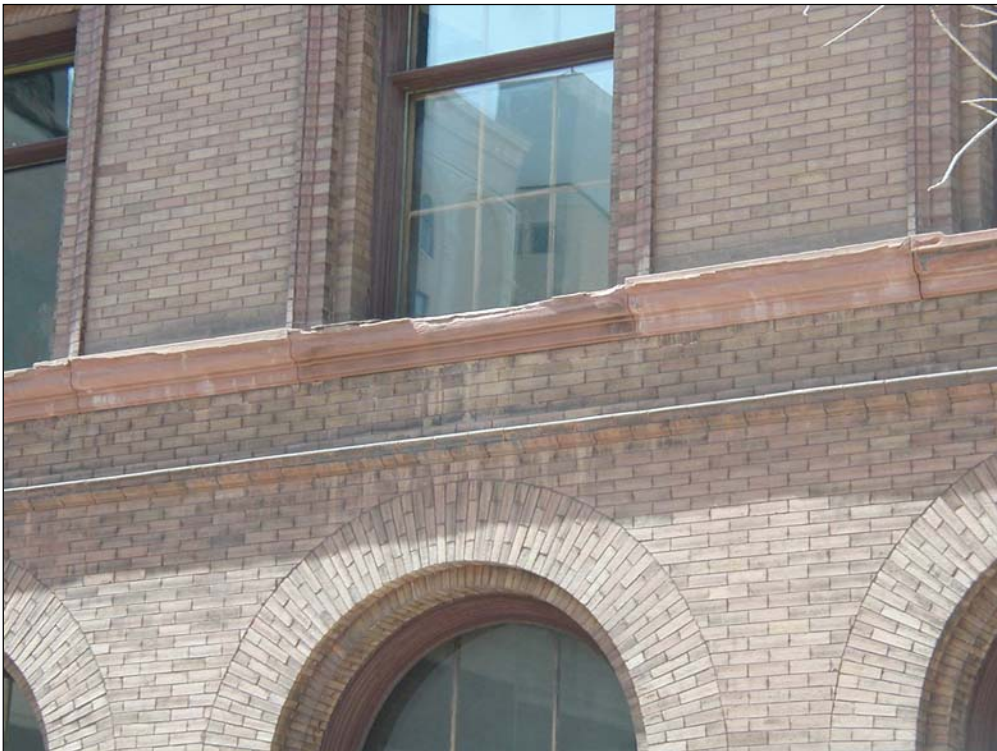
Plate 15 – Brick belt course and sandstone band that forms a continuous sill for second-floor. ( M. Peterson, 2003. )
