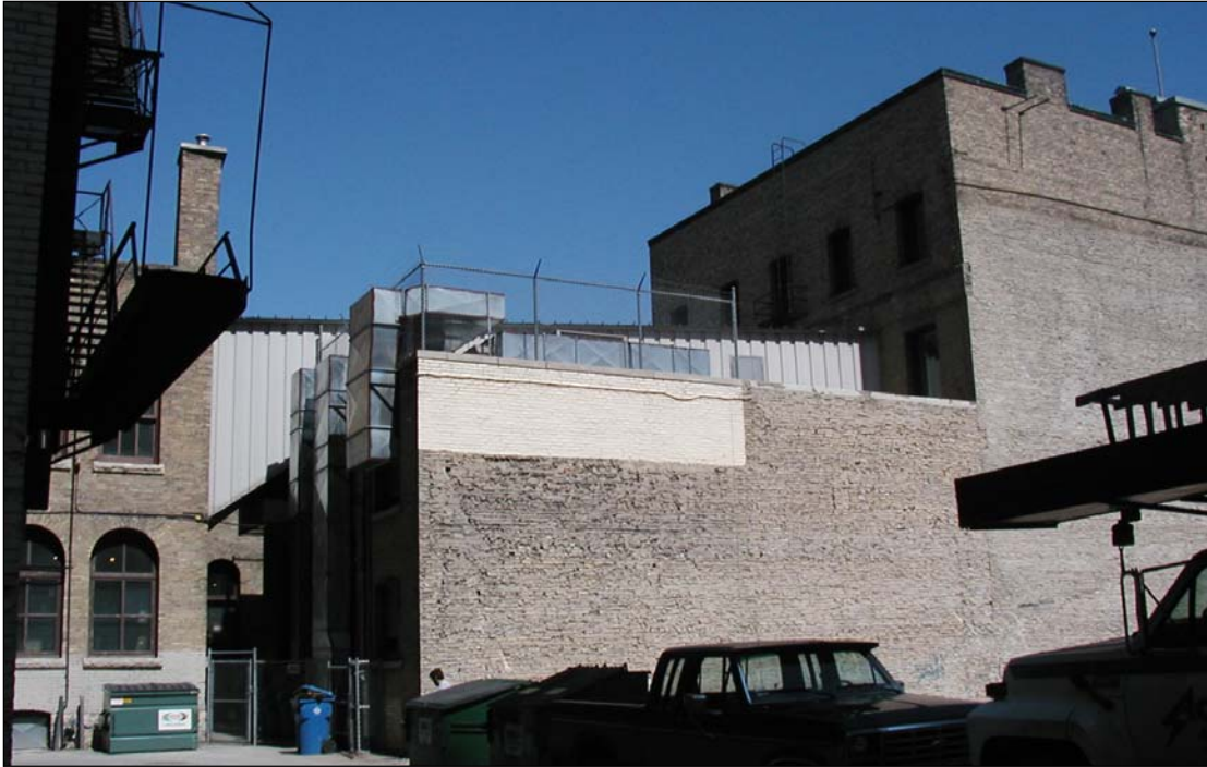
Plate 26 – Overhead walkway between the Lake of the Woods Building and Newmac Building. ( M. Peterson, 2003. )
