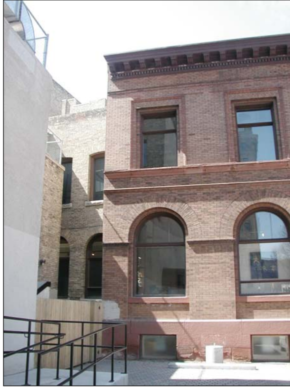
Plate 20 – Rear of east side. ( M. Peterson, 2003. )
