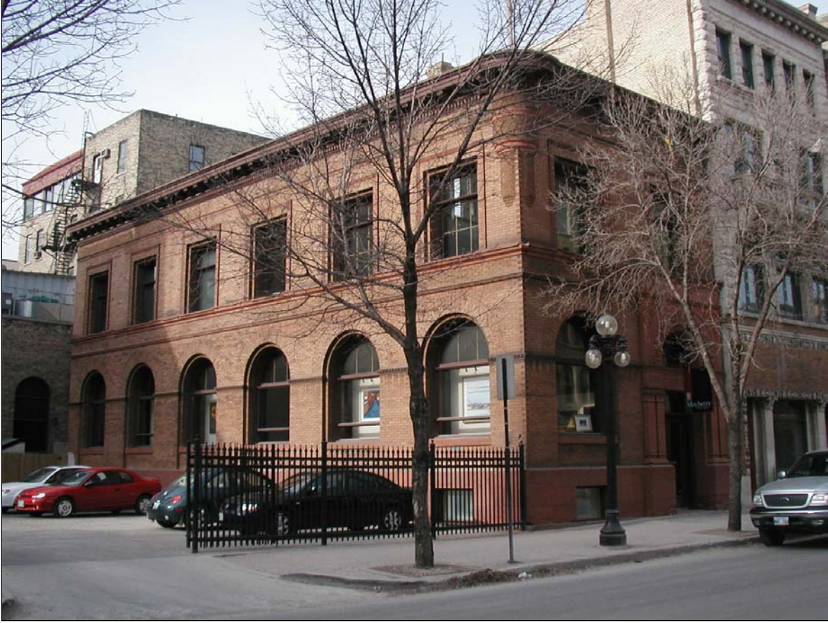
Plate 1 – Lake of the Woods Building, 212 McDermot Avenue, front (north) and east façades. ( M. Peterson, 2003. )
