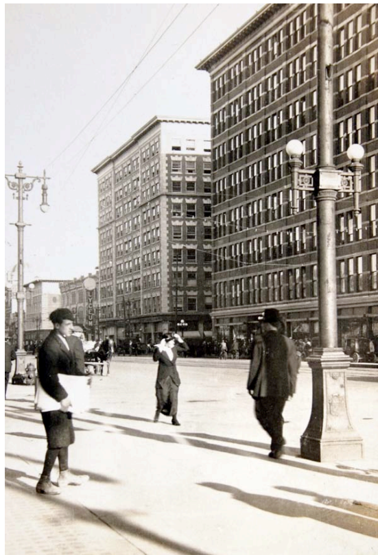
Portage Avenue retail section, no date
