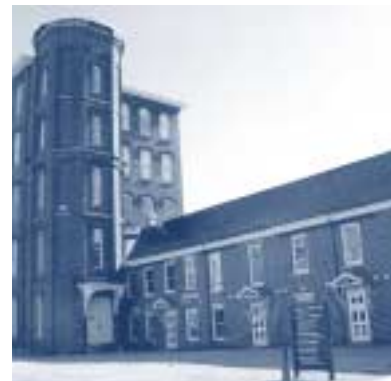
Interpretive Centre in a converted mill at the Boot Cotton Mill, Lowell, MA.
