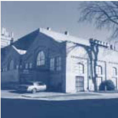
James Avenue Pumping Station, Winnipeg.
