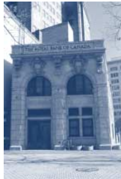
The west face of the Royal Bank Annex, Exchange District National Historic Site.
