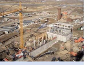
Winnipeg's new \$300 million (estimated) **Water Treatment Plant** is currently under construction at the Deacon Reservoir. The plant will be approximately 12,000 square metres about the size of the downtown MTS Centre. The concrete pour alone was 1,100 cubic metres, the largest by PCL Construction in Manitoba. When completed by the end of 2008, the plant will be able to treat 400 million litres of water a day.
